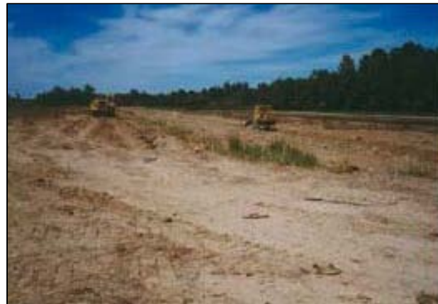
Figure 7-4: Wetland Mitigation Site During Construction
