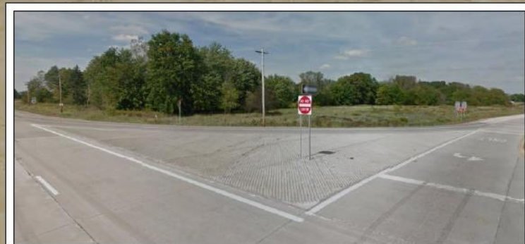
Raised Corrugated Island at US 31-US 6 Interchange NW Corner
