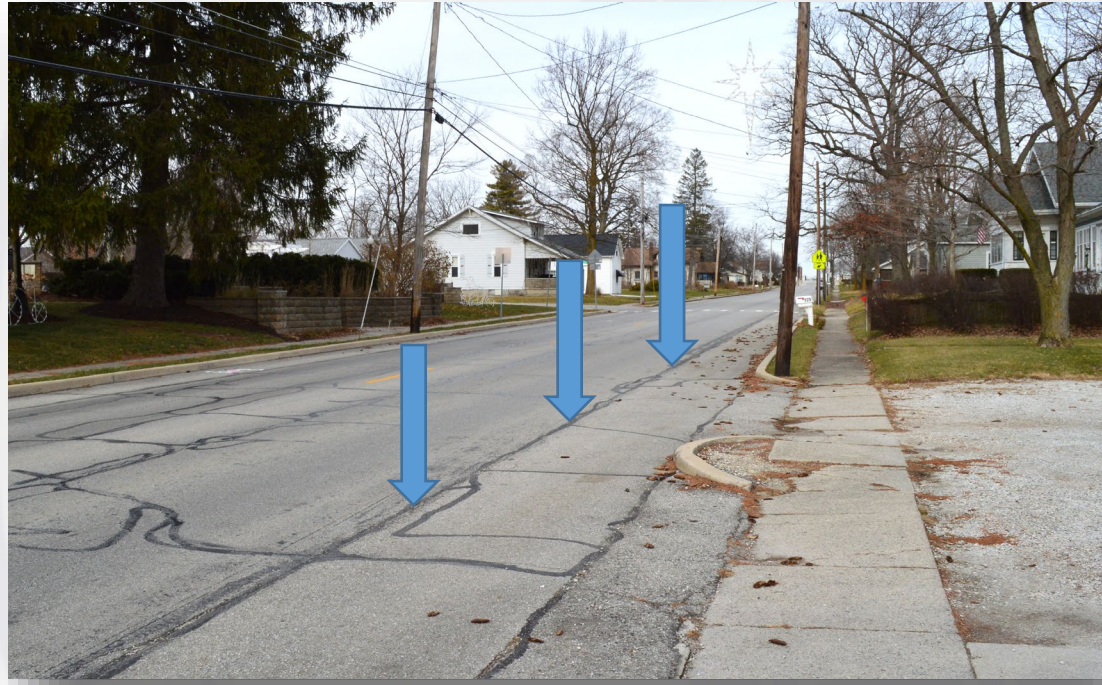
Looking north along SR 22 (Main Street)
