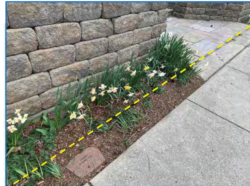
Photo 4 – View of area of proposed 1-foot wide strip of temporary right-of-way along entrance to Memorial Park facing down. The sidewalk will be replaced in the same location. Any features, if disturbed, will be restored including pavers and landscaping. (04-22-20)
