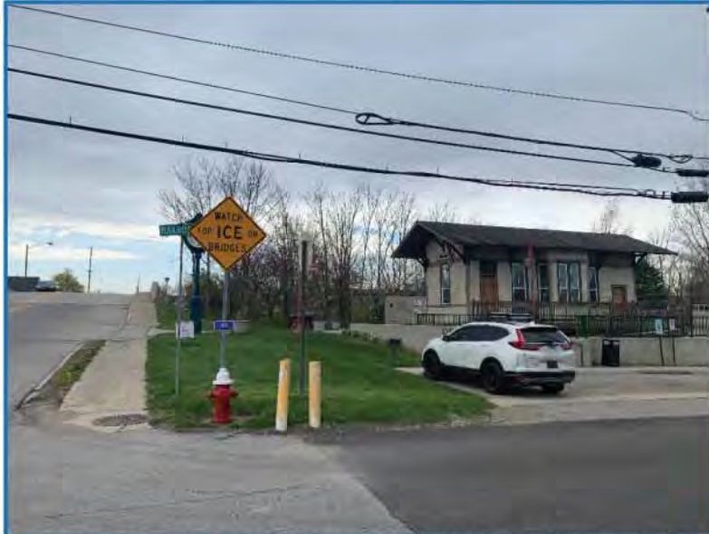
Photo 1 – View of Depot Park facing south from the intersection of SR 22 and Railroad Street. The SR 22 bridge over CERA railroad is on the left.(04-22-20)
