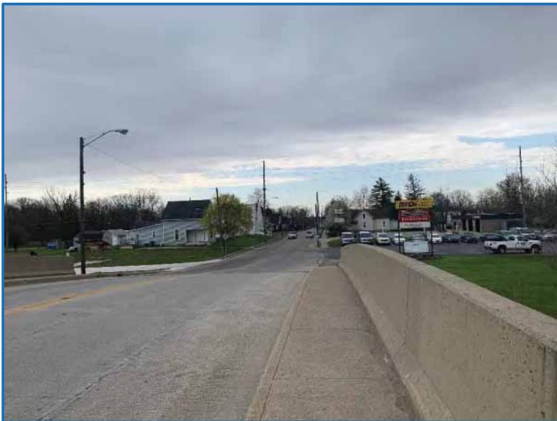
Photo 3 – View of SR 22 facing south from the west side of the SR 22 bridge over CERA railroad. The trailhead entrance is on the left. (04-22-20)
