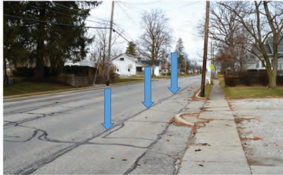
Looking north along SR 22 (Main Street)
