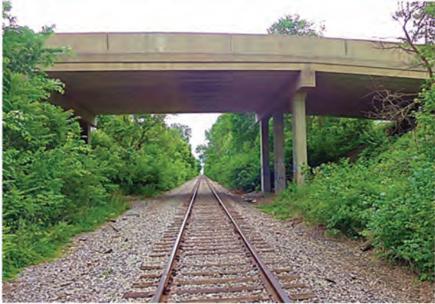
Looking east at the Main Street bridge
