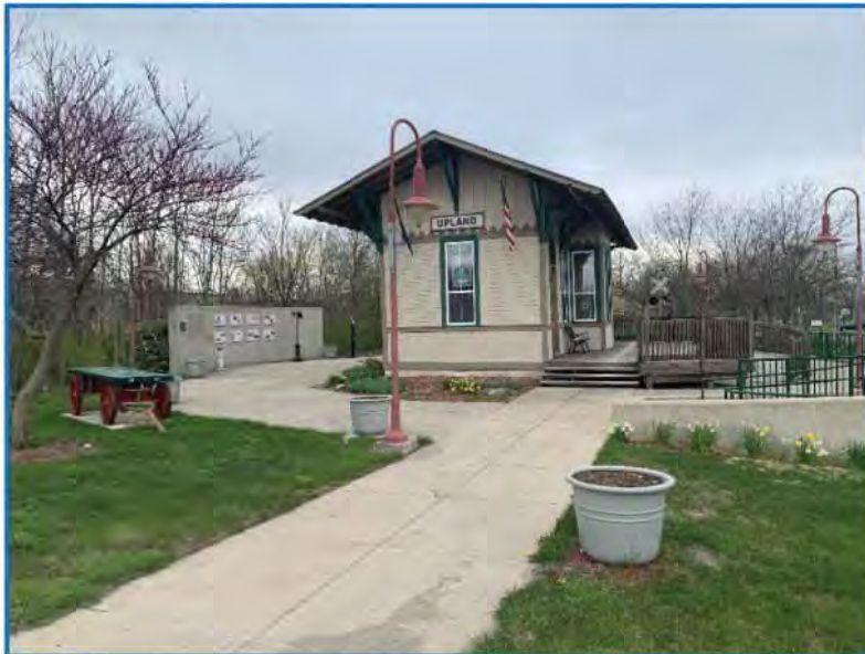
Photo 3 – View of existing walkway, light, and depot building facing west from SR 22. (04-22-20)
