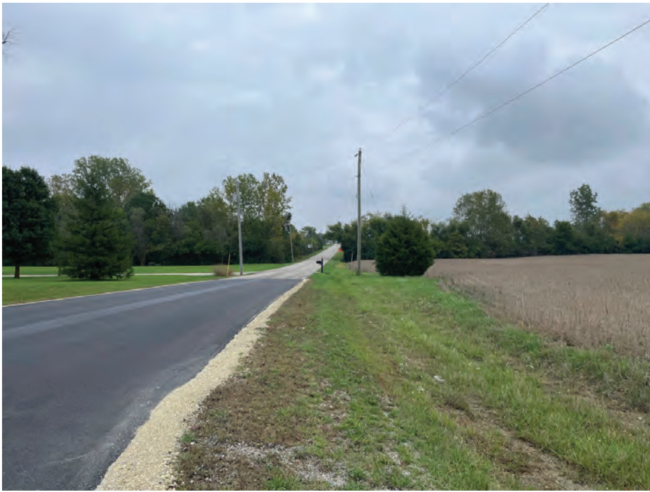
1. Looking E from the intersection of SR 1 and CR 800 W (10/4/2021)
