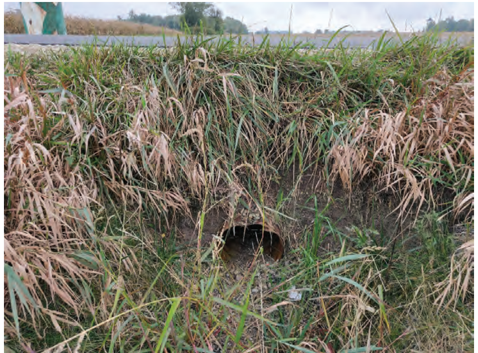
12. Looking S a drainage structure outlet that forms RSD 1 (10/4/2021)
