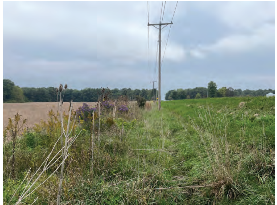
32. Looking N along UNT 1 to McClain Ditch from the small structure (10/6/2021)
