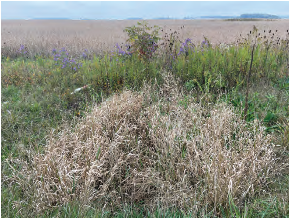
31. Looking E across the small structure inlet on the E side of SR 1 (10/6/2021)
