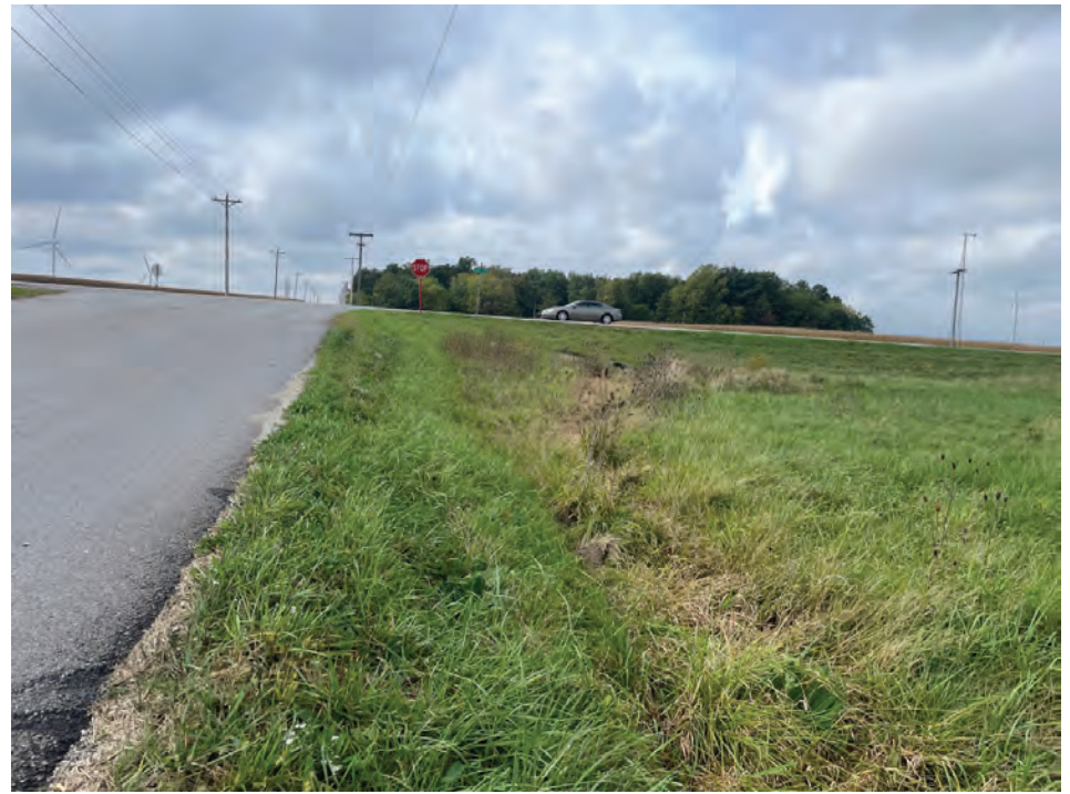
66. Looking W along the north side of CR 800 W towards wetland (10/15/2021)
