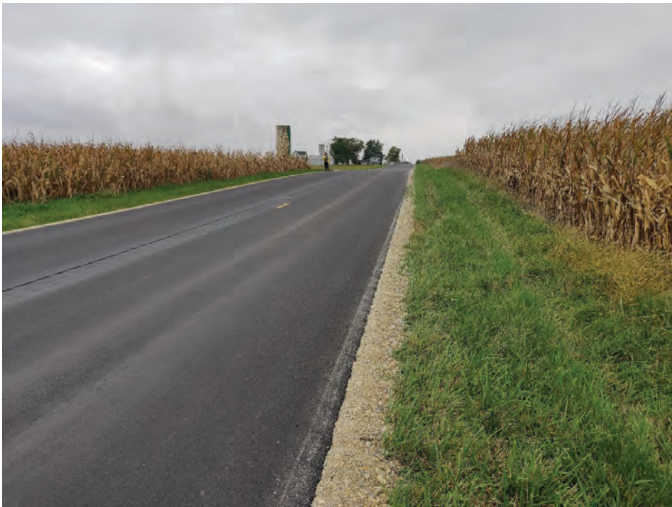
9. Looking W along the N side of SR 1 (10/4/2021)
