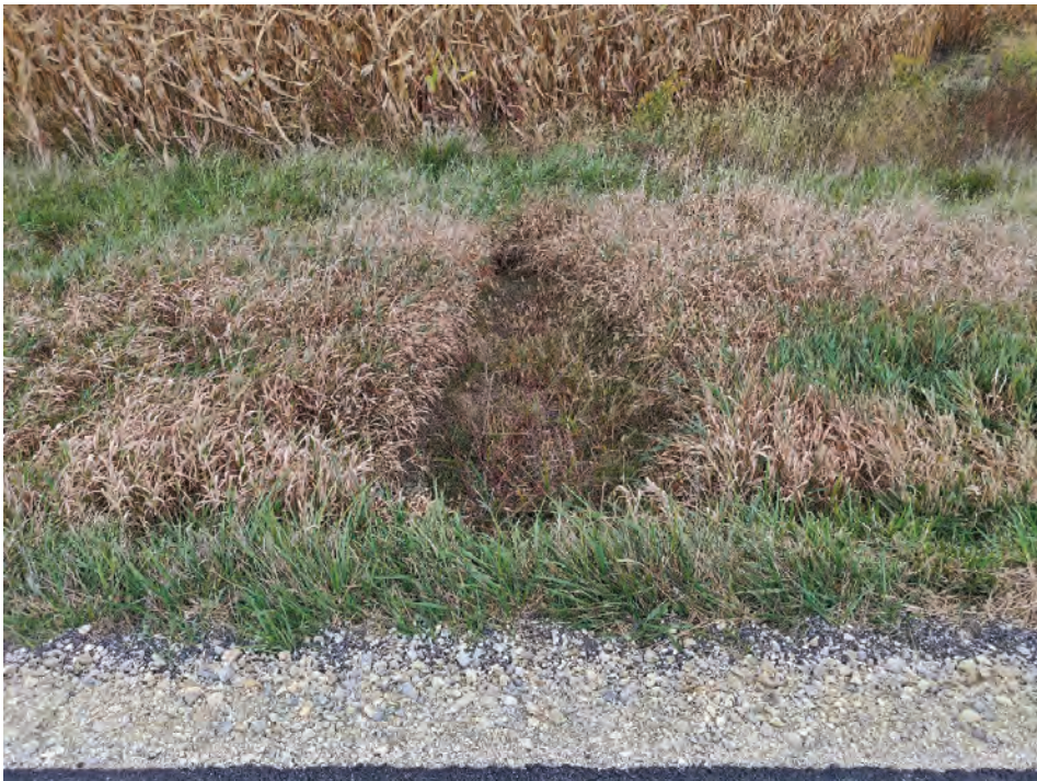
11. Looking N at the drainage structure outlet that forms RSD 1 (10/4/2021)
