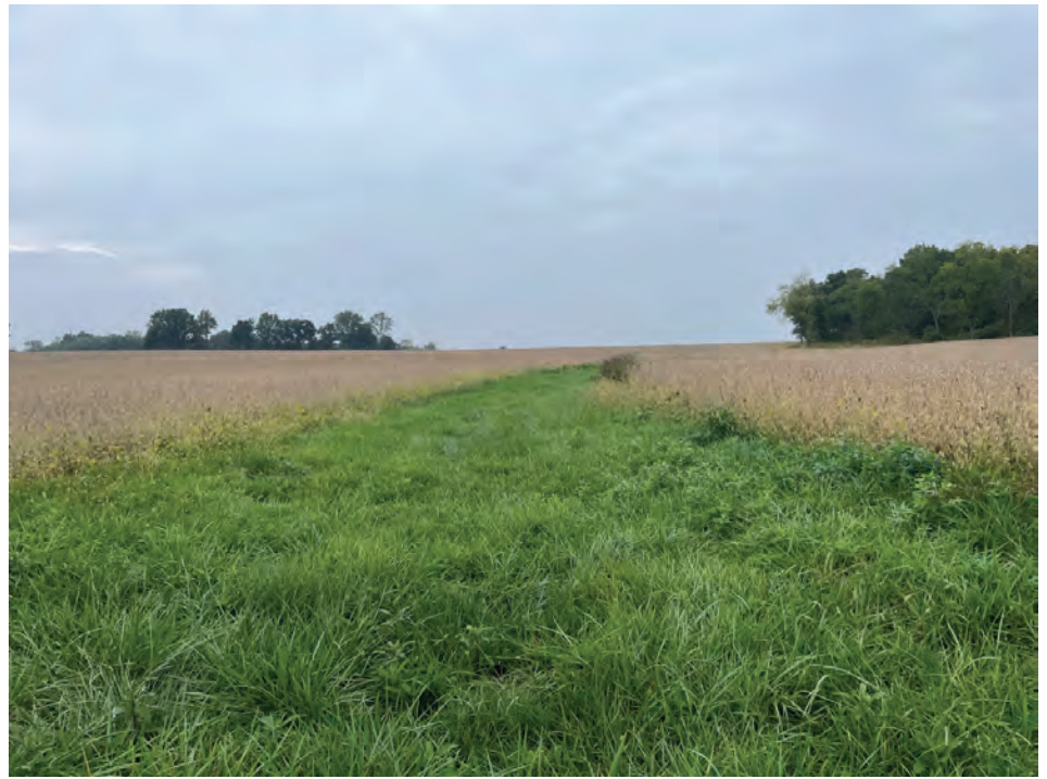
14. Looking W along grass swale on the W side of SR 1 (10/6/2021)
