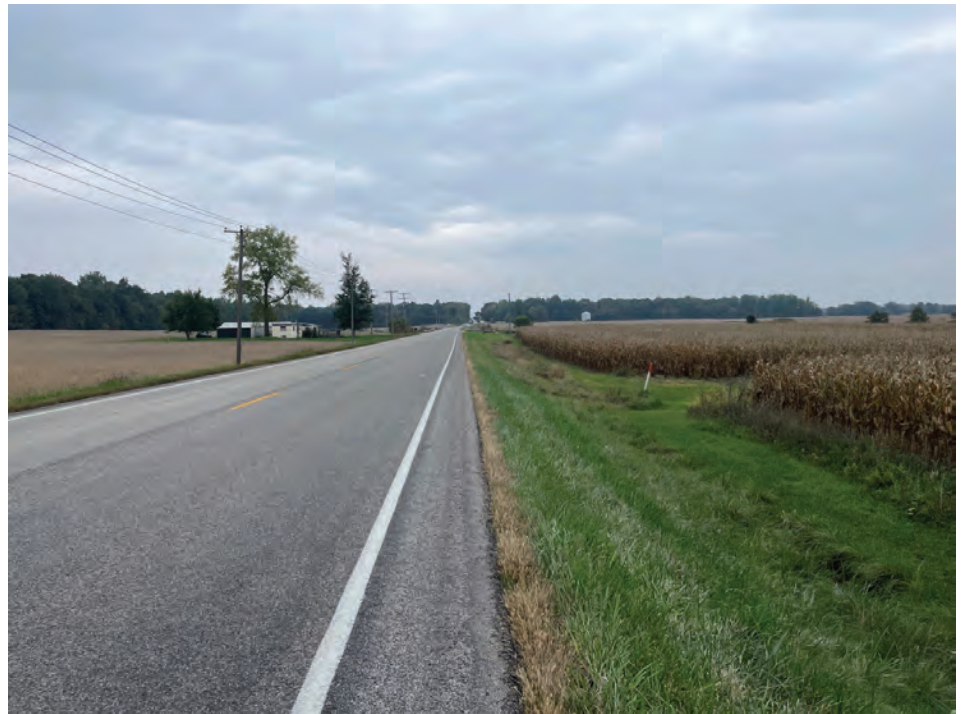
16. Looking N along the E side of SR 1 towards small structure (10/6/2021)
