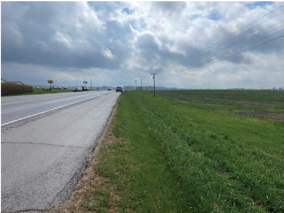
55. Looking S along the W side of US 27 (10/15/2021)
