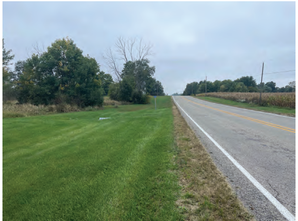
40. Looking W along the S side of SR 26 towards the small structure (10/6/2021)
