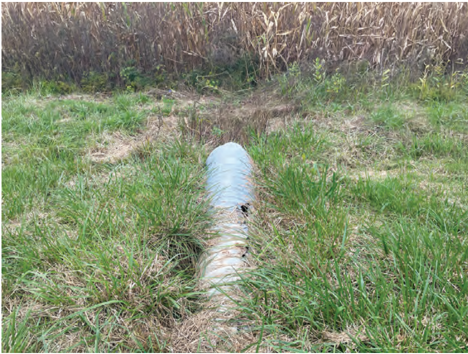
41. Looking N from SR 26 along the small structure (10/6/2021)
