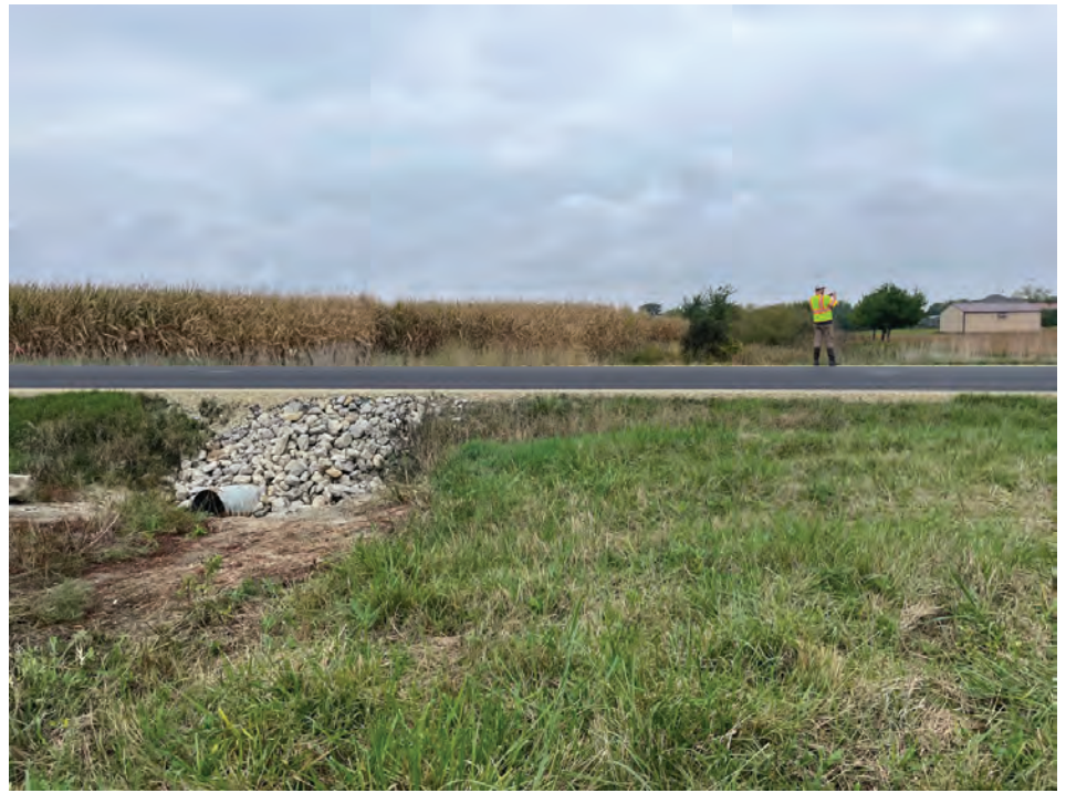
6. Looking N towards SR 1 and the small structure inlet (10/4/2021)
