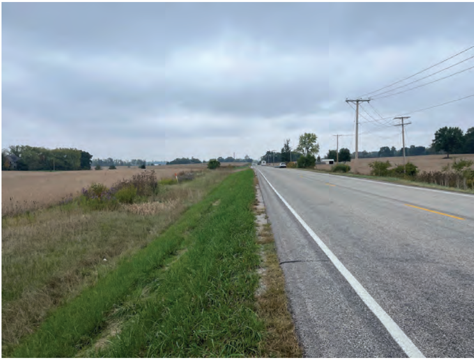
37. Looking S along the E side of SR 1 (10/6/2021)
