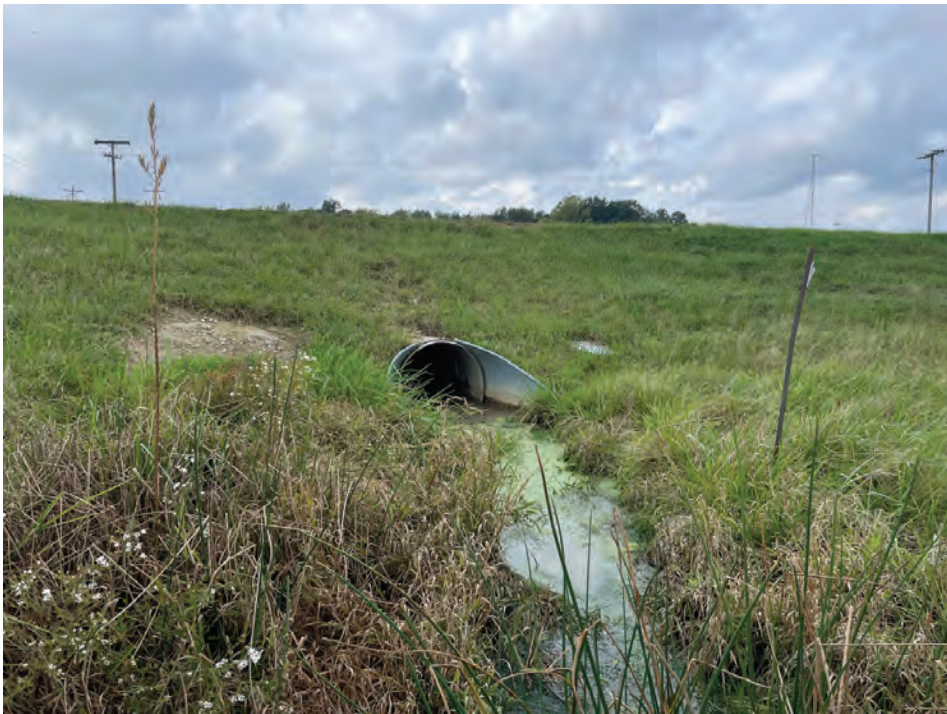
67. Looking W towards structure in northeast quadrant of intersection (10/15/2021)
