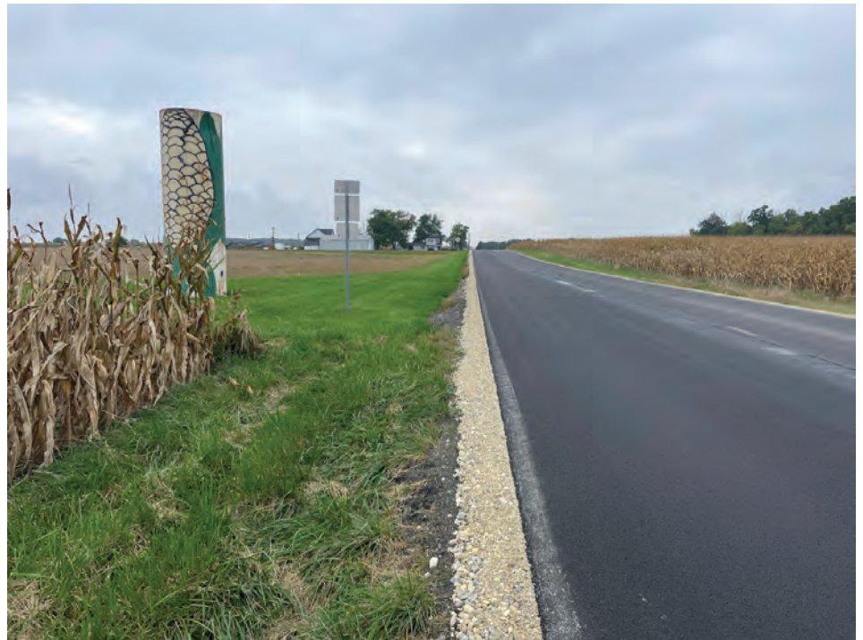
10. Looking W along the S side of SR 1 (10/4/2021)
