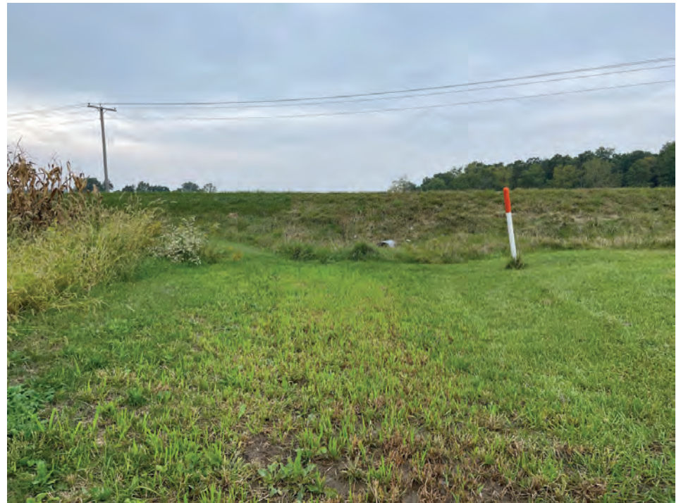
20. Looking W toward the small structure along the grass swale (10/6/2021)
