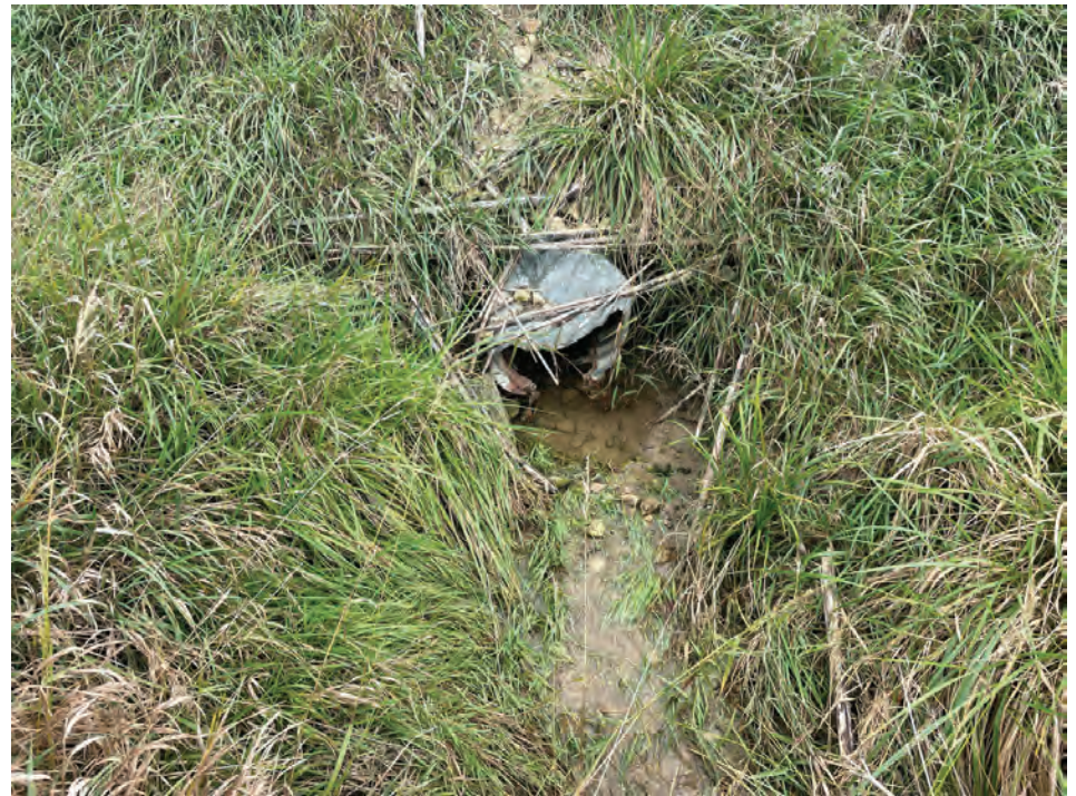
35. Looking W at the small structure outlet (10/6/2021)
