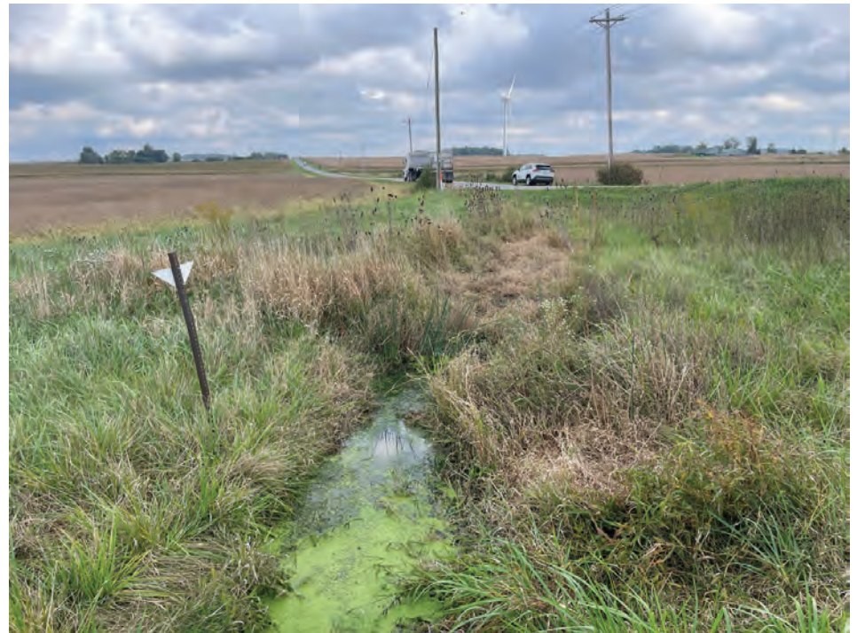
68. Looking SE along wetland from structure outlet (10/15/2021)
