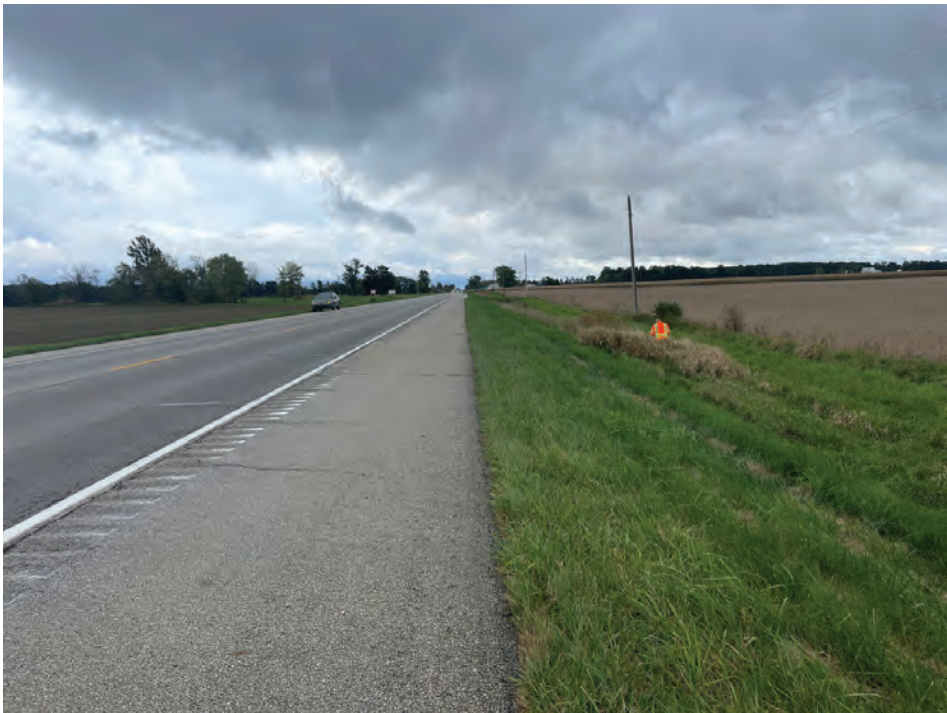
79. Looking S along the W side of US 27 (10/15/2021)
