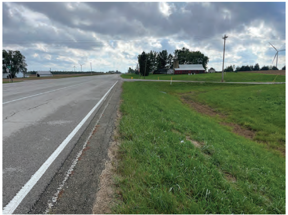
70. Looking S along the W side of US 27 (10/15/2021)
