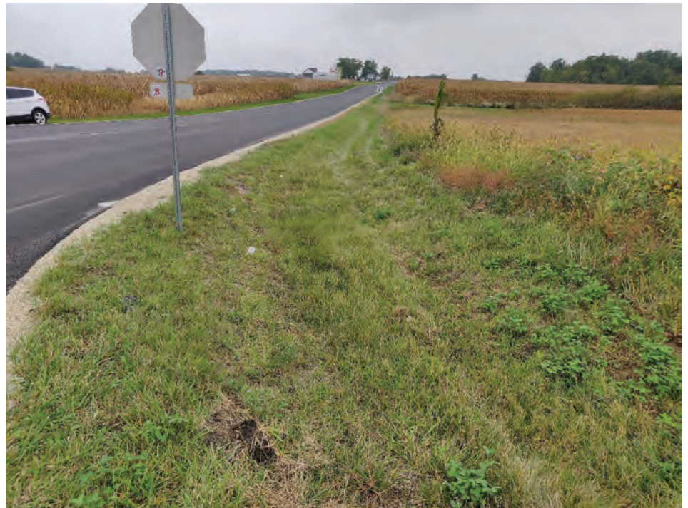
4. Looking W along the N side SR 1 (10/4/2021)
