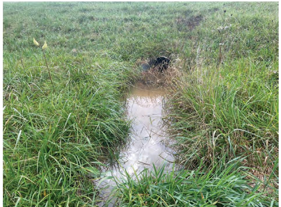
60. Looking W towards the small structure outlet (10/15/2021)
