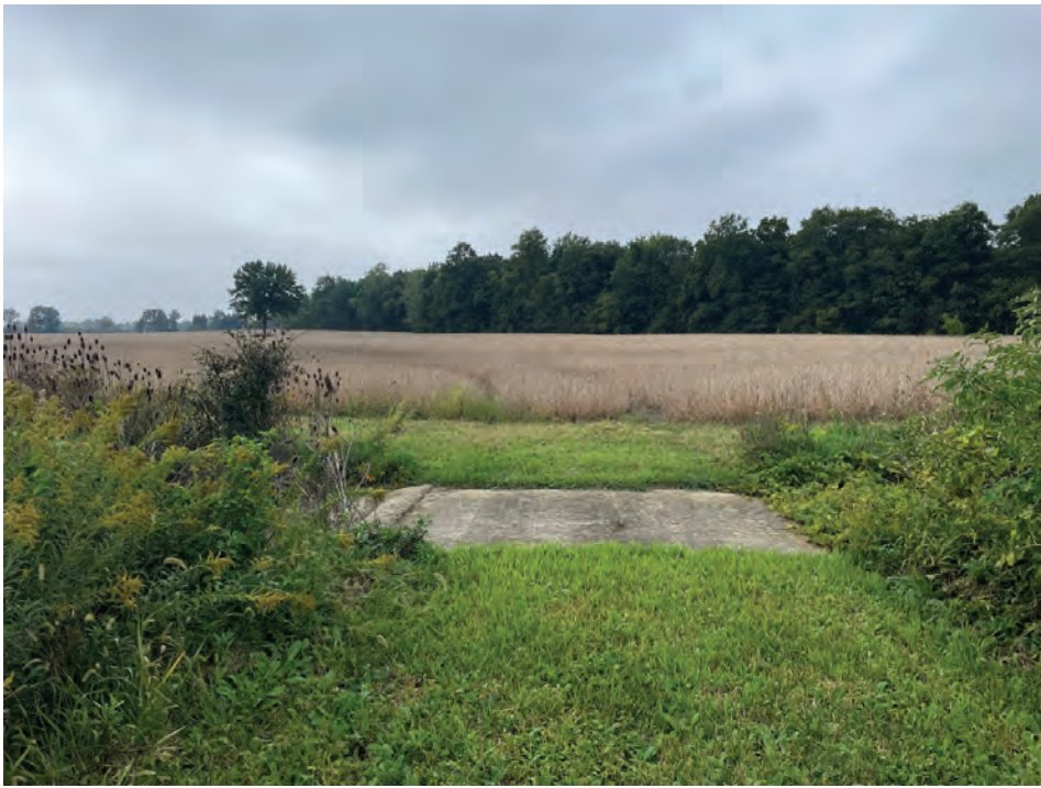
29. Looking SW across field access culvert carrying UNT 2 to McClain Ditch (10/6/2021)
