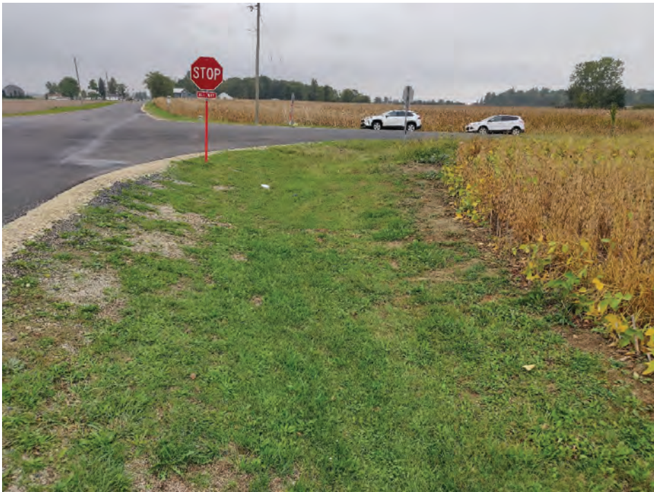
3. Looking S along the W side CR 800 W towards SR 1 (10/4/2021)
