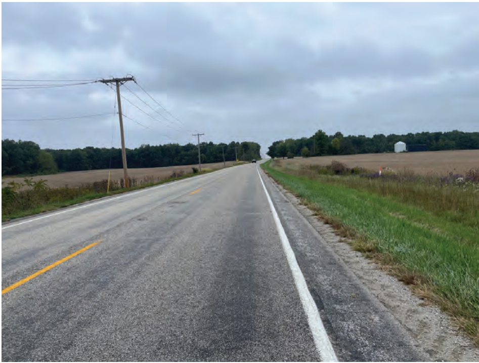
25. Looking N along the E side of SR 1 (10/6/2021)
