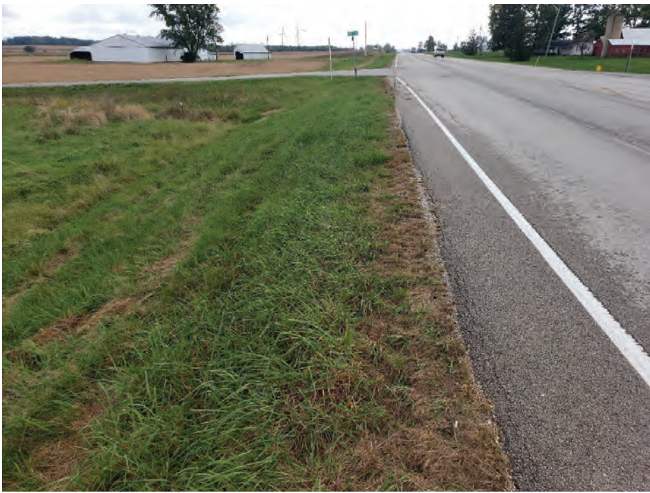
69. Looking S along the E side of US 27 (10/15/2021)
