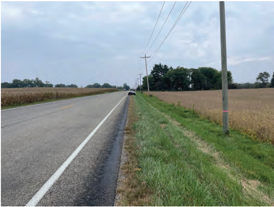
13. Looking S along the W side of SR 1 (10/6/2021)
