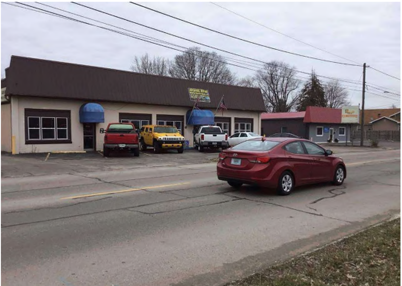
100 Looking northeast at c. 1950 “Non-contributing” commercial buildings along Main Street.
