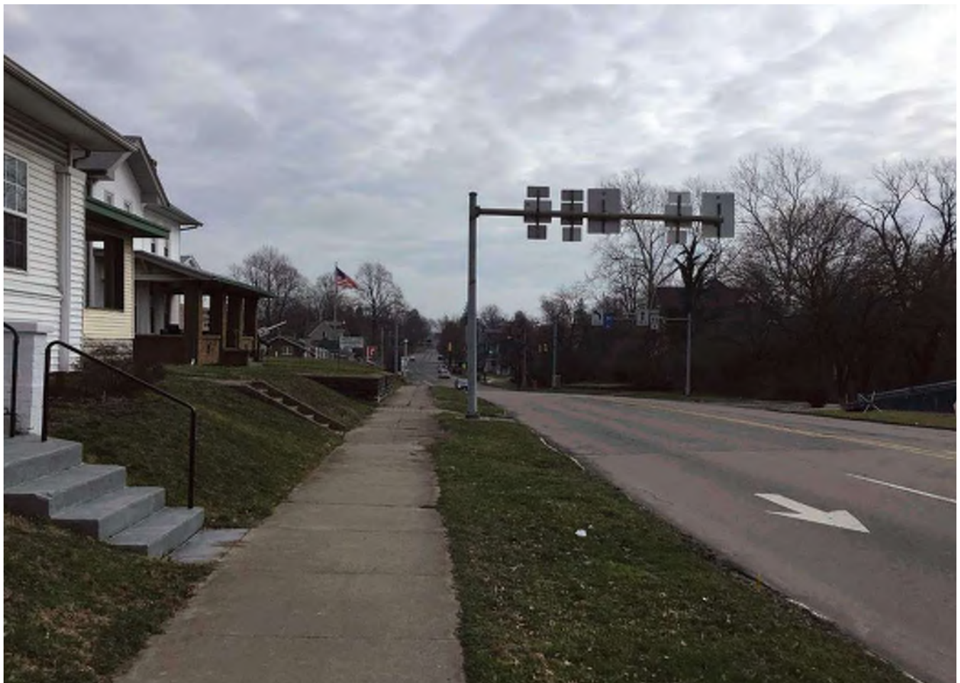
52 Looking east along E. Main Street between East Street and Lincoln Street.
