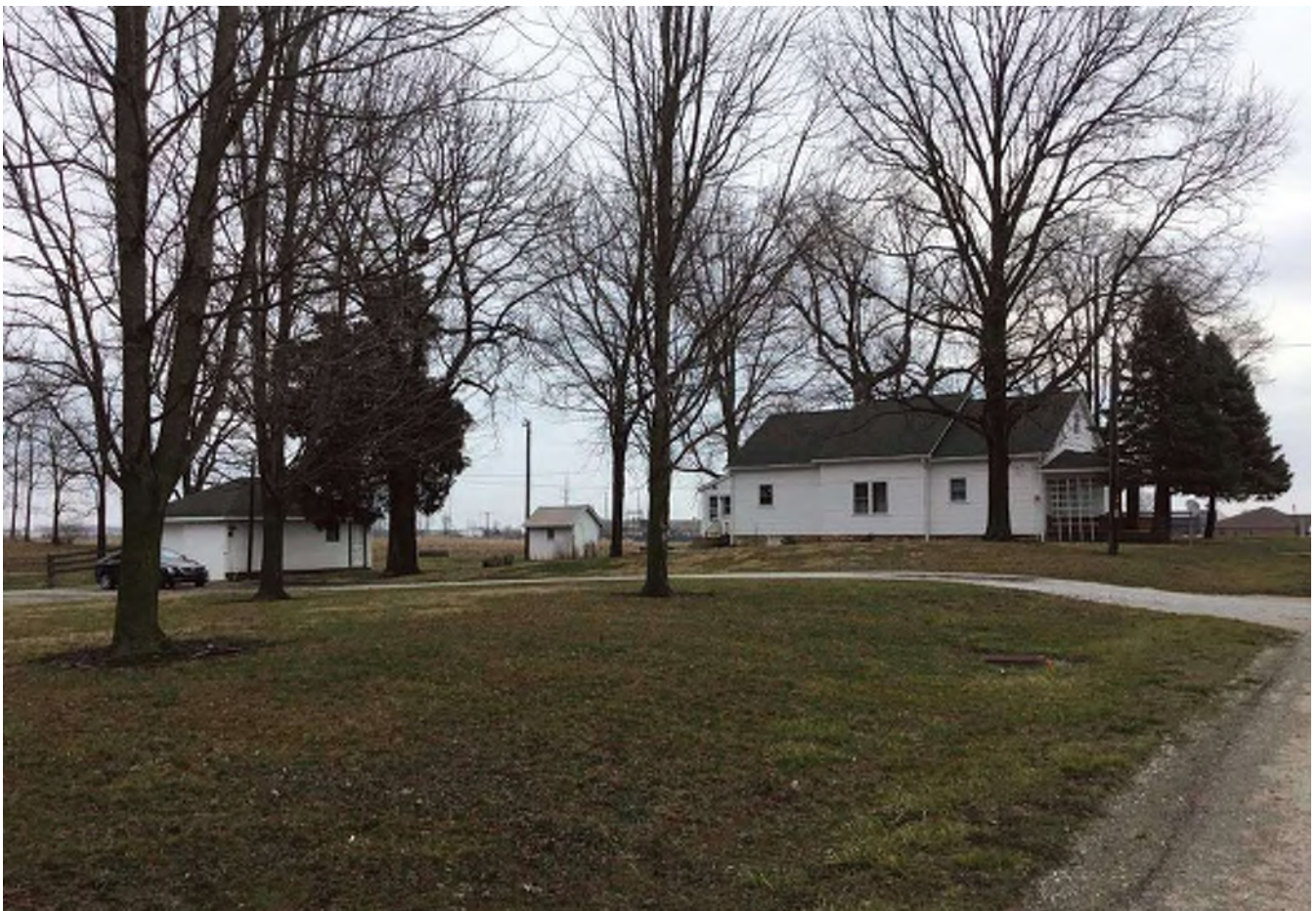
16 Looking northeast at c.1900 "Contributing" farm (RQAW # 4) at 1520 W. State Road 46 (Main Street) with altered porch and additions.
