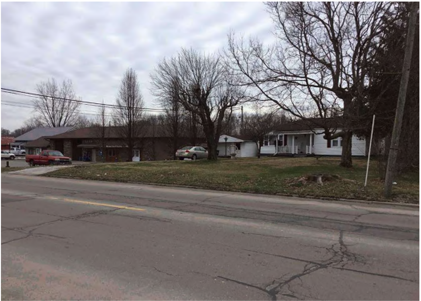
99 Looking southeast at c. 1945 “Non-contributing” house and commercial building along Main Street.
