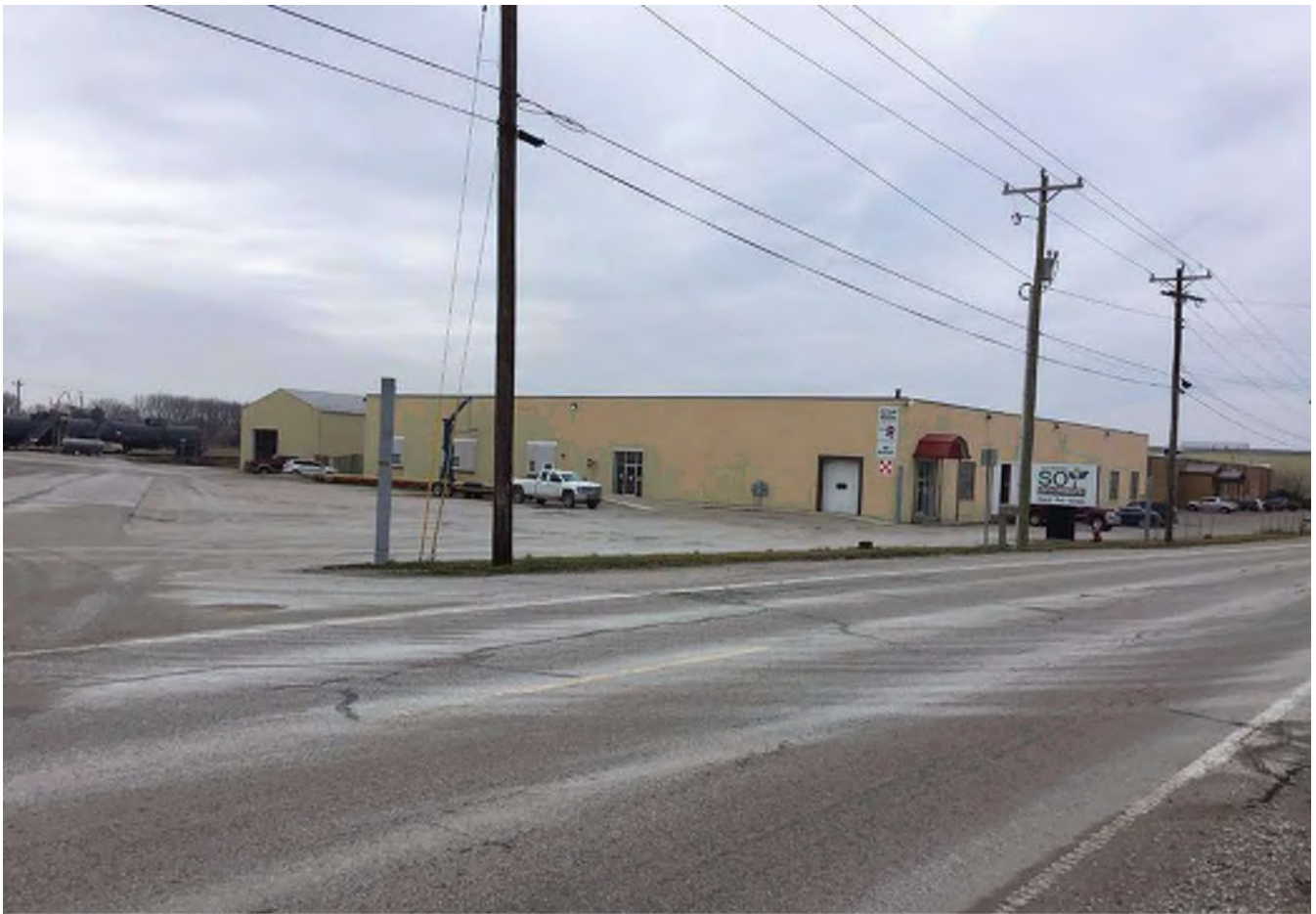
27 Looking south at “Contributing” c. 1958, 1964, and 1971 industrial buildings (RQAW #6) at 1115 W. Main Street (SR 46).
