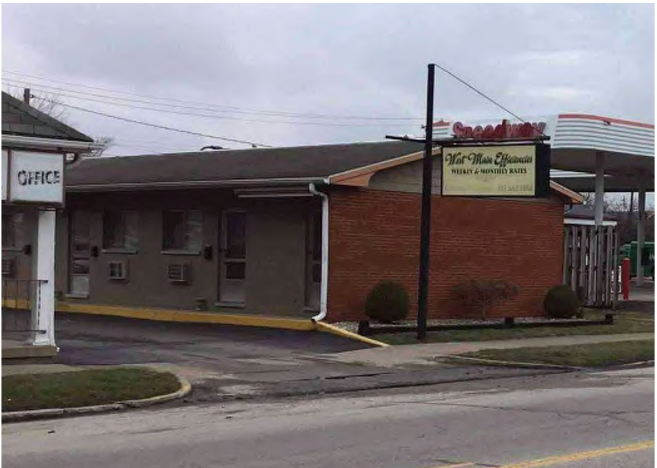
44 Looking northeast at c. 1963 “Non-Contributing” motel at 426 W. Main Street.
