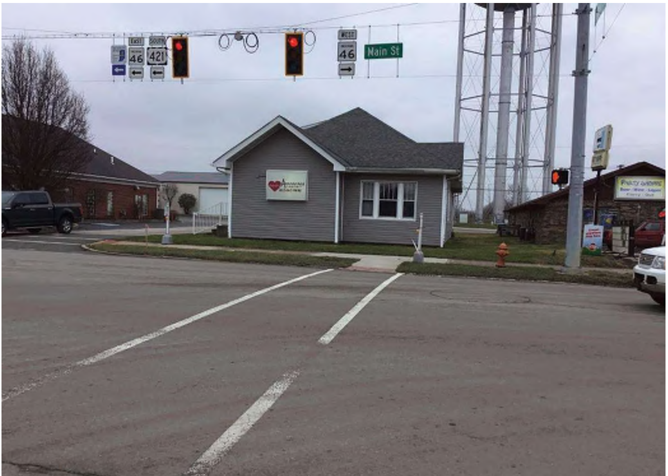
48 Looking south at “Non-contributing” house at 342 W. Main Street.
