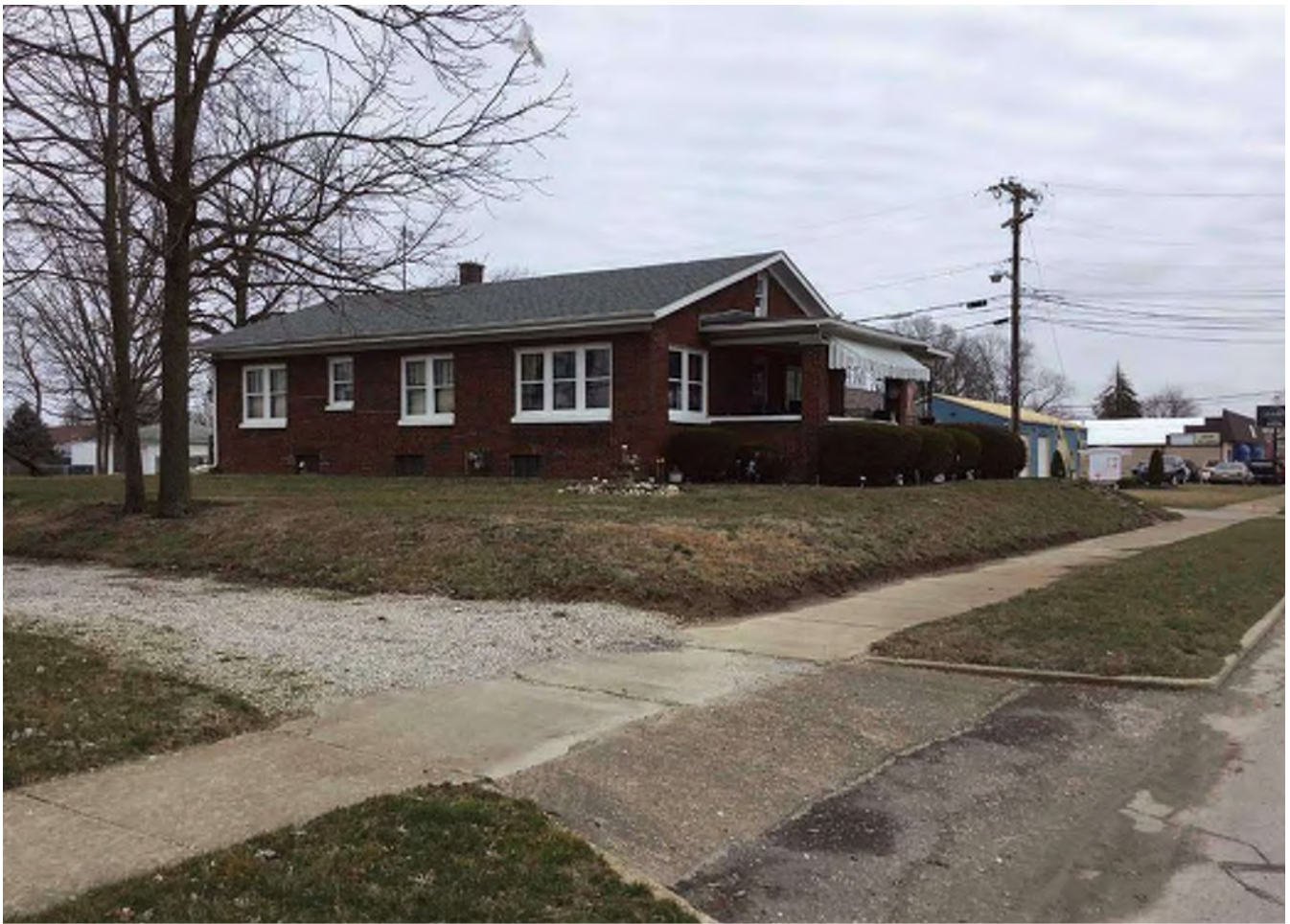
97 Looking northeast at “Contributing” Bungalow (RQAW # 14) at 940 E. Main Street.
