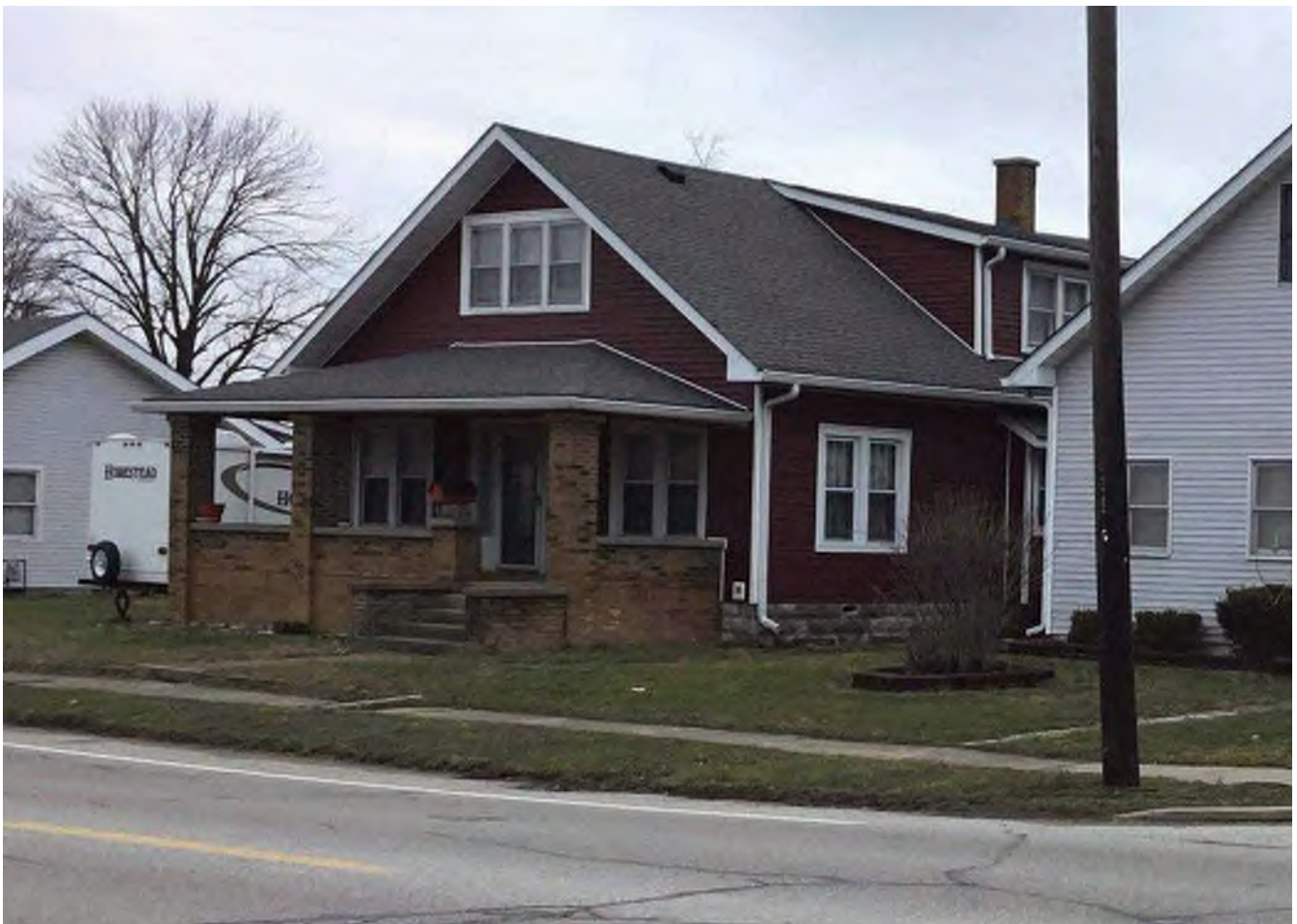
38 Looking northwest at “Contributing” (RQAW # 7) at 606 W. Main Street.
