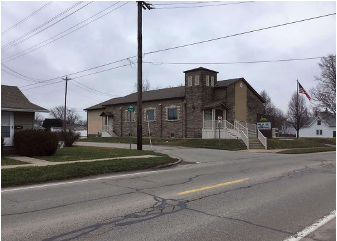
33 Looking at c. 1950 “Non-contributing” church with alterations at 634 W. Main St.
