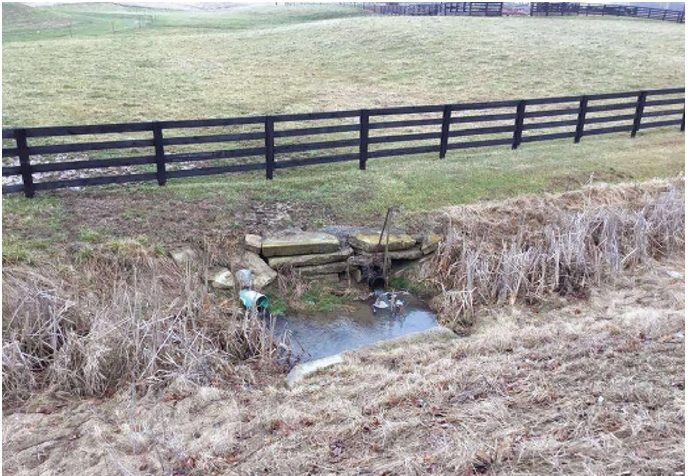
6 Looking northeast at the top of “Non-contributing” concrete headwall for drainage pipe running under SR 46, and stacked pieces of broken concrete as headwall to field drain pipe outlet.
