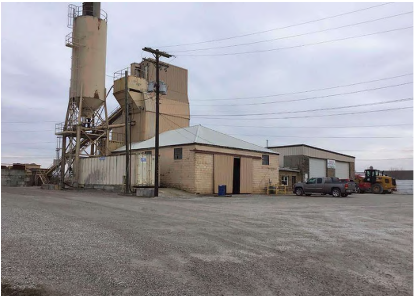
24 Looking south at "Non-contributing" c. 1950 CMU block industrial building at 1100 W. Main Street (SR 46).
