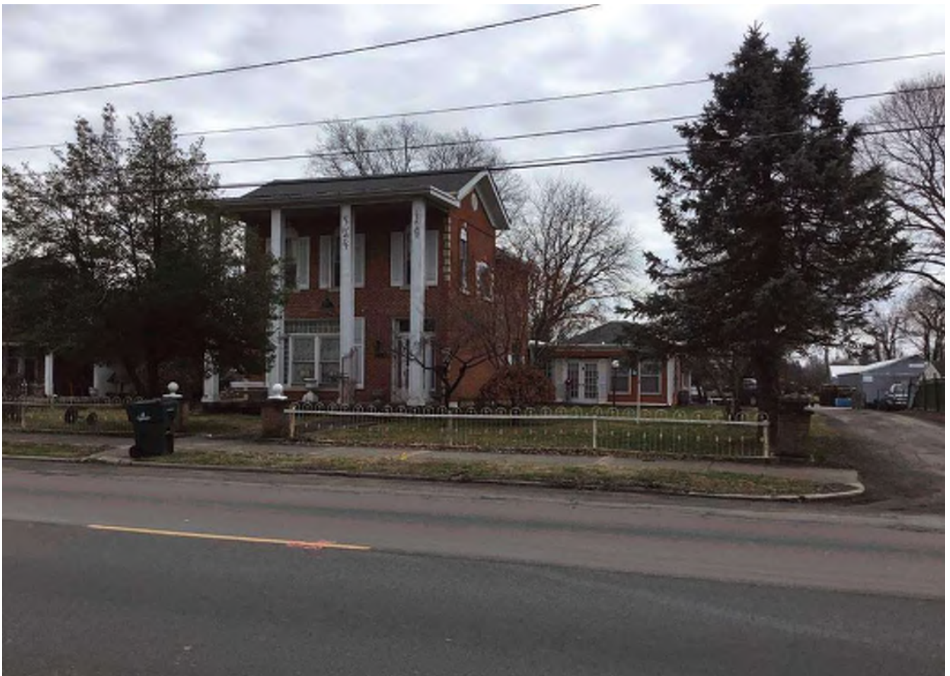
92 Looking southeast at not recommended eligible “Notable” house (RQAW # 10) at 319 E. Main Street.
