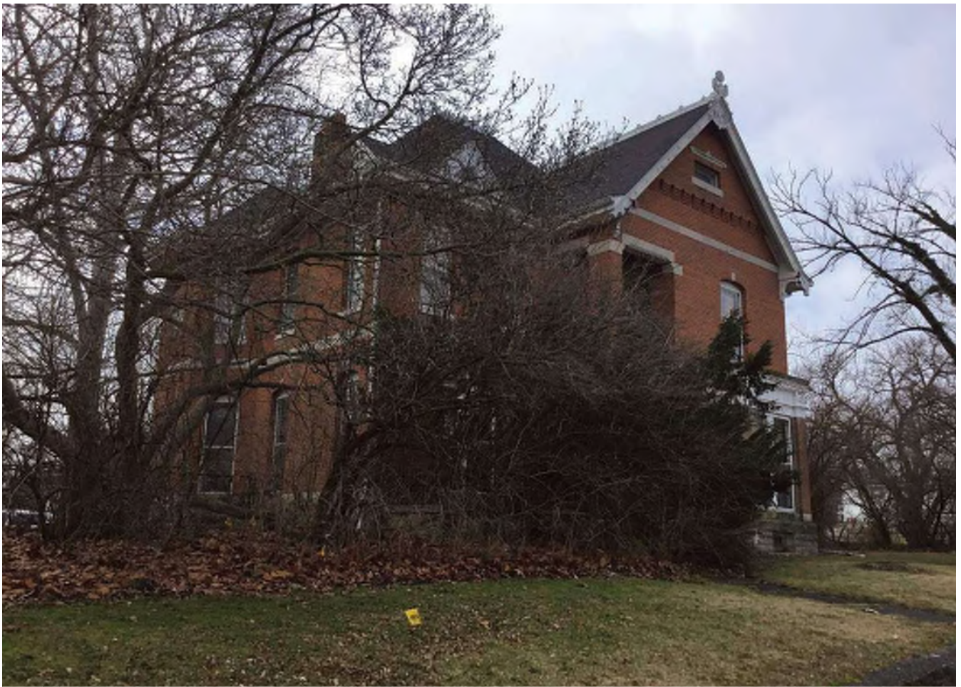
57 Looking southwest at the State Register-listed Charles Zoller House (NR-0308).
