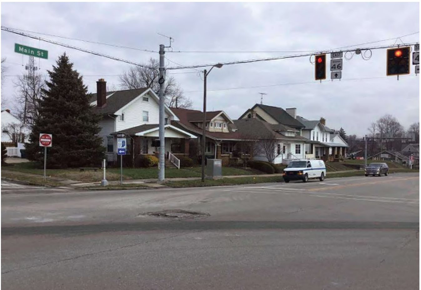
50. Looking northeast at “Contributing” Craftsman Bungalow (RQAW # 9) at 308 E. Main Street and “Non-contributing” houses east of East Street.
