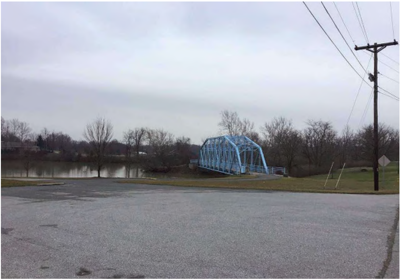
5 Looking southeast outside of the APE at the 1915 pedestrian steel truss “Boyd Bridge” (Decatur County Bridge 140, NBI 1600116) relocated in 2006 over Muddy Fork of Sand Creek in Decatur County Park at 1650 W. Park Rd.
