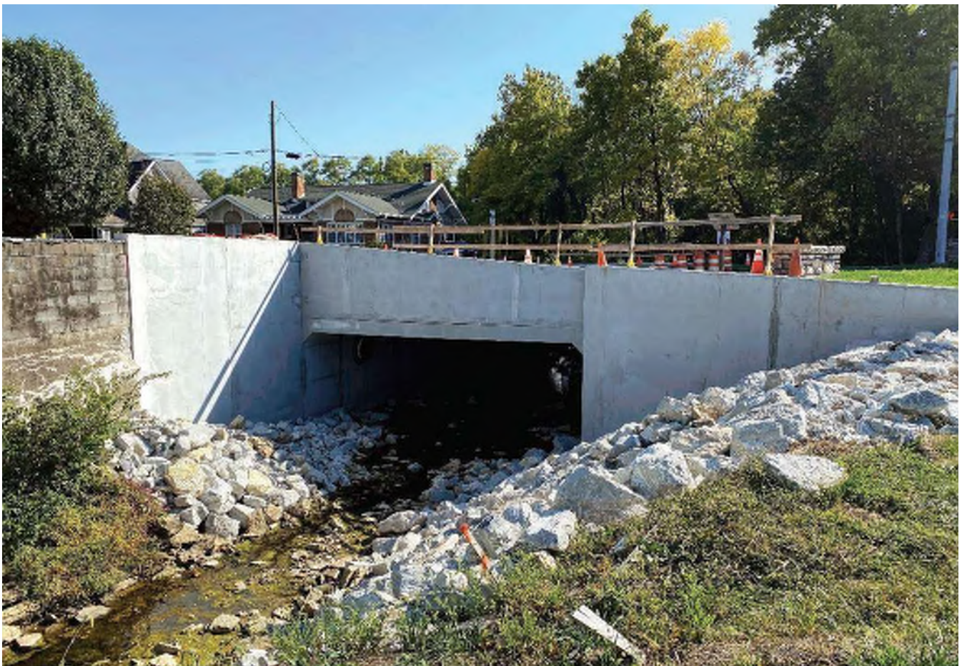
62. October 2020 photo looking southeast at the new concrete bridge within the Greensburg Eastside Residential Historic District. The bridge original stone arch bridge was replaced in the summer of 2020.
