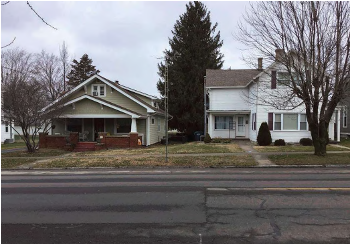
79 Looking north at “Contributing” and “Non-contributing” houses within the recommended National Register-eligible Greensburg Eastside Residential Historic District. Note limestone curbs.
