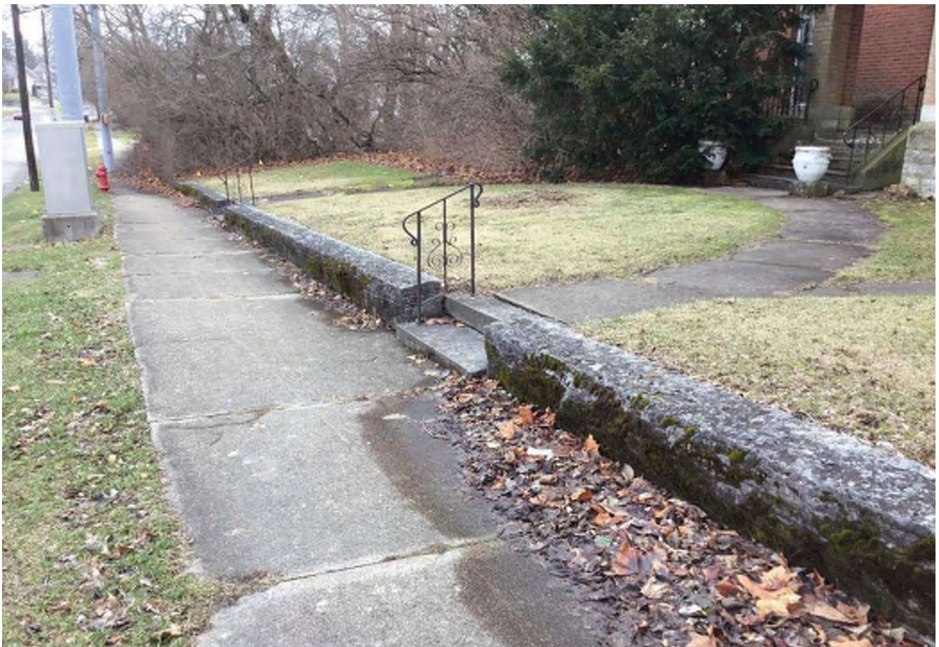
56 Looking southeast at the limestone wall and steps in front of the State Register-listed Charles Zoller House (NR-0308) property.
