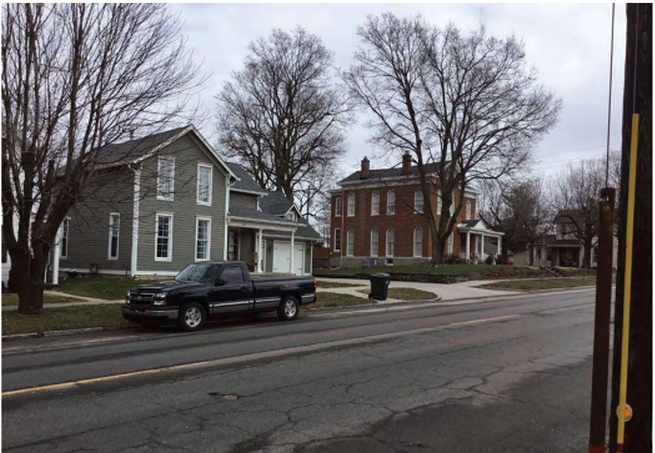
80 Looking northeast at “Notable” and “Contributing” houses west of Wilder Street within the recommended National Register-eligible Greensburg Eastside Residential Historic District.
