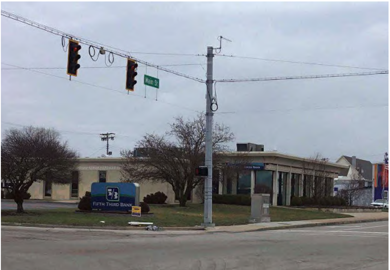
47 Looking northeast across the Main Street (SR 46) and US 421 (Ireland Street) intersection at the c. 1973 “Contributing” bank (RQAW # 8).
