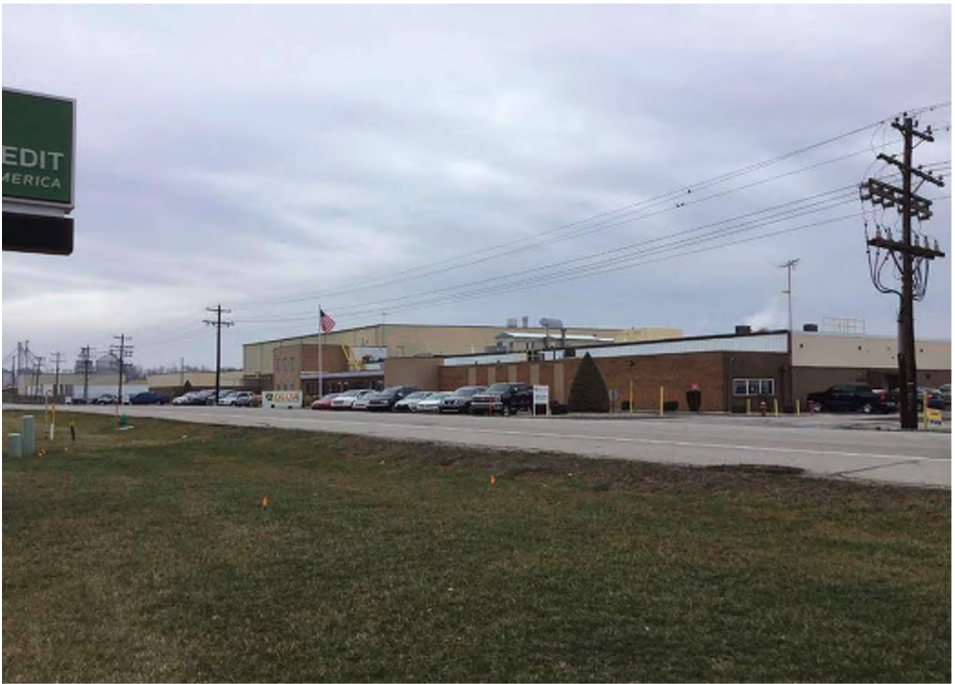
19 Looking south at “Non-contributing” c. 1958 industrial building at 1425 W. Main Street (SR 46).
