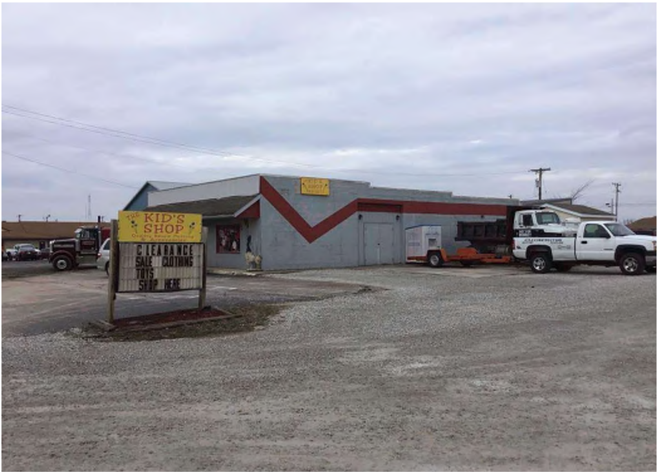
25 Looking northwest at “Non-contributing” c. 1950 CMU block industrial building at 1206 W. Main Street (SR 46).
