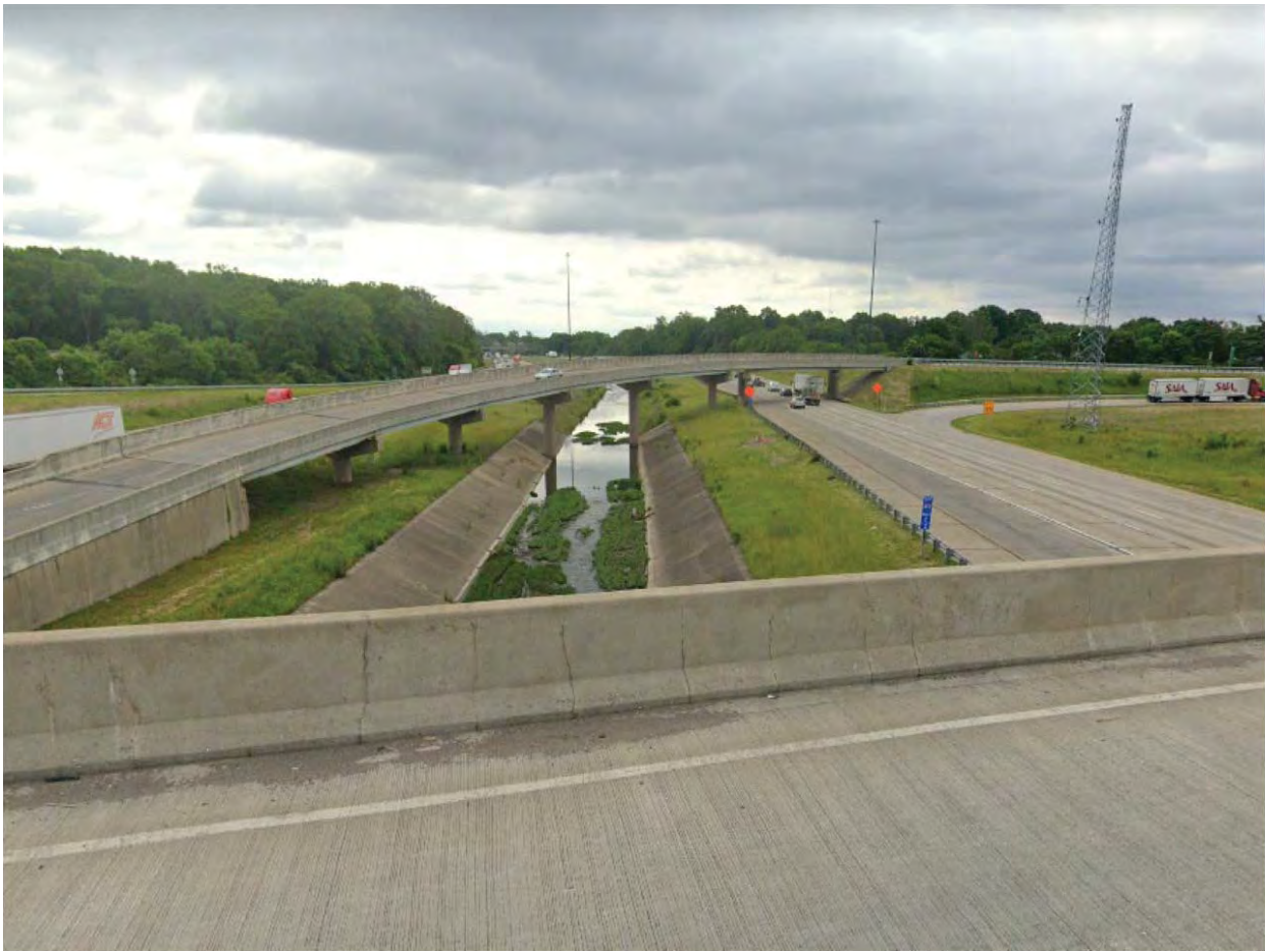
3. Looking southeast to I-465 from US 31
