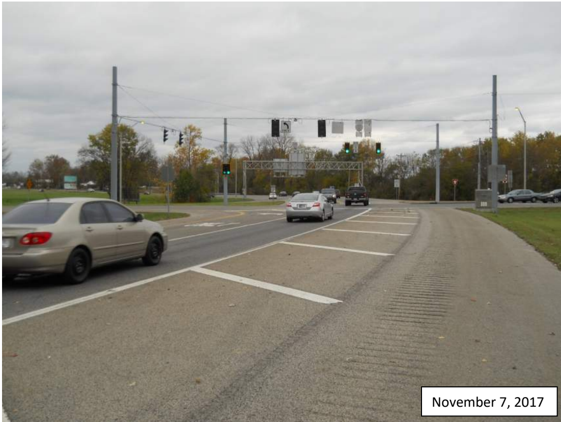
Photograph #11: Looking southwest along SR 46 toward intersection with SR 11.
