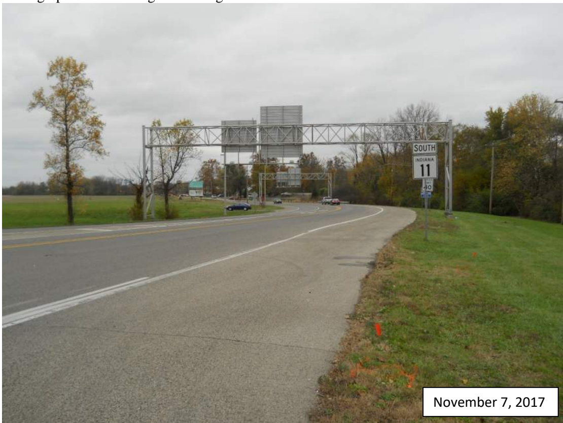
Photograph #18: Looking south along SR 11.
