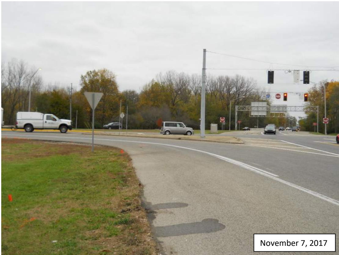
Photograph #19: Looking north towards SR 46 right-turn lane onto SR 11.
