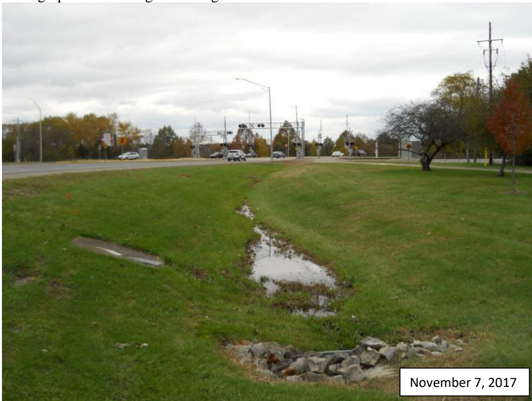
Photograph #6: Looking west along roadside ditch #1.
