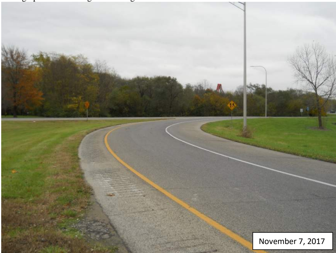
Photograph #22: Looking north along SR 11 ramp to SR 46.
