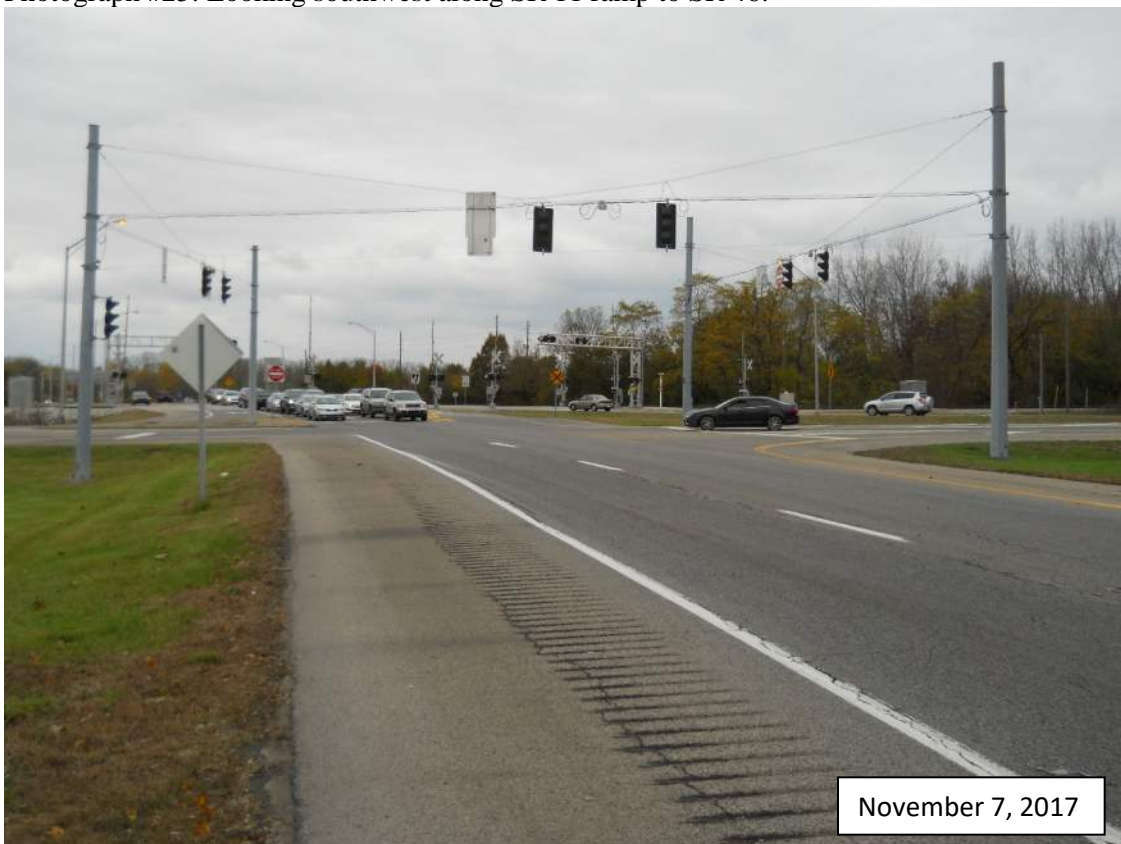
Photograph #26: Looking west toward SR 46 intersection with SR 11.
