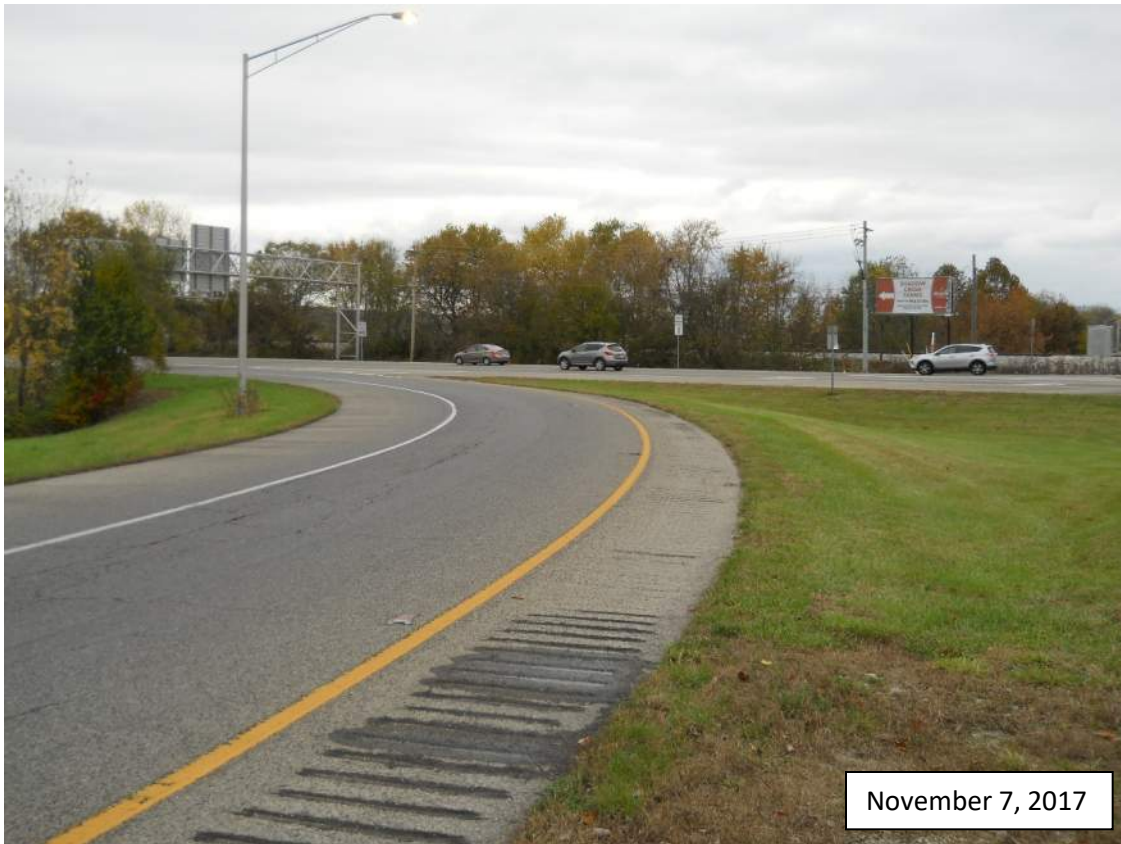
Photograph #25: Looking southwest along SR 11 ramp to SR 46.
