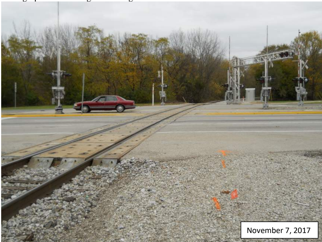
Photograph #2: Looking north along Louisville & Indiana Railroad.
