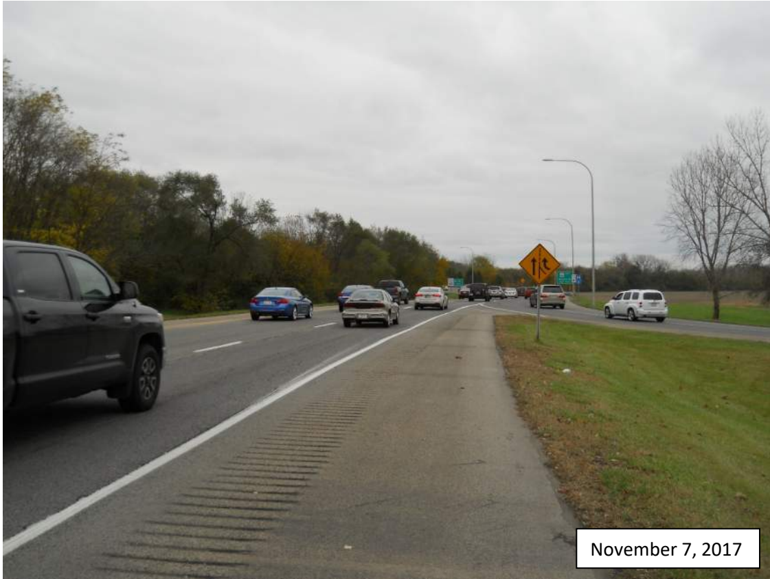
Photograph #27: Looking east along SR 46.
