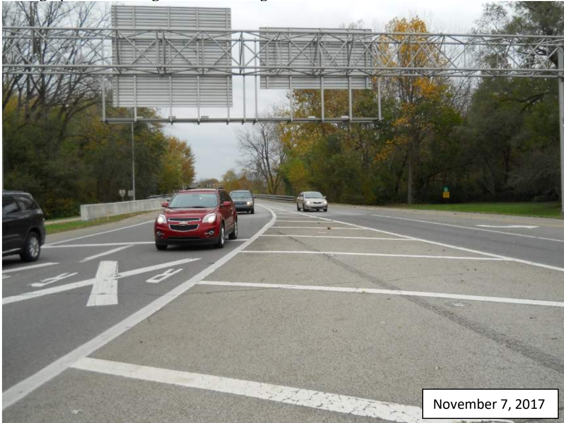
Photograph #10: Looking northeast along SR 46 toward Flatrock River.
