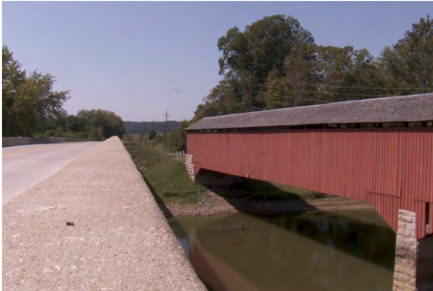
Jackson County's Medora Covered Bridge runs parallel with St. Road 235 and crosses over The East Fork White River. (Seth Tackett, WTIU/WFIU News)
