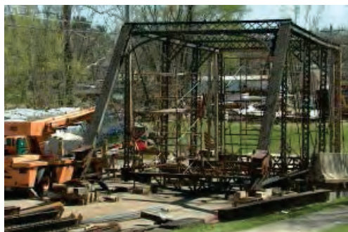
Historic Paoli Bridge Repaired, Still Closed To Traffic
