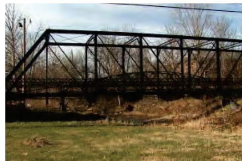
Re-Opening Of Historic Paoli Bridge Planned For Early 2018
