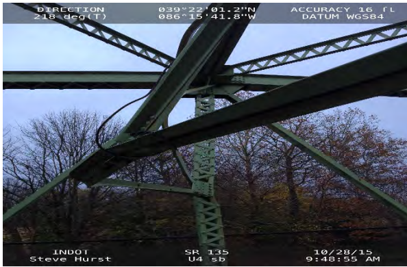
L4U4 West Truss facing West
