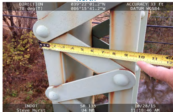
L4U4 East Truss at UC facing East
