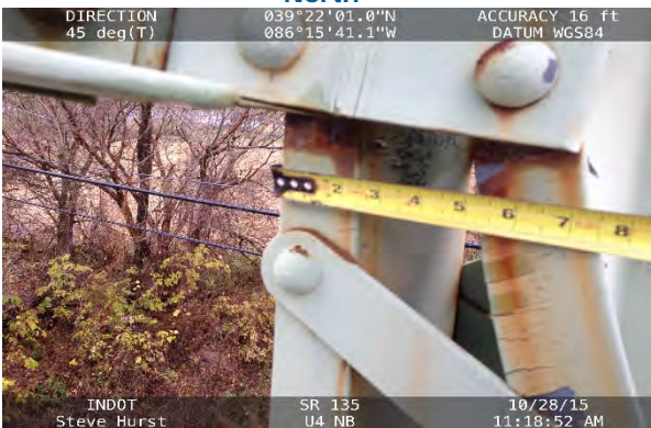
L4U4 East Truss at Sway Bracing facing East
