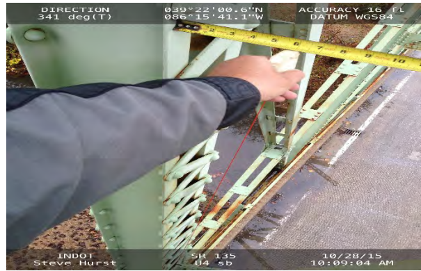
L4U4 West Truss Vert Meas 1
