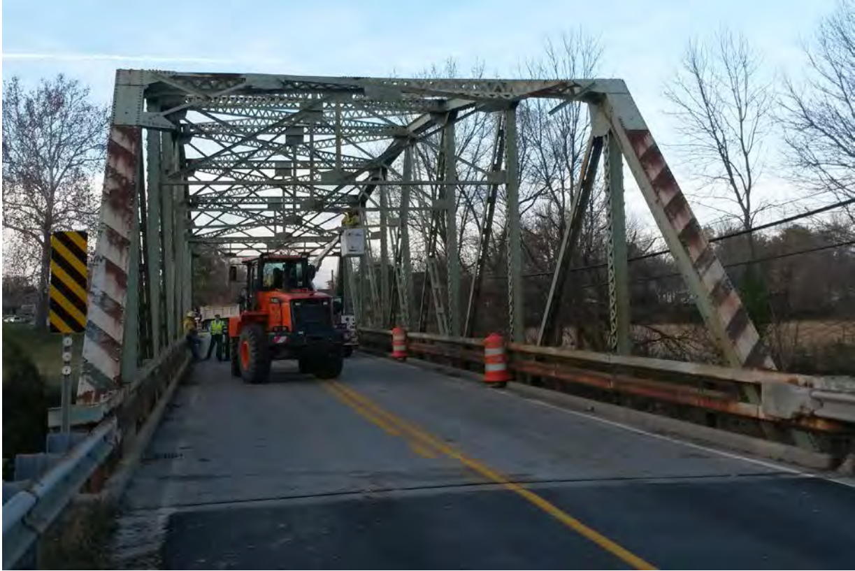
South portal after removal of damaged pieces
