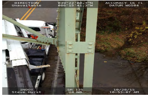
L3U4 East Truss (L4U4 Background) facing North
