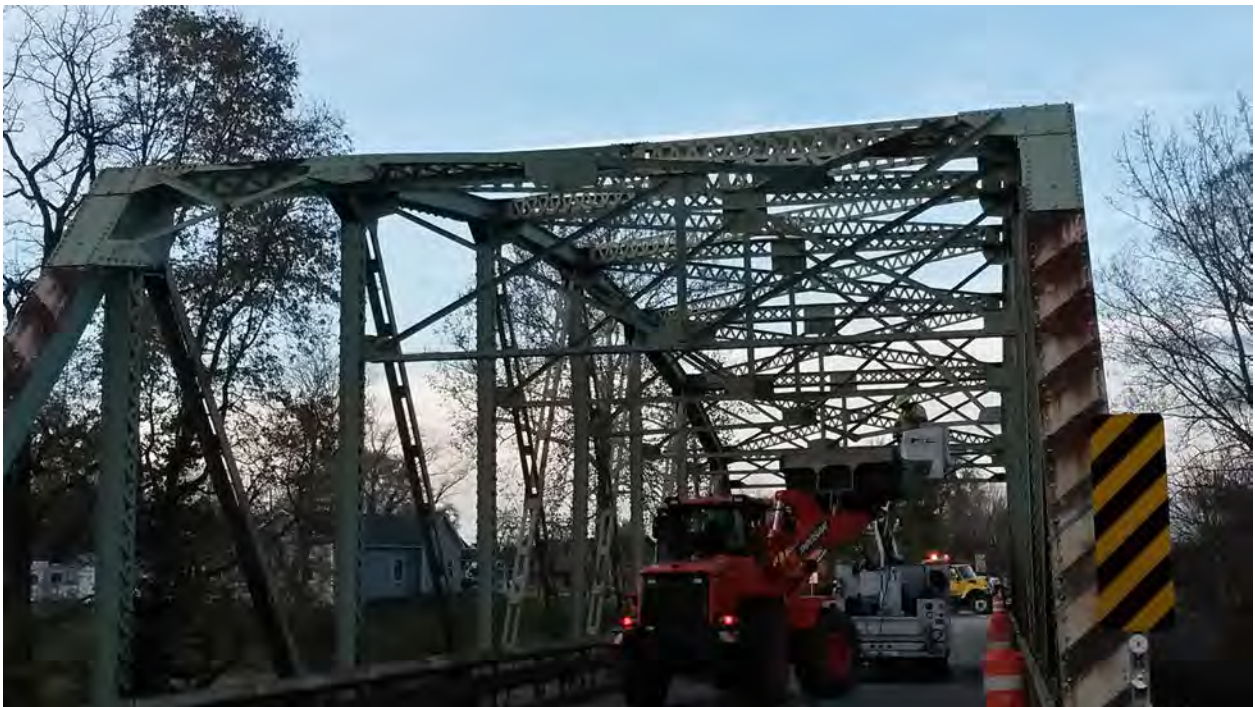
South portal after removal of damaged pieces
