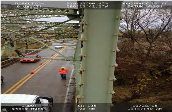
L3U3 East Truss (L4U4 Background) facing North
