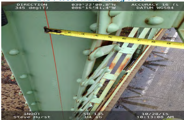
L4U4 West Truss Vert Meas 3
