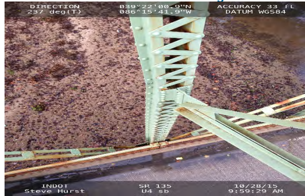
L4U4 west Truss facing Down
