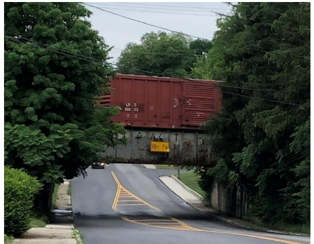
Figure 5-1: Signage at low clearance bridge.
