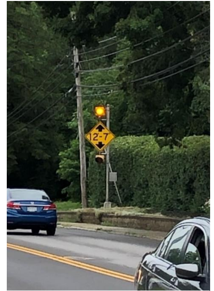
Figure 5-4: 24-7 Flashing Beacon with Clearance Sign
