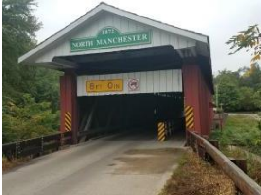
Figure 4-3: Vertical clearance bar constructed at entrance of North Manchester Covered Bridge in Wabash County, IN.
