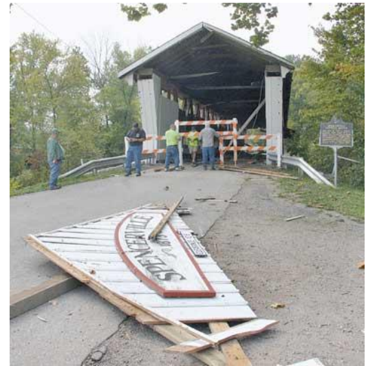
Figure 2-3: Overheight vehicle damage to DeKalb County Bridge No. 3 (Bridge No. 17-00003; NBI No. 1700004). September 2012. (KPC News)
