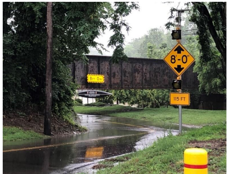
Figure 5-6: Advance signage with sensor-triggered flashing lights and static signage on low clearance bridge.
