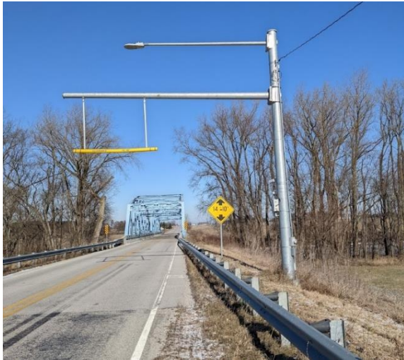
Figure 4-6: Flexible vertical clearance bar ahead of bridge on in Wells County, IN
