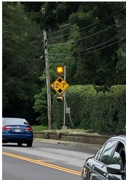
Figure 4-1: 24-7 Flashing Beacon with Clearance Sign
