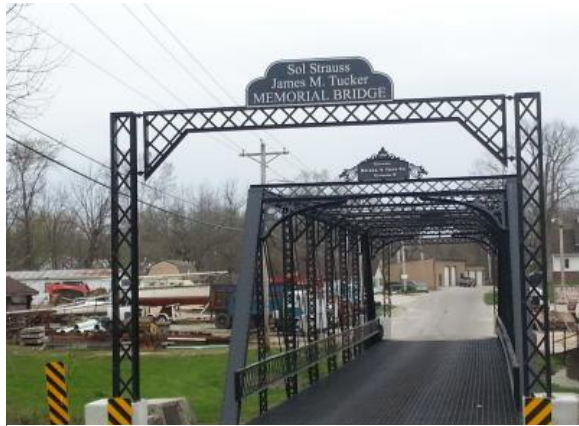
Figure 4-5: Portal frame placed in advance of Gospel Street Bridge in Paoli, Orange County, IN.
