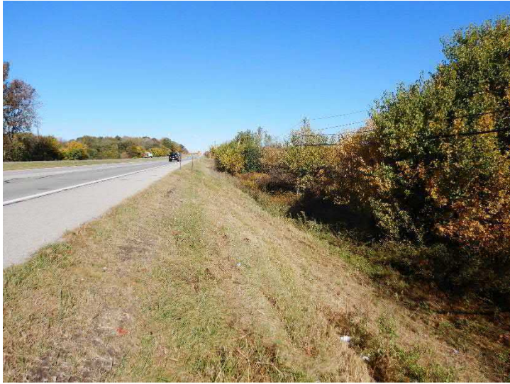
Photo 1: Facing northwest at roadside on east side of US 31
