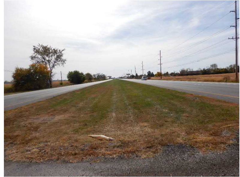
Photo 22: Facing southeast in median of US 31
