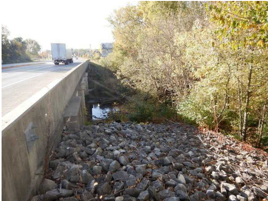
Photo 7: Facing southeast along west side of structure over Youngs Creek
