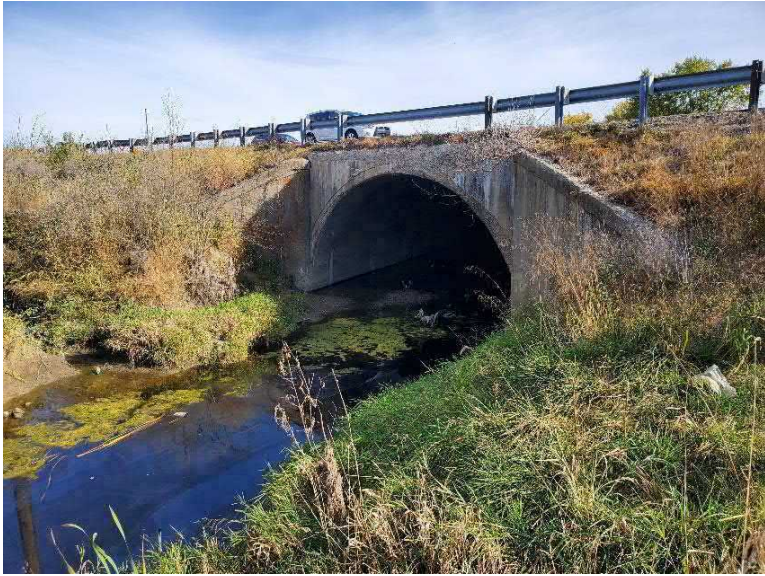
Photo 13: Facing northeast at outlet of structure carrying Canary Ditch under US 31
