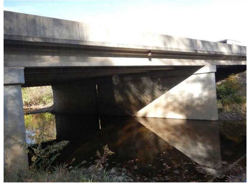
Photo 6: Facing northwest from Youngs Creek
