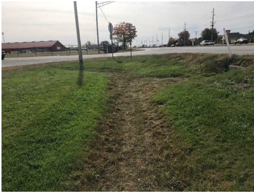
Photo 19: Facing southeast at roadside on east side of US 31
