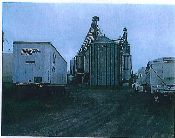
View northwest from north end of 6 th St.
