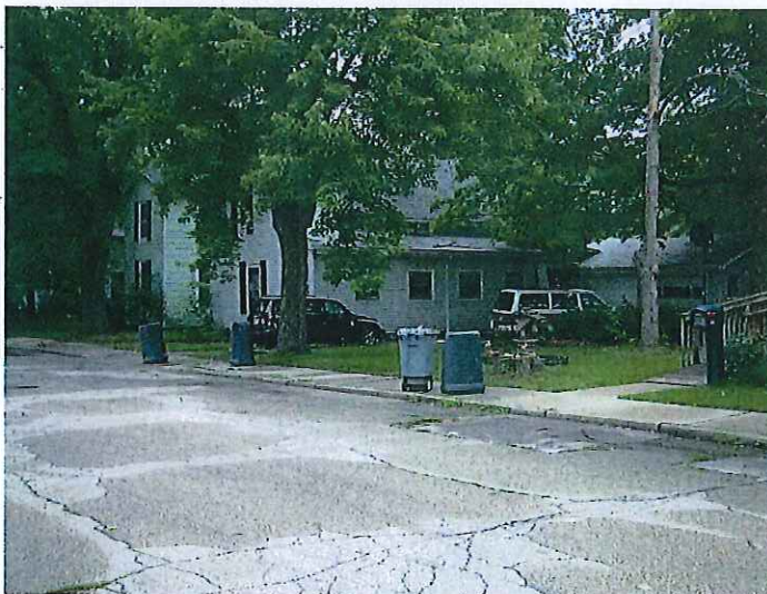
View northwest from Washington St. between 9 th St. and 10 th St.
