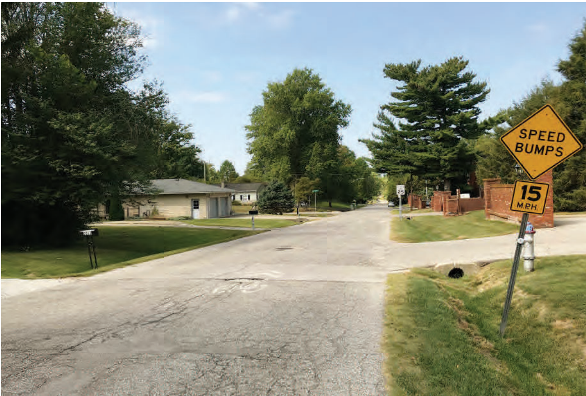
15. Looking west on Morningside Drive
