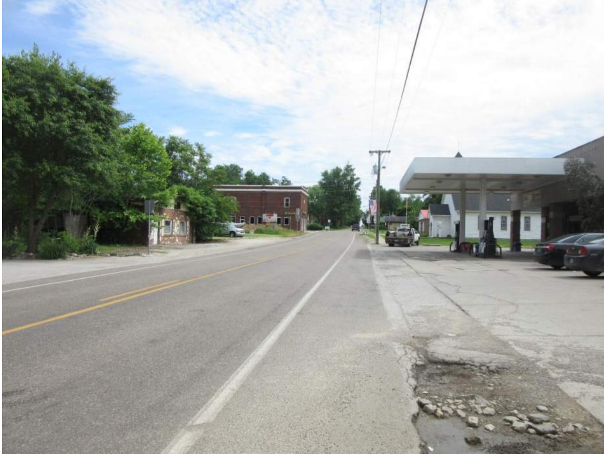
3. From west side of SR 42 looking south down the roadway in Eminence. Photo taken 6/12/19.
