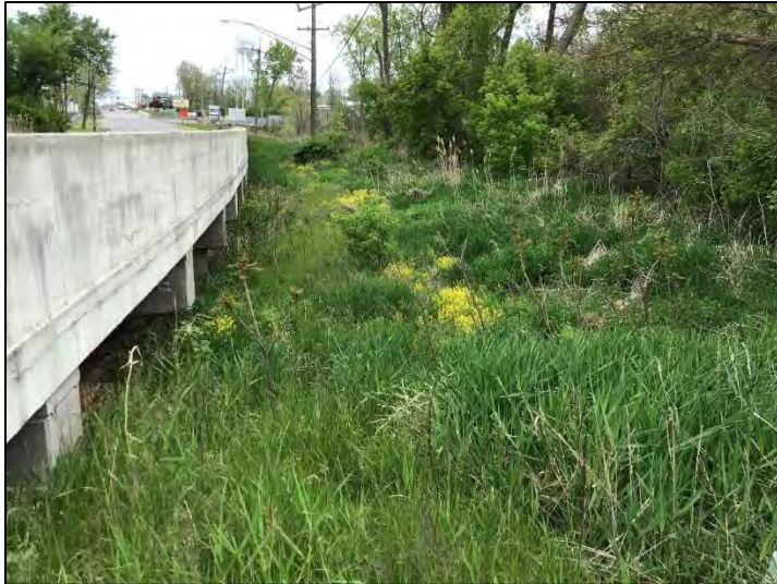
Photo 17. Wetland A east of bridge over Muck Pocket ((6)51-45-01943 B), viewing north, 5/17/2021
