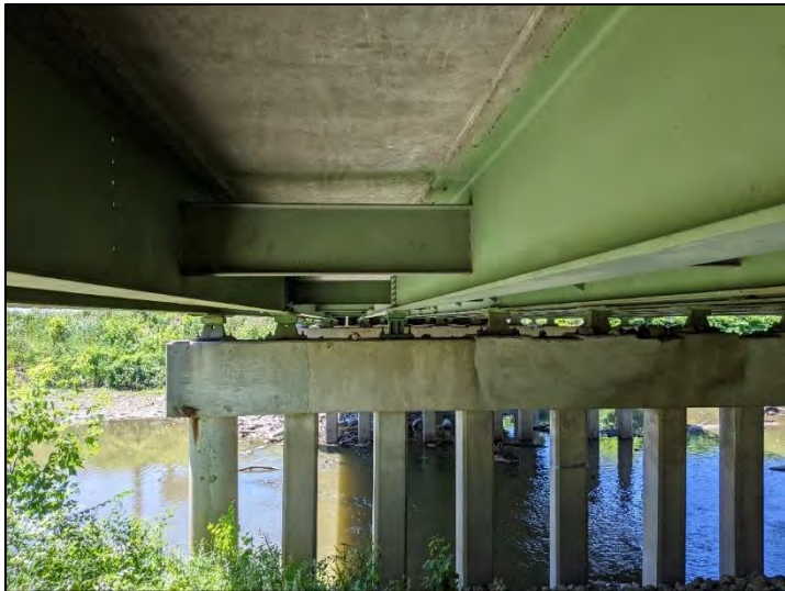
Photo 49. Below bridge over Deep River ((6)51-45-01934 C), viewing north, 6/14/2021
