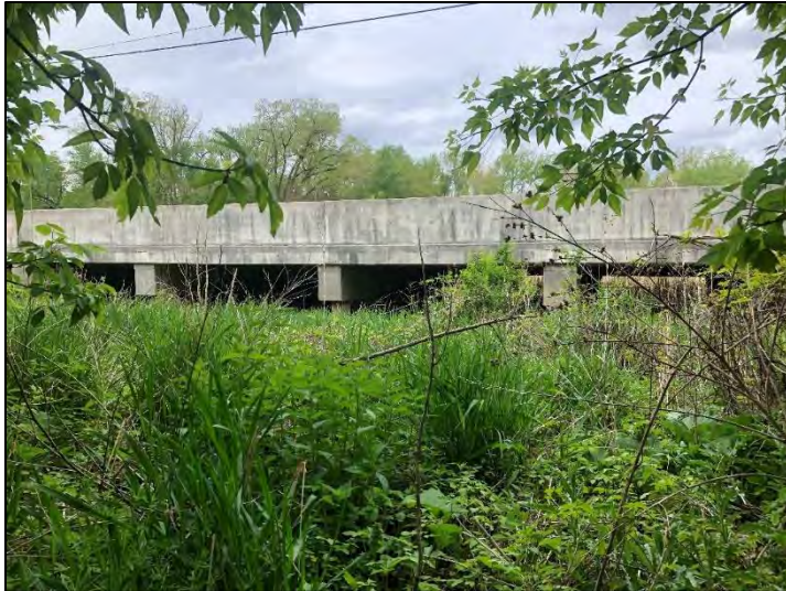
Photo 5. Eastern side of the bridge over Muck Pocket ((6)51-45-01943 B), viewing southwest, 5/17/2021
