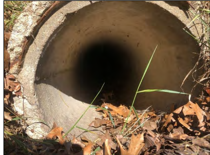
Photo 46. Viewing through inlet of Str. 1, viewing west, 6/14/2021
