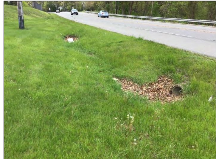
Photo 48. RSD 1 with Str. 1 south of bridge over Muck Pocket, viewing southwest, 5/17/2021
