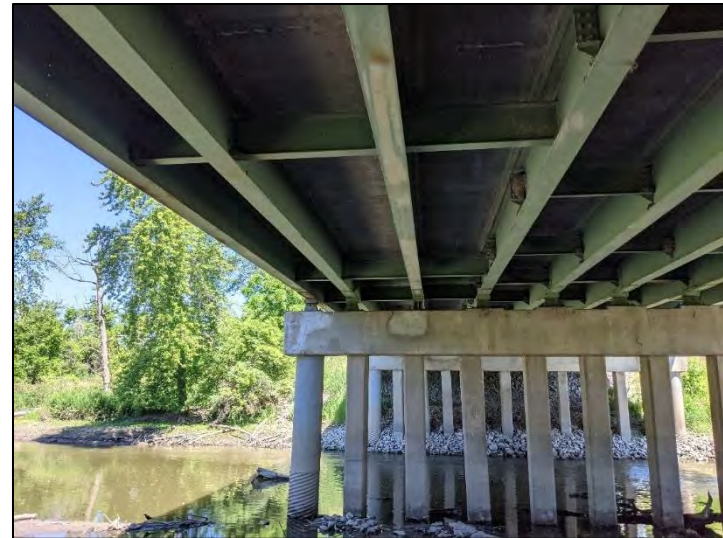
Photo 50. Below bridge over Deep River ((6)51-45-01934 C), viewing north, 6/14/2021
