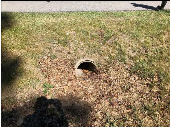
Photo 45. Inlet of Str. 1 south of bridge over Muck Pocket, viewing west, 6/14/2021
