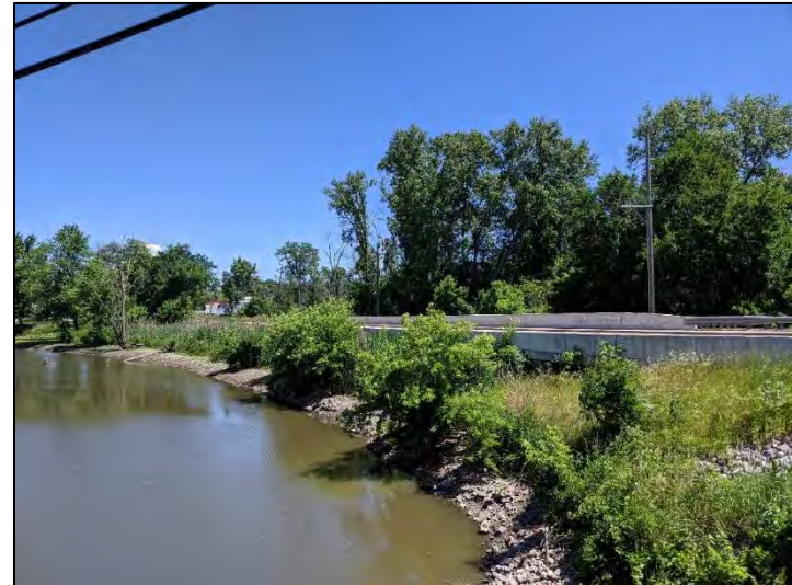
Photo 8. West side of bridge over Muck Pocket ((6)51-45-01943 B) and US 6 from covered bridge, viewing northeast, 6/14/2021
