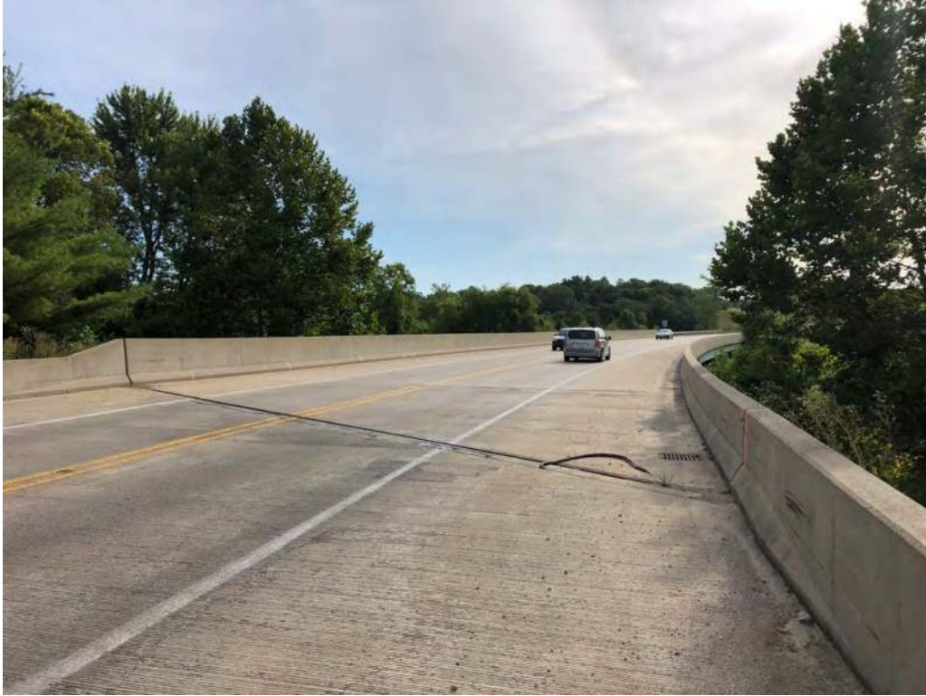
3. Facing east along SR 38 at Bridge over Wildcat Creek
