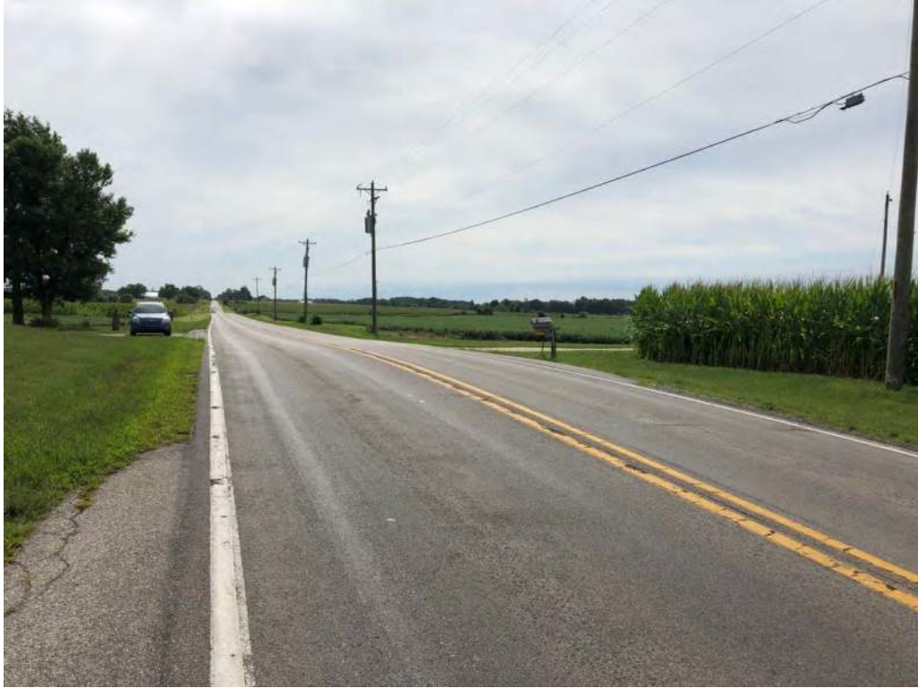
9. Facing west along SR 38 at 10230 SR 38
