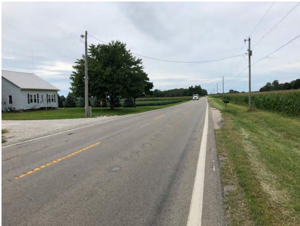
16. SR 38 looking west along alignment
