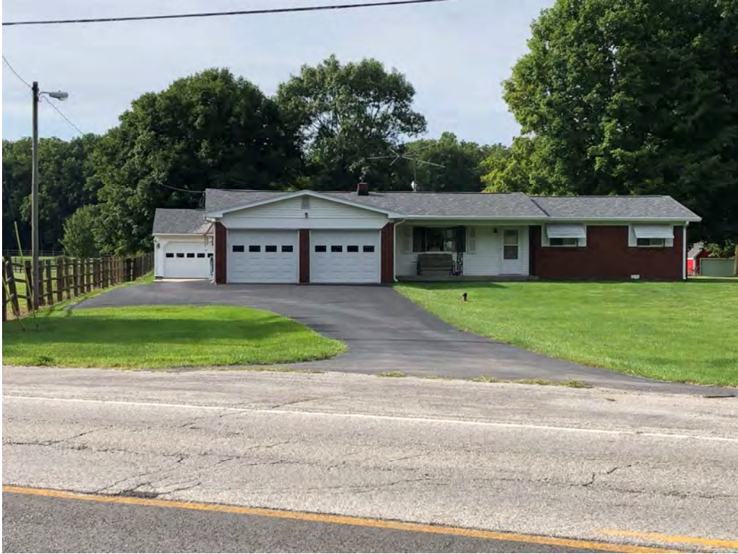
7. 8805 SR 38, a non-contributing property
