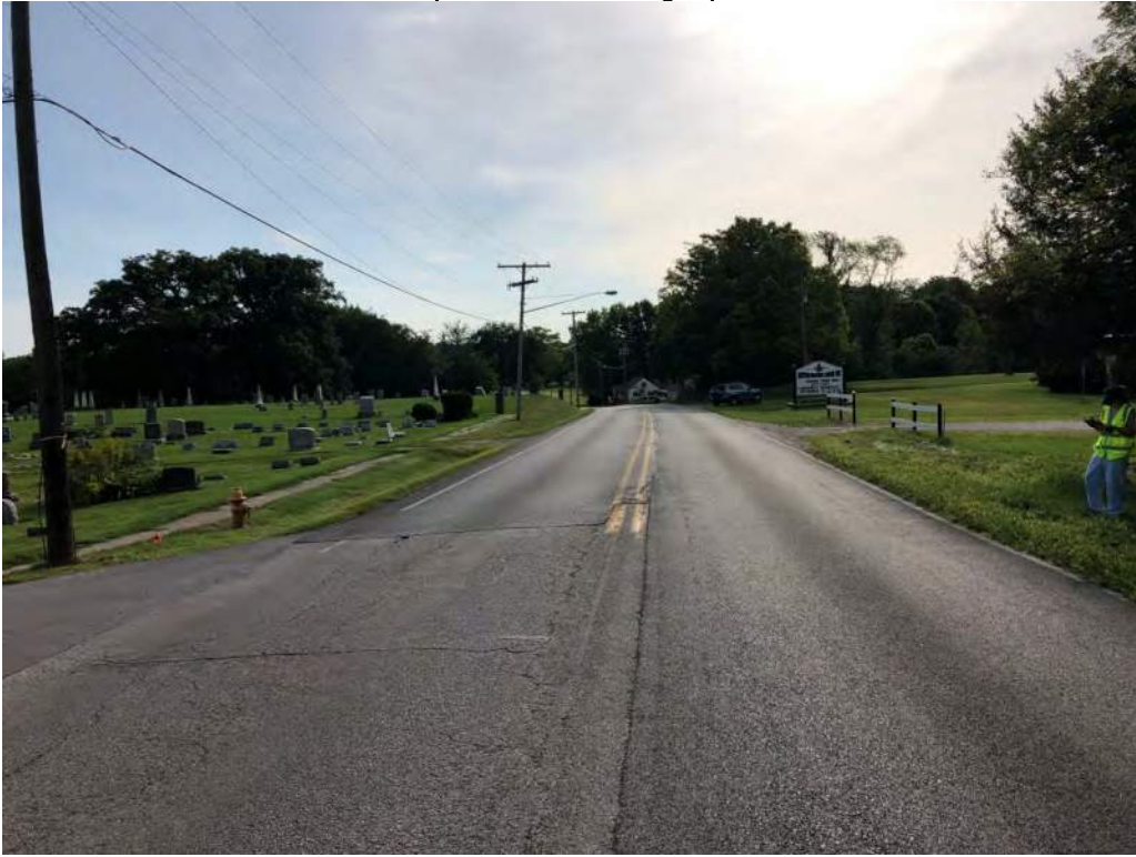
1. Facing east along SR 38 at Delaware St. at western end of APE
