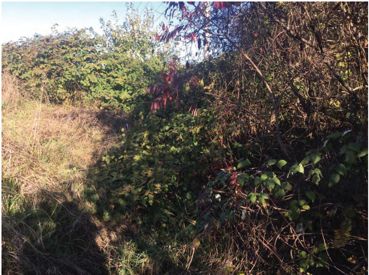
28. Looking north west down concrete side ditch
