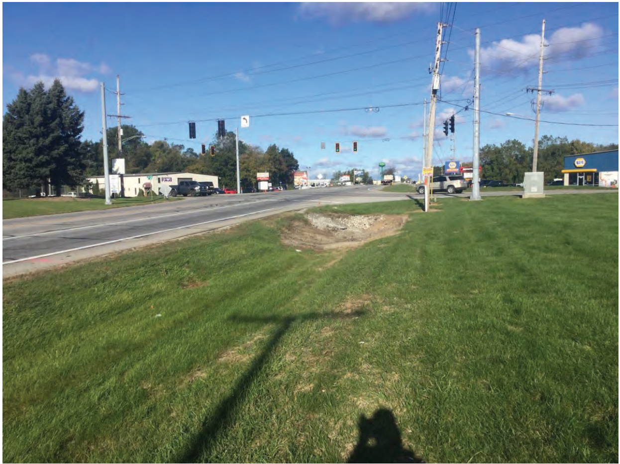
35. Looking north west at US 20 and SR 22
