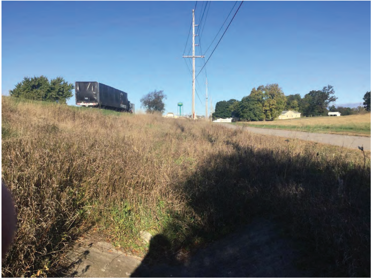
23. Looking north west along concrete side ditch
