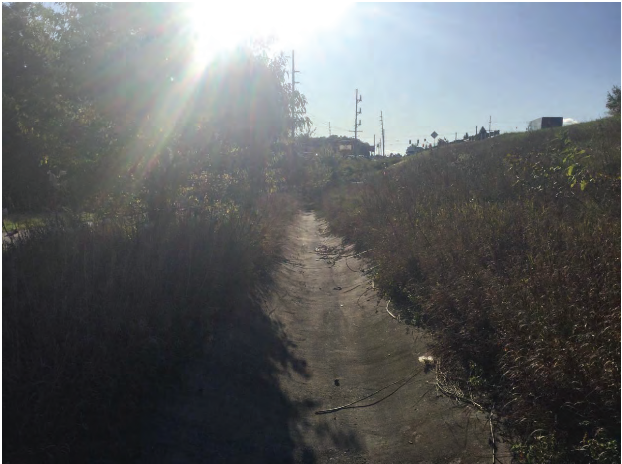
22. Looking south east down concrete side ditch
