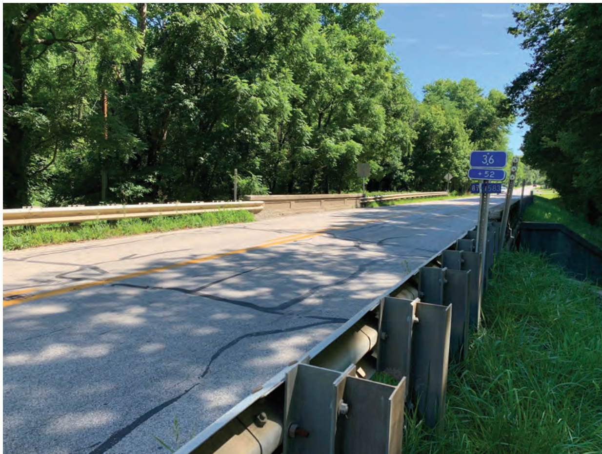
5. Looking northeast along SR 68 toward bridge
