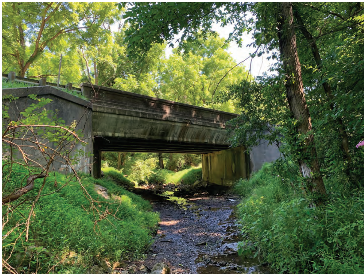
3. Looking upstream at Mill Creek facing northeast
