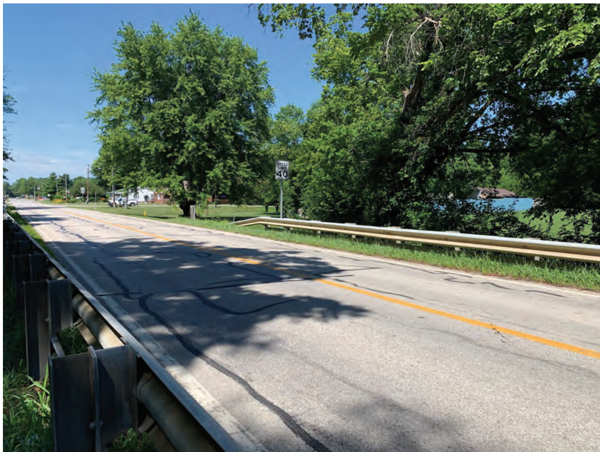
6. Looking west along SR 68 away from bridge
