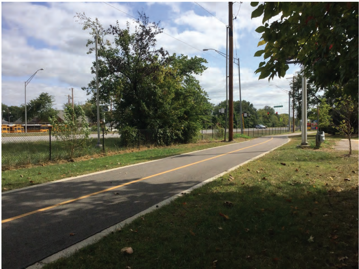
1. Looking southeast at the potential pedestrian crossing location from Blackford Avenue.
