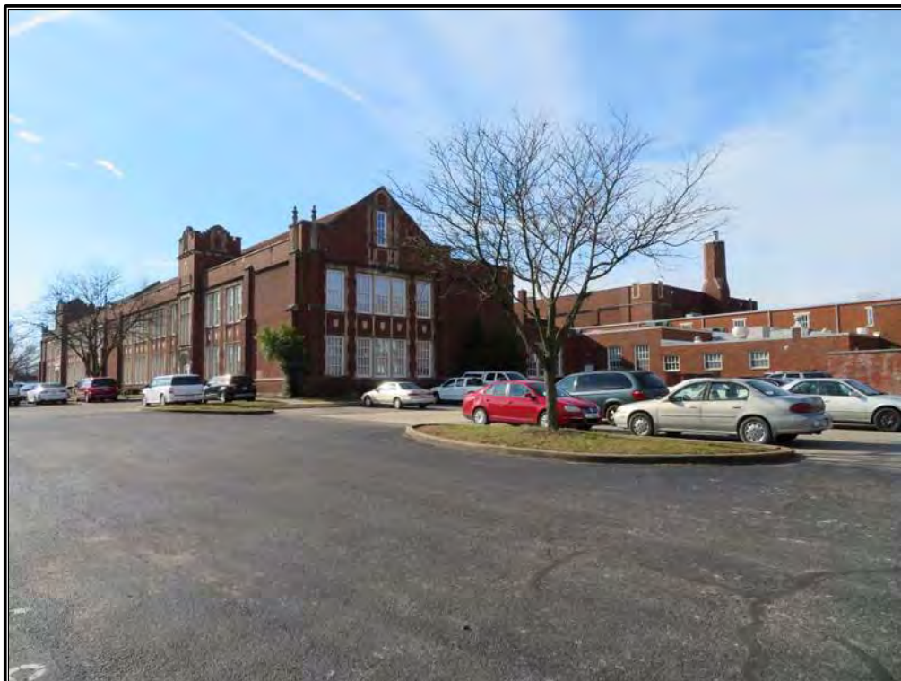
Figure B-13. Rear (north) and west elevation of Benjamin Bosse High School (IHSSI No. 163-196-41045), "Outstanding," located within a part of the Lincolnshire Historic District (NR-0908), facing southwest.
