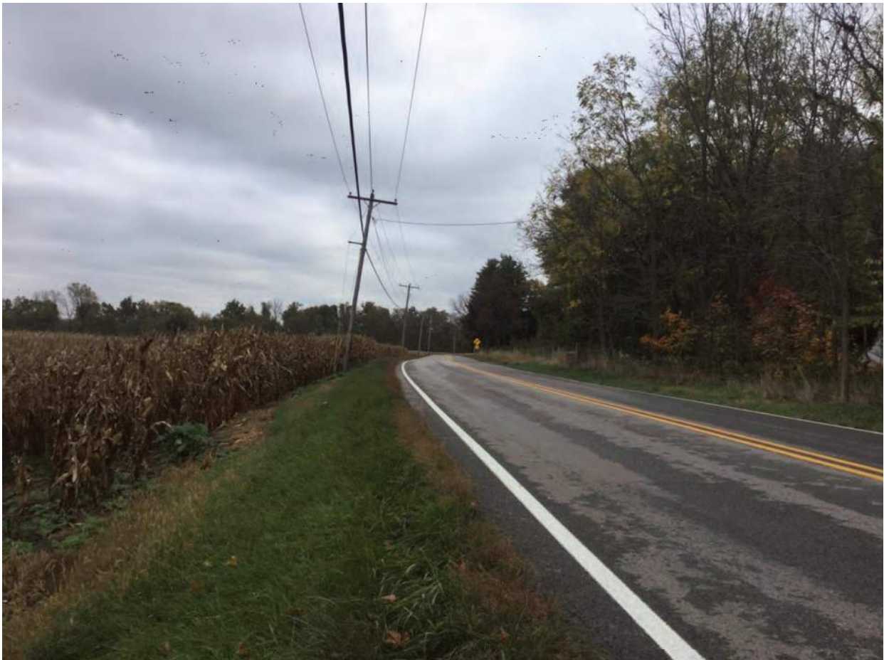
22. Looking northeast along SR 124 along roadside ditch on north side of road
