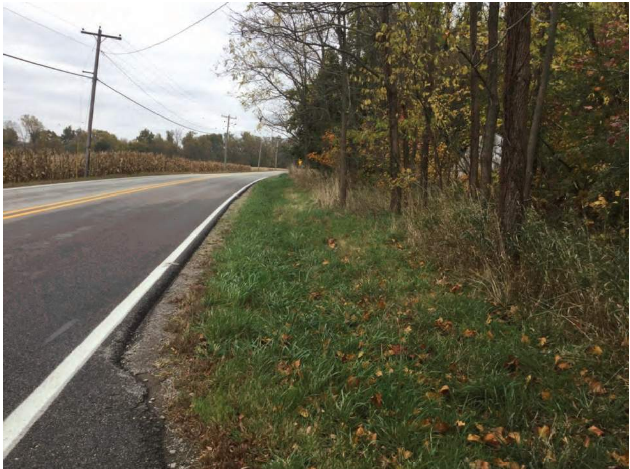
24. Looking northeast along south side of SR 124 at roadside drainage from driveway Des No 1800552 Appendix B, Page 34 of 101
