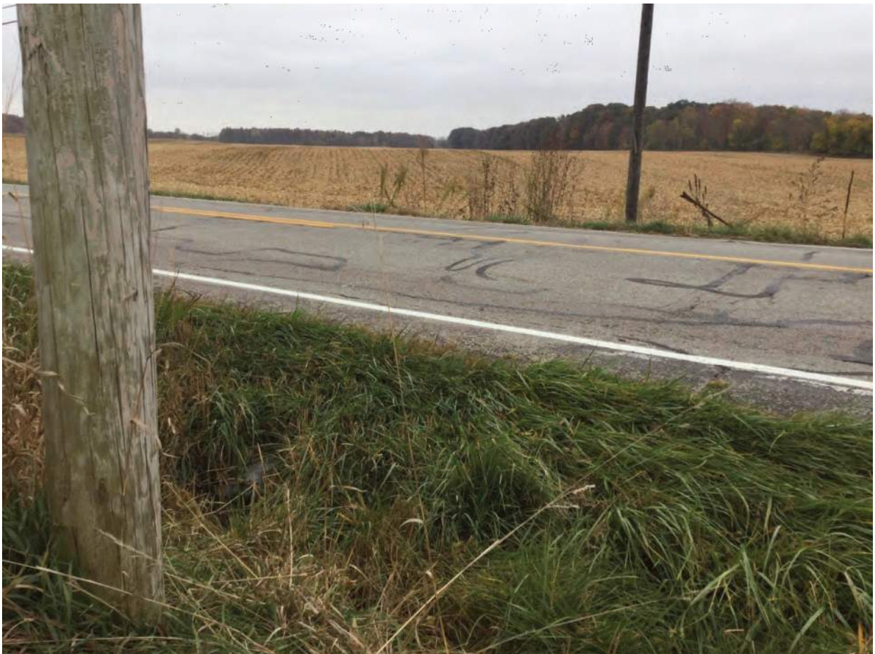
74. Looking south at culvert under SR 124
