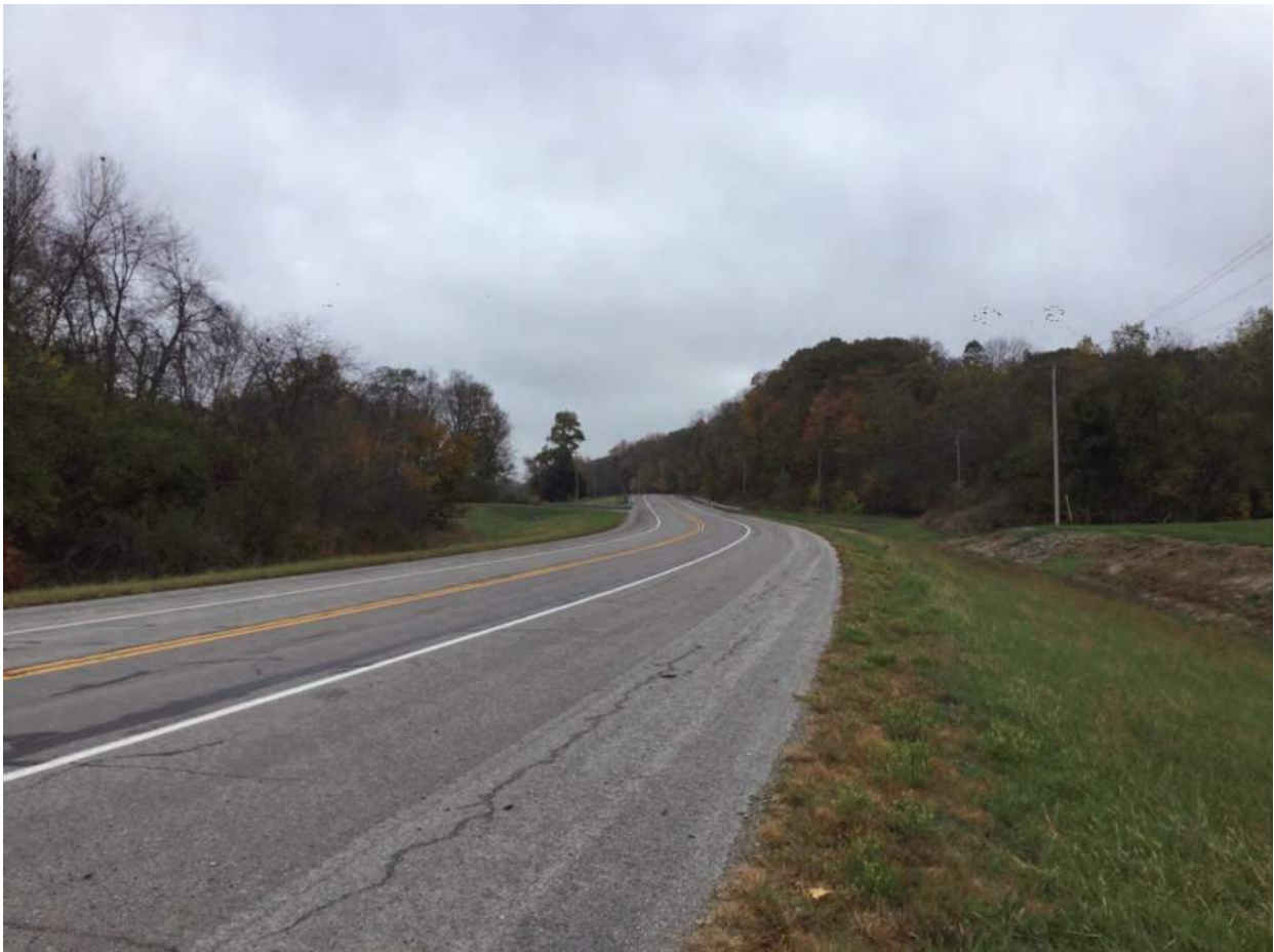
20. Looking east along SR 124 towards bridge
