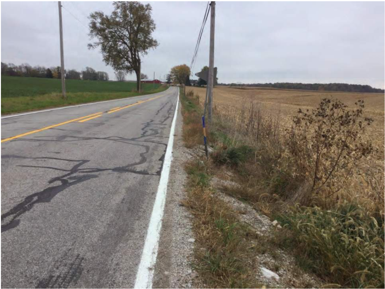
69. Looking southeast along SR 124 to culvert COID 19871, located at shovel
