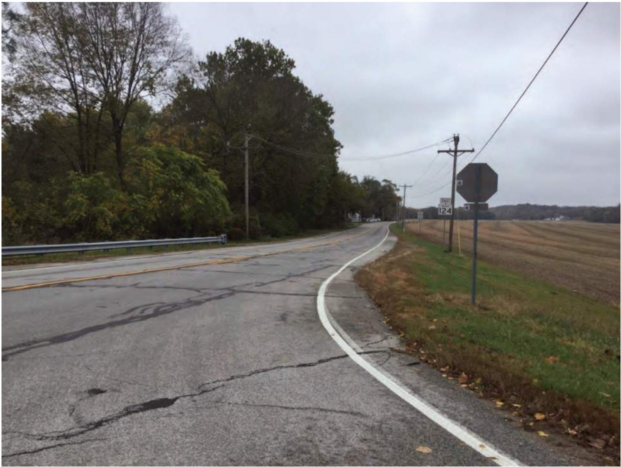
17. Looking east along SR 124 from Wallace Avenue intersection
