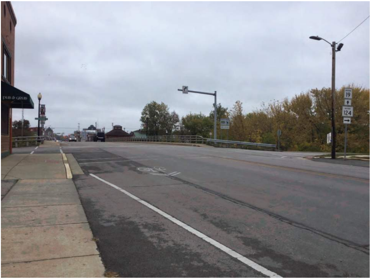
5. Looking northwest to SR 19 bridge over Mississinewa River
