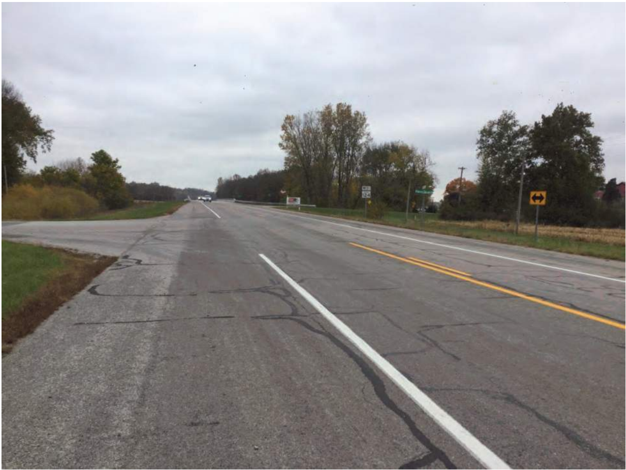
67. Looking northwest towards intersection with Francis Slocum Trail
