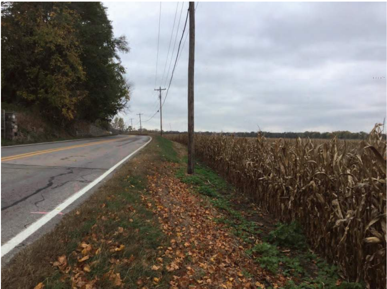
36. Looking southwest along SR 124 on north roadside
