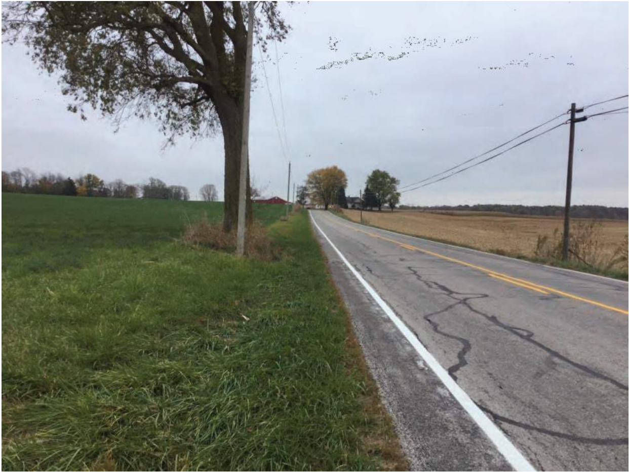
75. Looking southeast along SR 124 towards culvert
