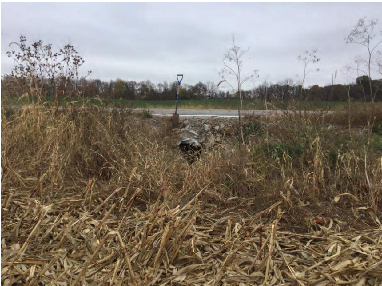
70. Looking northeast to culvert COID 19871 under SR 124
