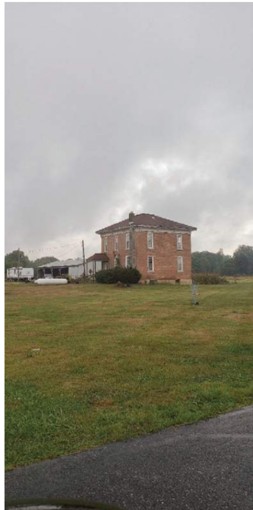
D. Looking northwest to 2 story brick Italianate residential structure
