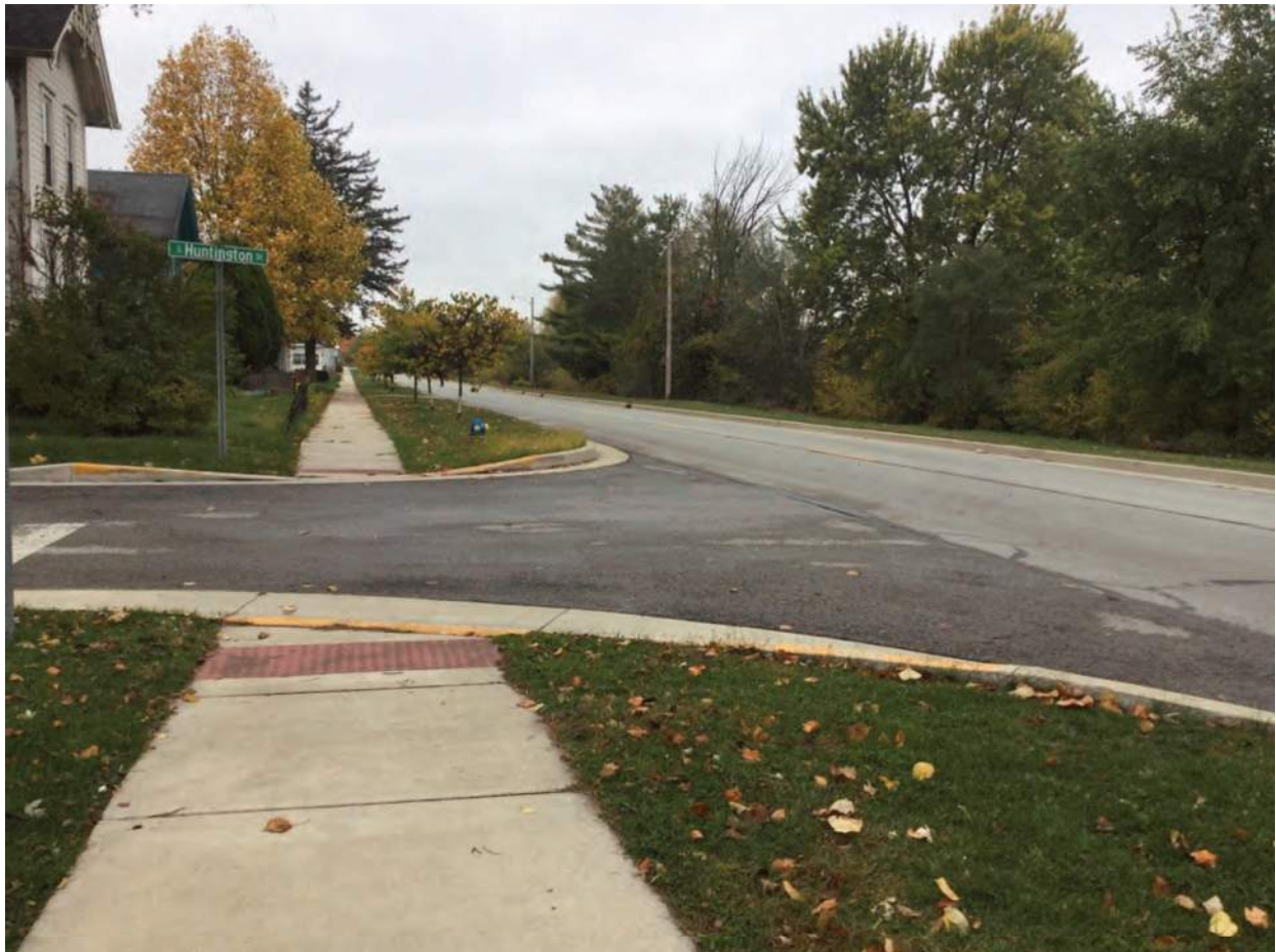
8. Looking southwest along SR 124 from Huntington Street
