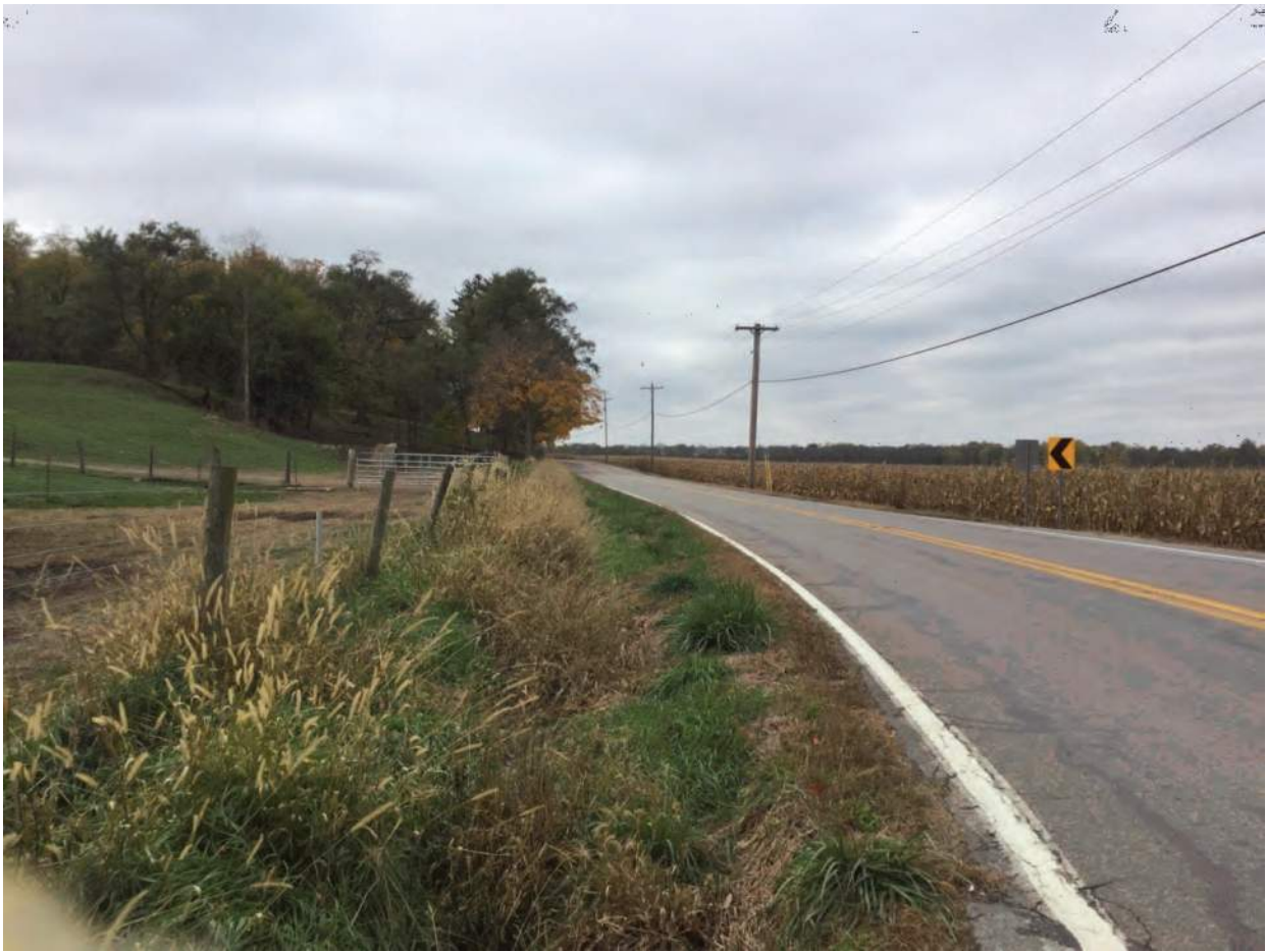
39. Looking southwest along UNT 1 to Mississinewa river and SR 124 from culvert under SR 124
