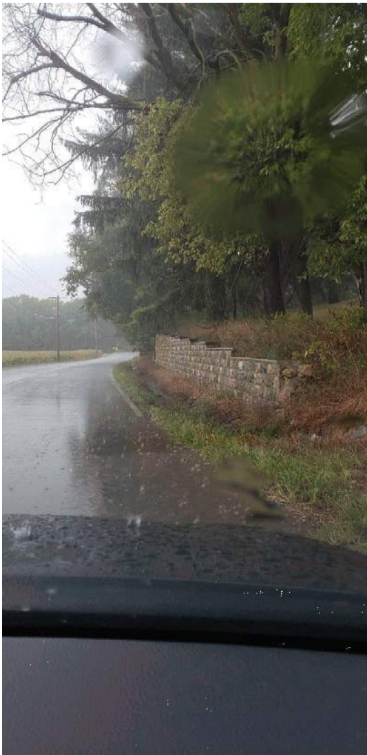
A. Looking northeast at stone retaining wall on SR 124
