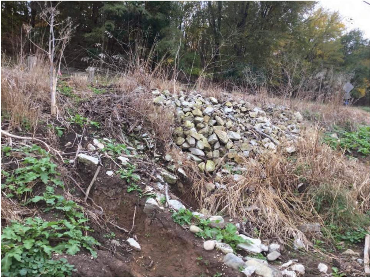
31. Looking southwest to riprap stabilization
