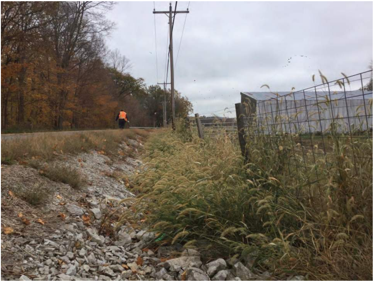
41. Looking southeast along riprap roadside ditch
