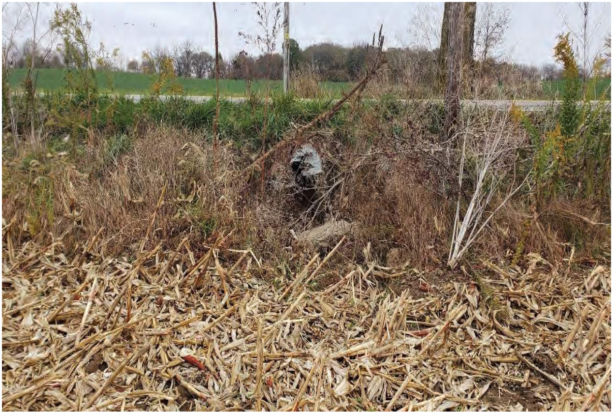
73. Looking north at downstream end of culvert under SR 124
