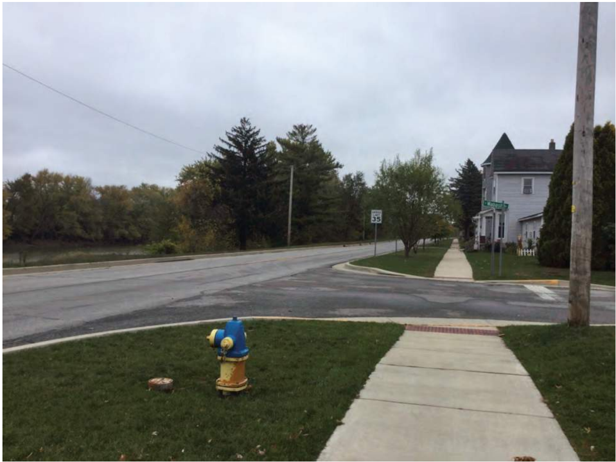
7. Looking northeast along SR 124 from intersection with Wabash Street
