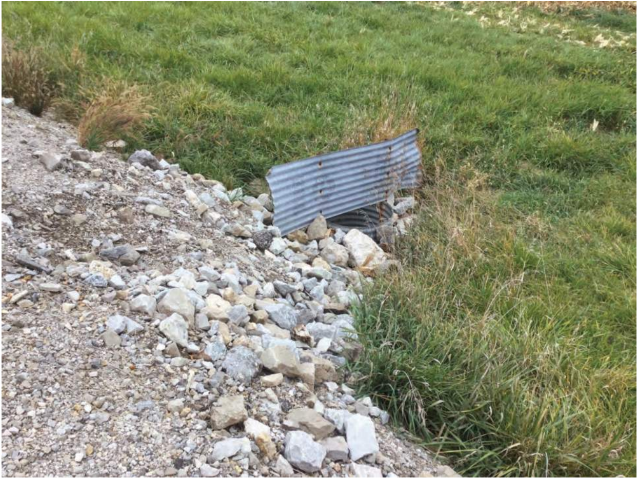
83. Looking south to culvert COID 19871
