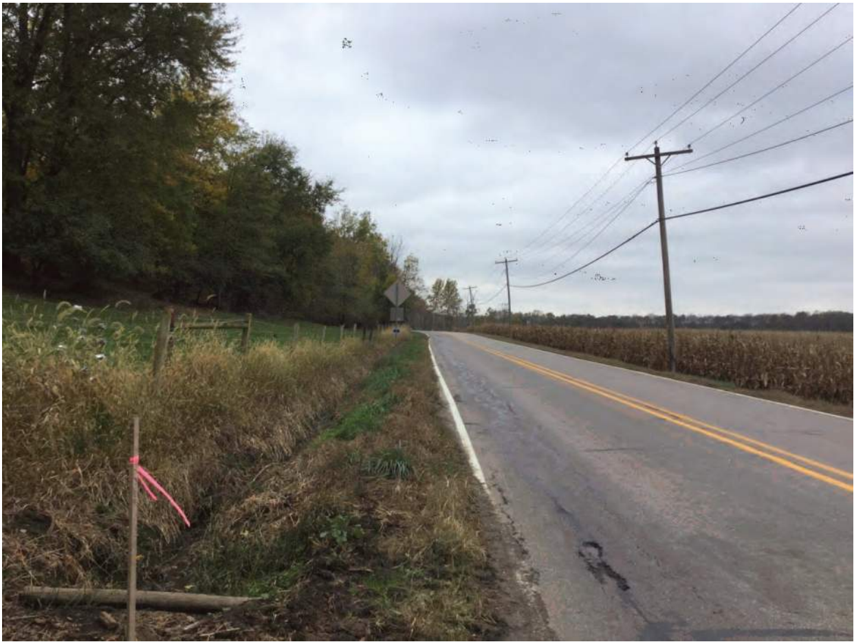
29. Looking southwest along SR 124 and UNT 1 to Mississinewa River from south side
