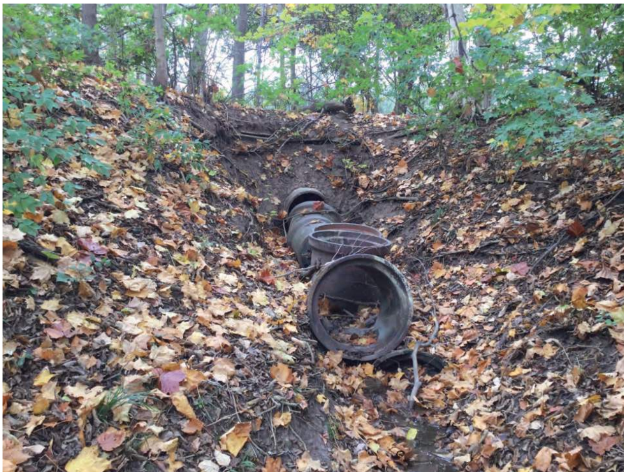
50. Looking south to culvert draining UNT 1 to Mississinewa River
