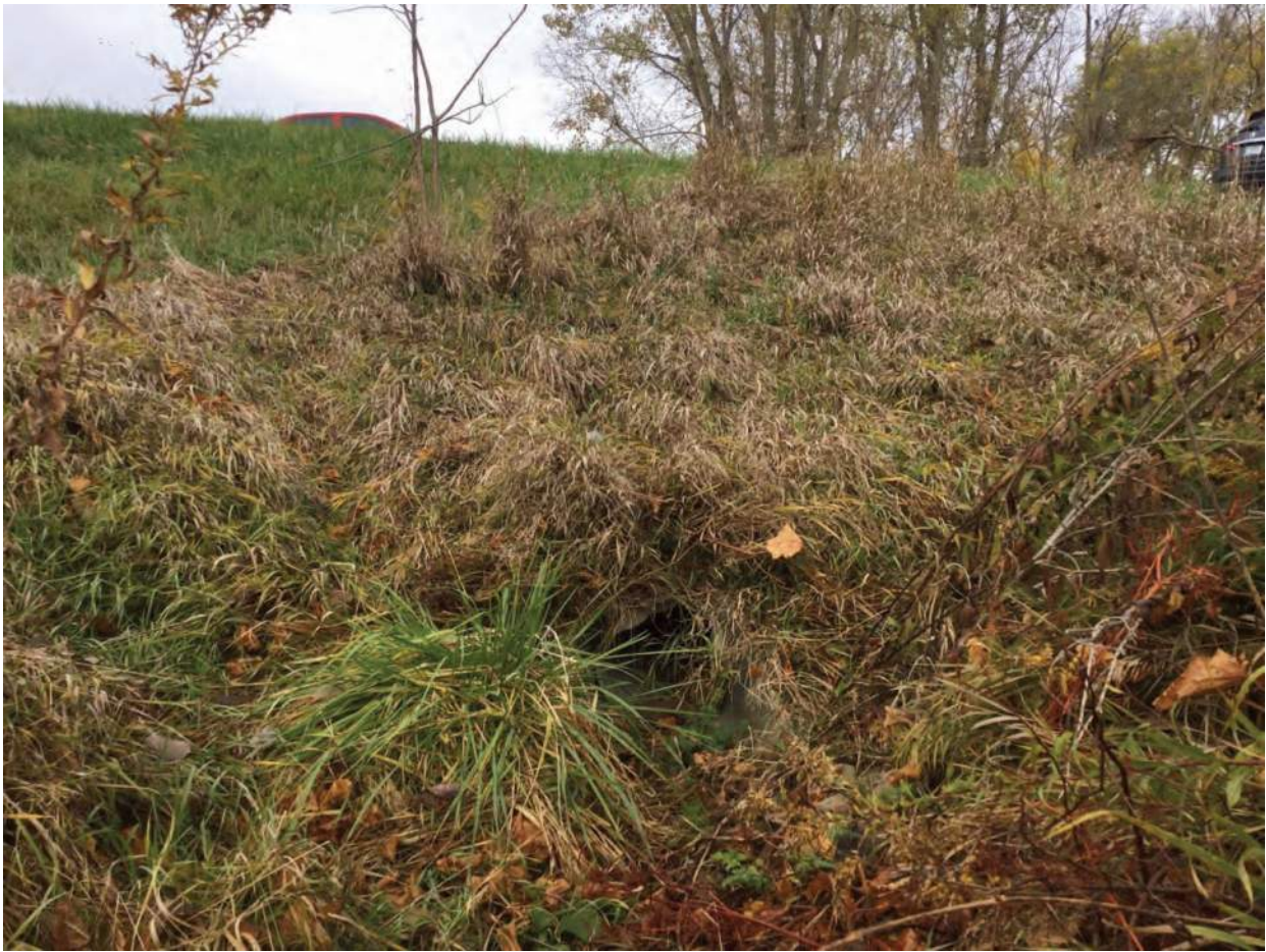
55. Looking northwest towards culvert COID 19925, conveying RSD 1 under Circus Lane
