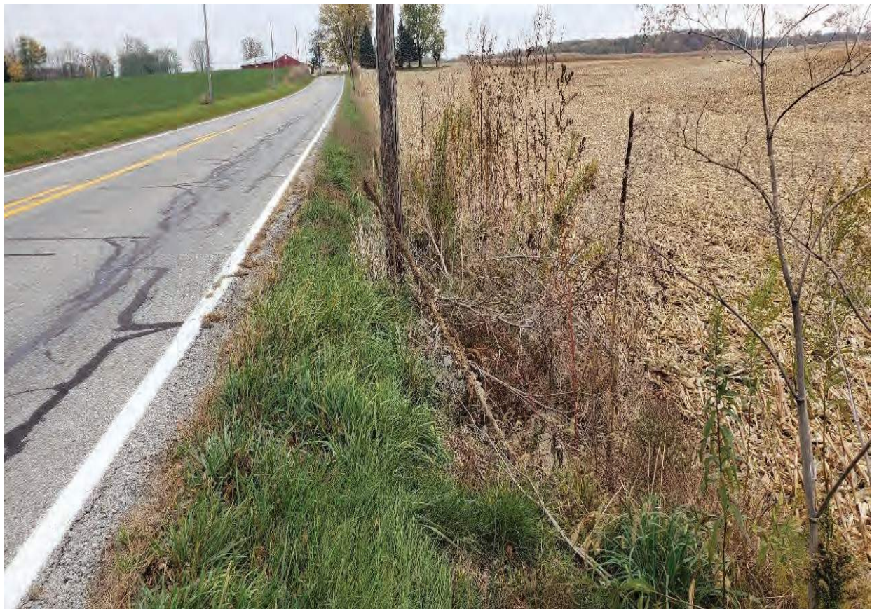
72. Looking southeast along SR 124 at culvert
