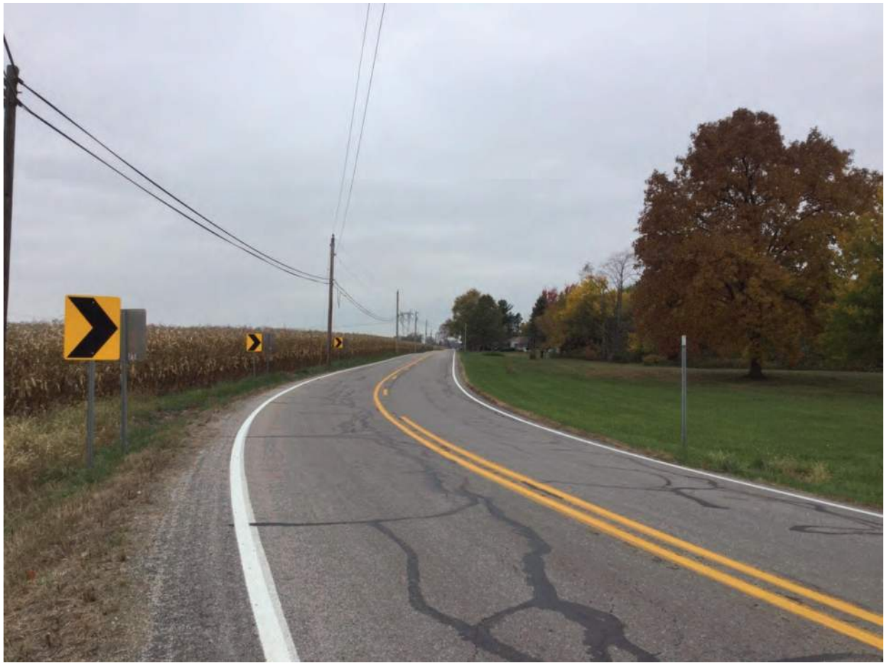
79. Looking northwest along SR 124 from 550 East
