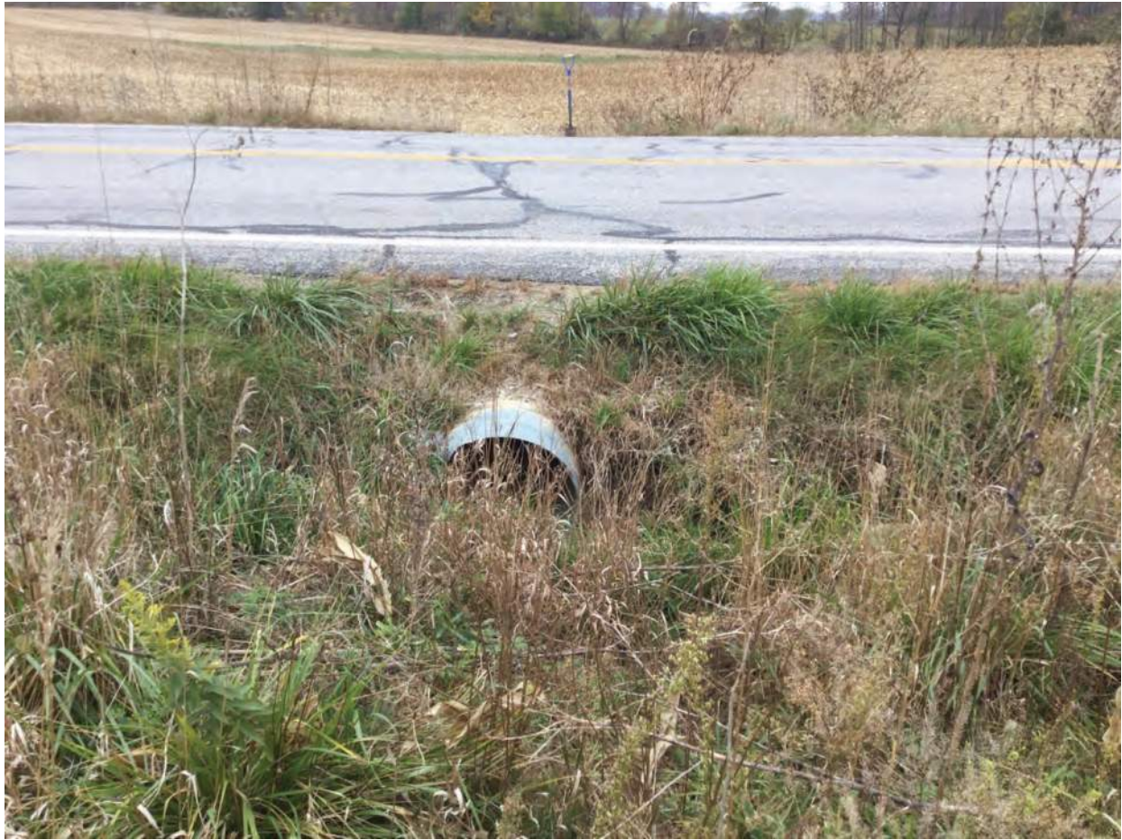
71. Looking southwest to culvert COID 19871 under SR 124
