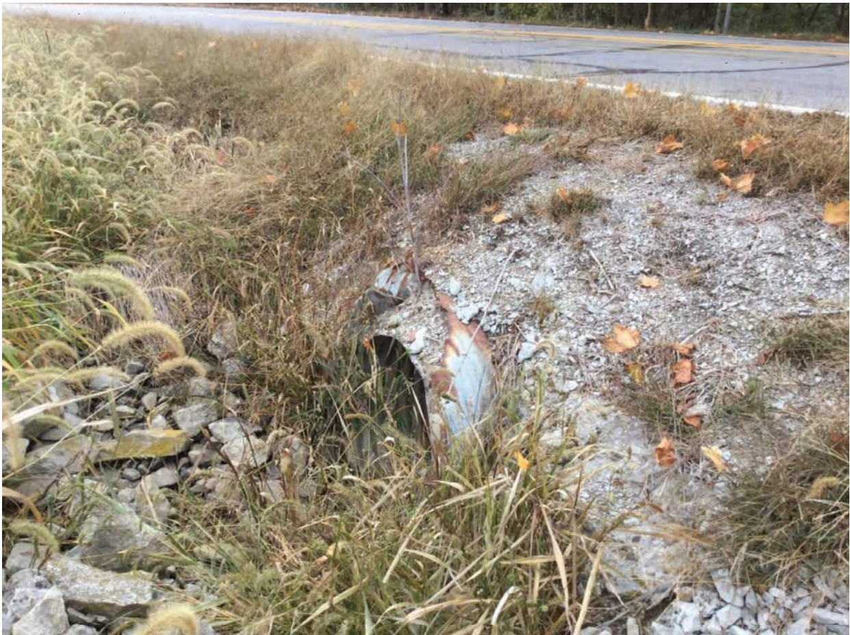
40. Looking northwest to culvert draining UNT 1 to Mississinewa River under SR 124
