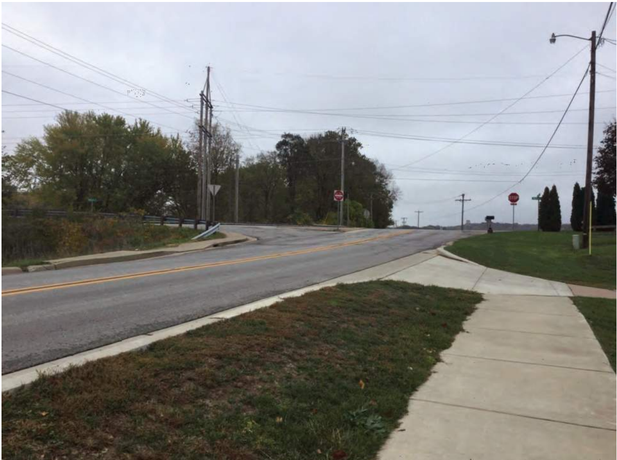
12. Looking east towards SR 124 intersection with Wallace Avenue
