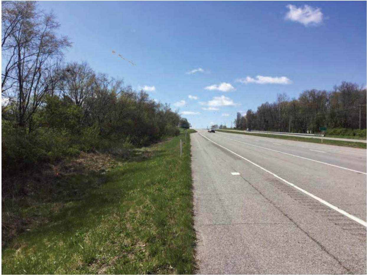
9. Looking south along US 41
