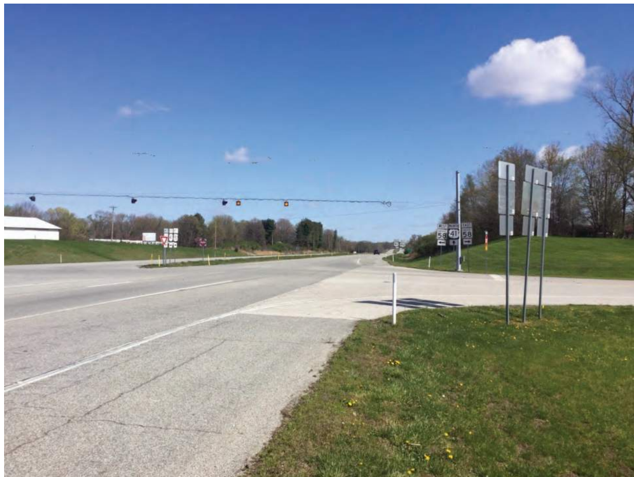
6. Looking north at US 41 & SR 58 intersection
