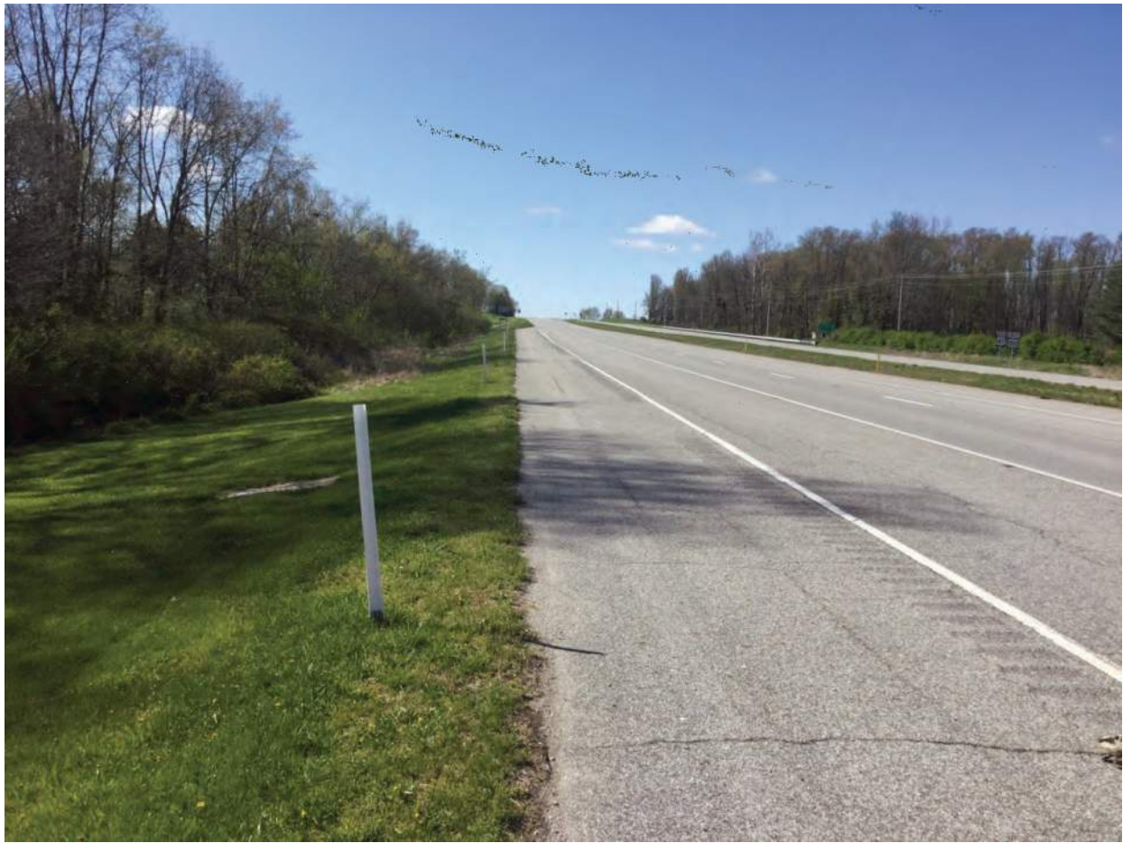
1. Looking south along northbound US 41
