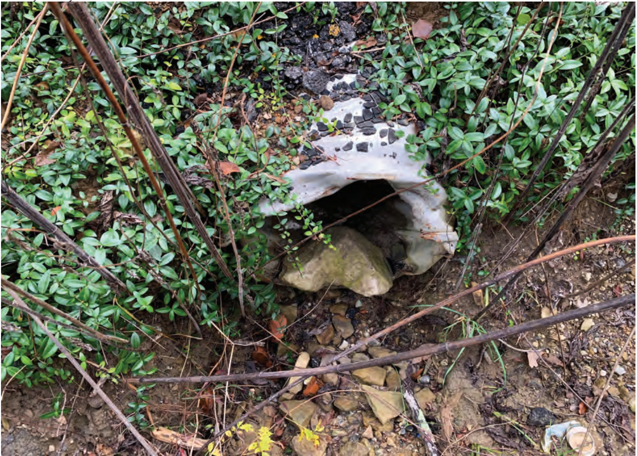
3. View of culvert outlet under SR 145 facing southeast
