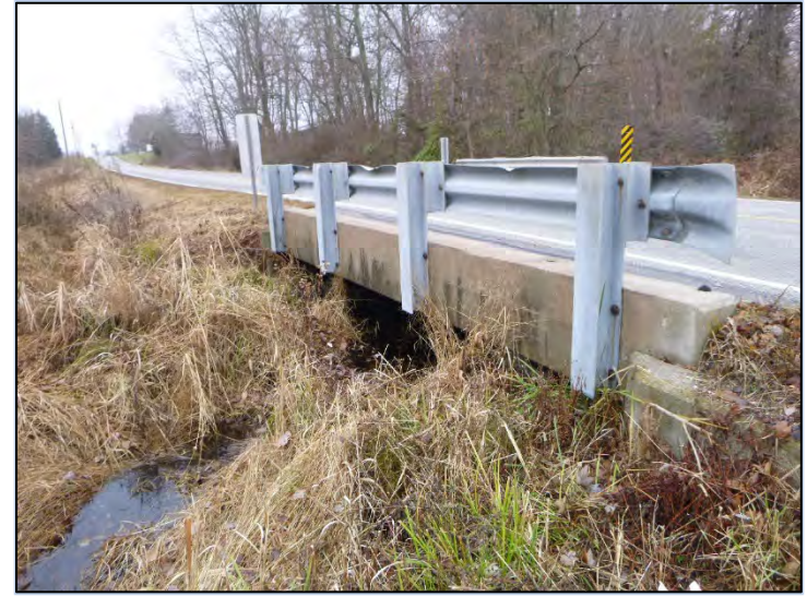
Photo 2: Existing structure on SR 250 over UNT to Rider Ditch.
