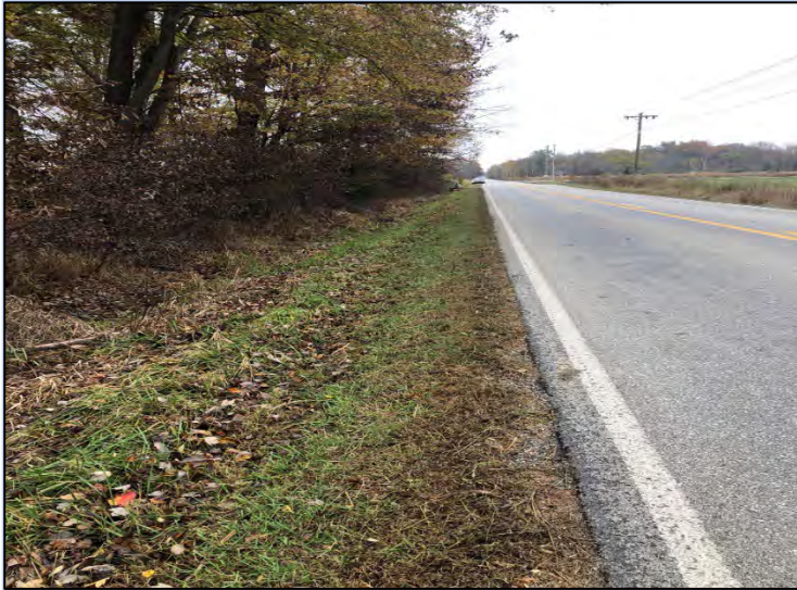
Photo 3: Looking east on the north side of SR 250.
