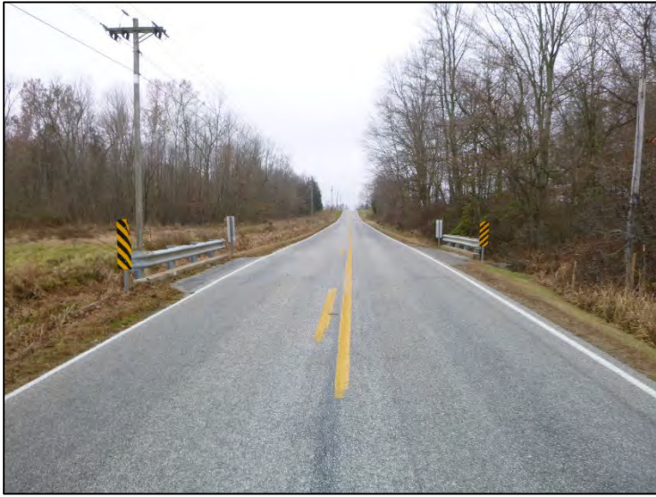
Photo 1: Looking west on SR 250 at the existing structure.
