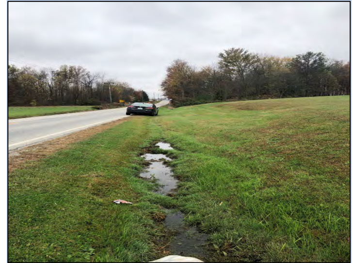
Photo 8: Looking west at north roadside of SR 250.
