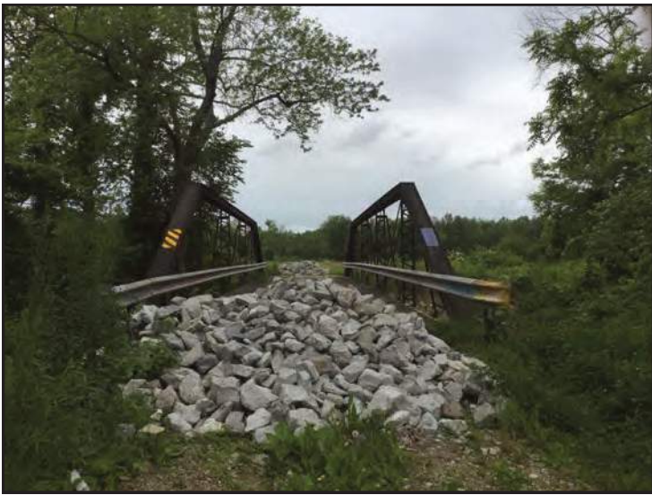
1. View looking west at Jackson County Bridge No. 154
