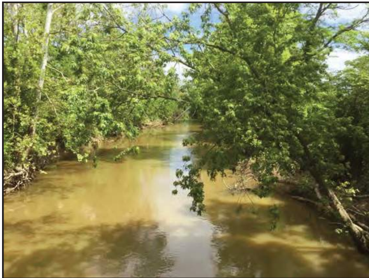
7. View of Rider Ditch looking north (upstream)
