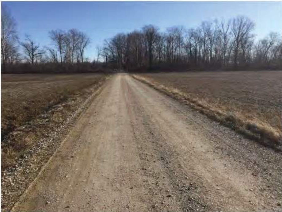
Photo 10. CR 300 South, camera facing east toward Jackson County Bridge 154.
