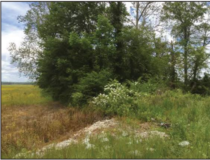
5. View of the northwest quadrant of the Jackson County Bridge No. 154 crossing
