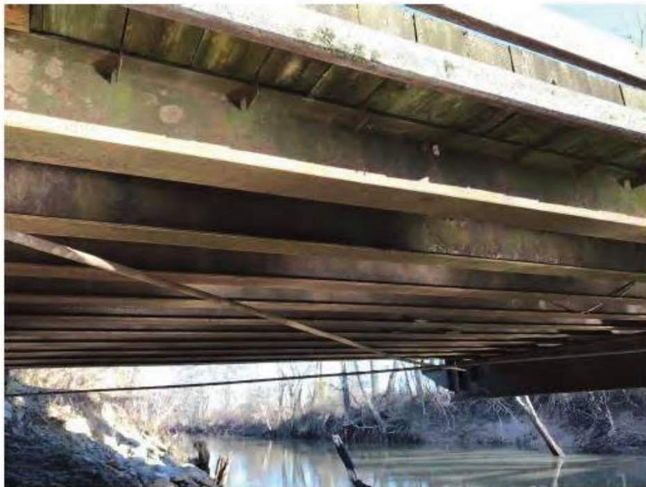
Photo 8. Detail of Jackson County Bridge 154.
