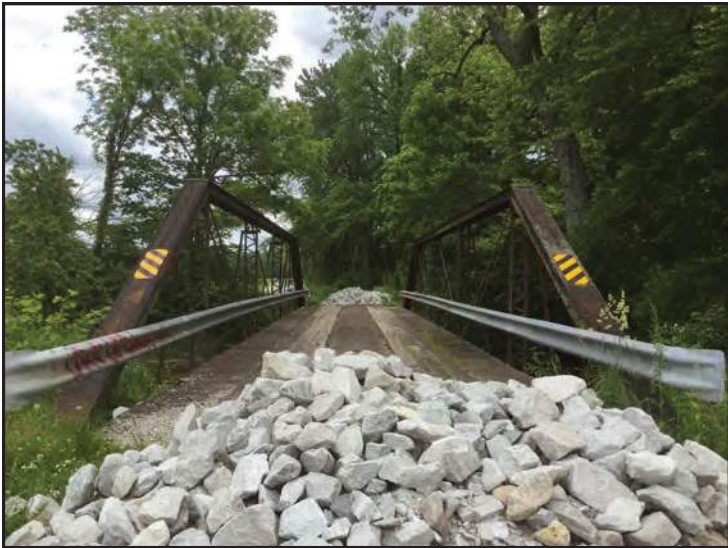
3. View looking east at Jackson County Bridge No. 154
