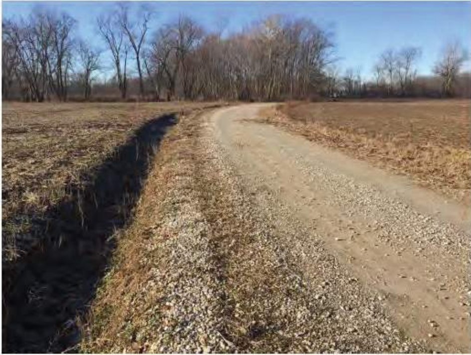
Photo 1. CR 300 South, camera facing west towards Jackson County Bridge 154.
