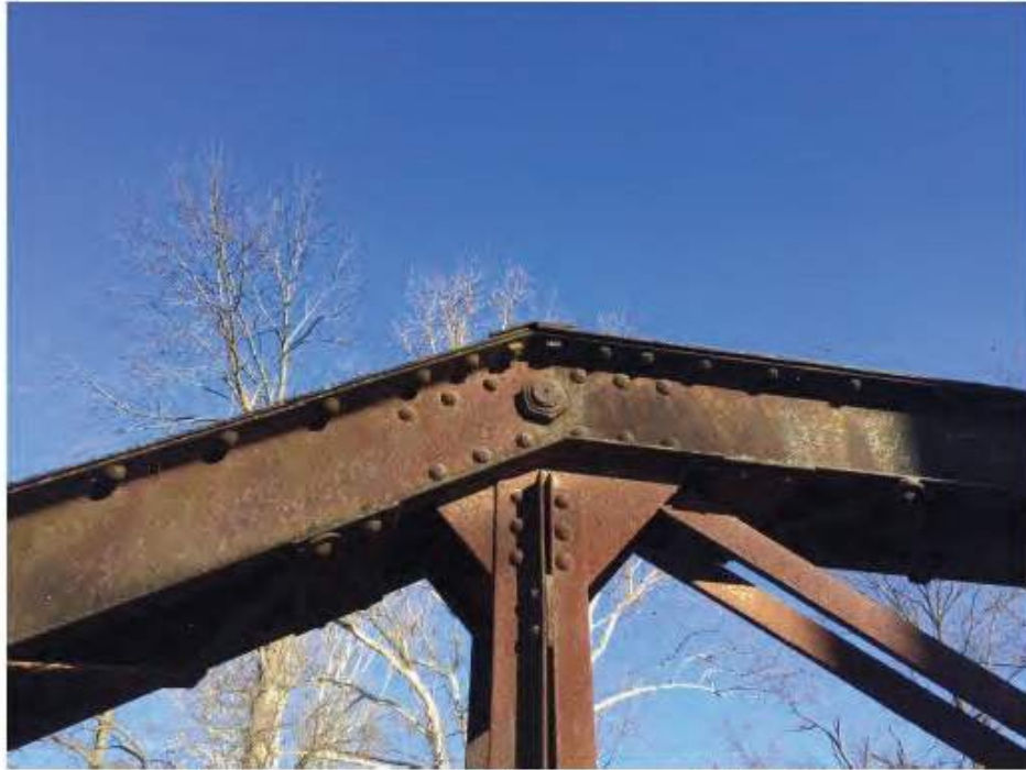
Photo 7. Detail of Jackson County Bridge 154.
