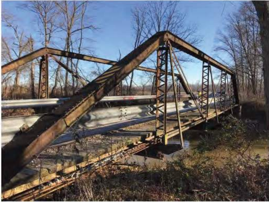
Photo 3. Jackson County Bridge 154, camera facing northeast.
