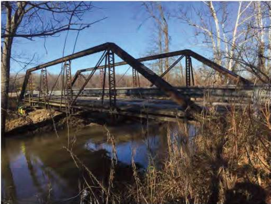
Photo 2. Jackson County Bridge 154, camera facing northwest.
