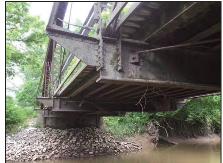
8. View of east embankment of Jackson County Bridge No. 154
