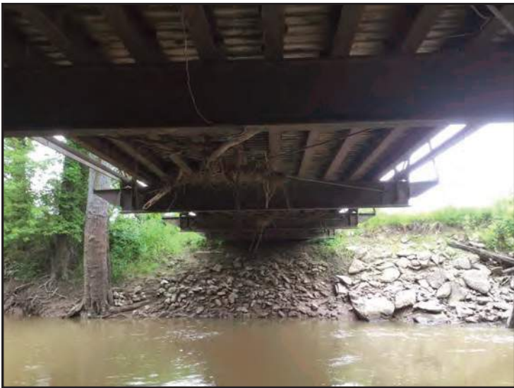
9. View of west embankment of Jackson County Bridge No. 154
