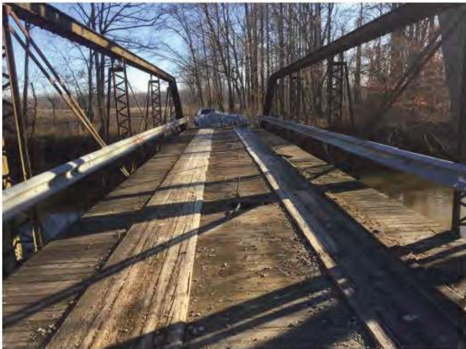
Photo 4. Jackson County Bridge 154, camera facing east.
