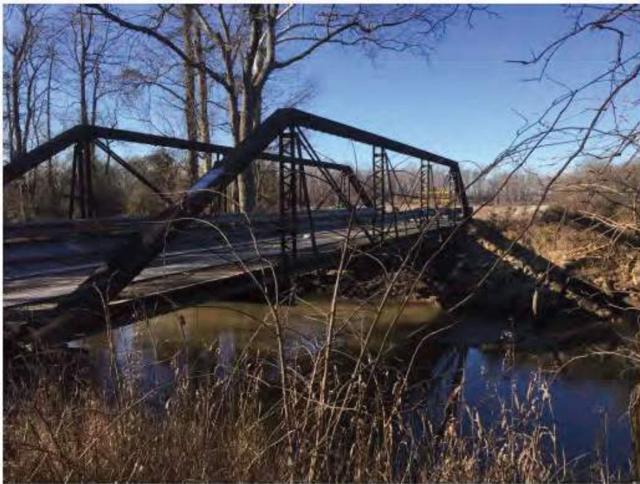
Photo 6. Jackson County Bridge 154, camera facing southwest.
