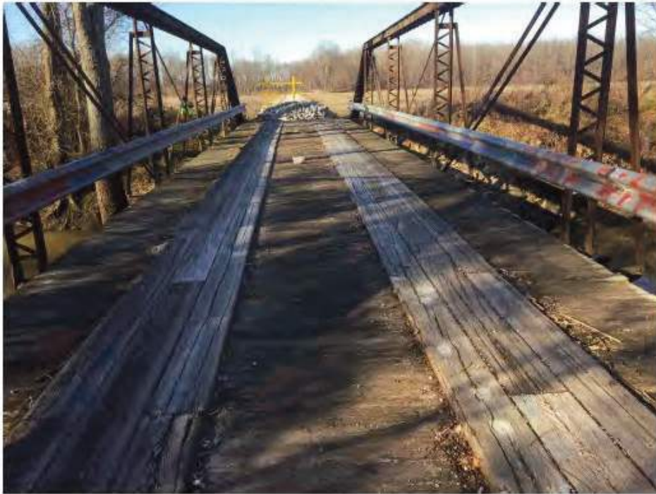
Photo 5. Jackson County Bridge 154, camera facing west.
