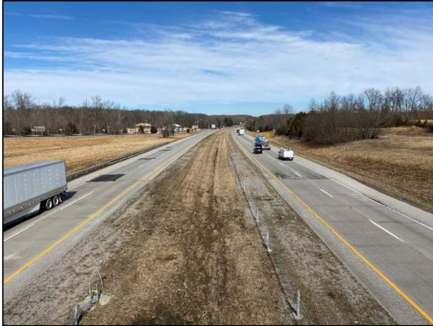
Photo 5: Looking north on I-65 from SR 160 Henryville interchange overpass.
