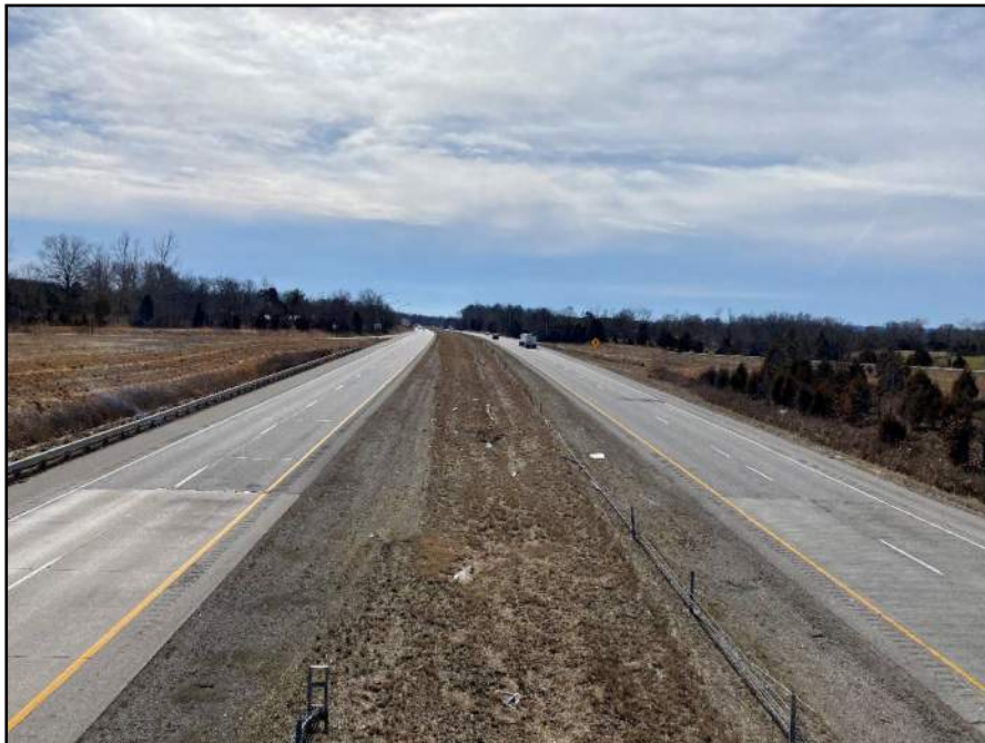
Photo 4: Looking south on I-65 from SR 160 Henryville interchange overpass.
