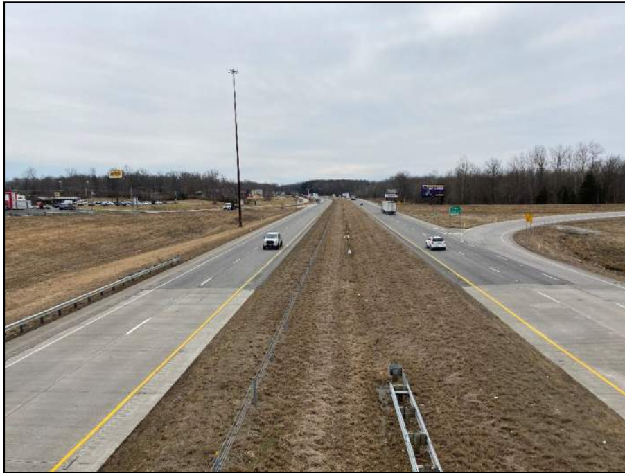
Photo 15: Looking south on I-65 from SR 56 Interchange overpass.
