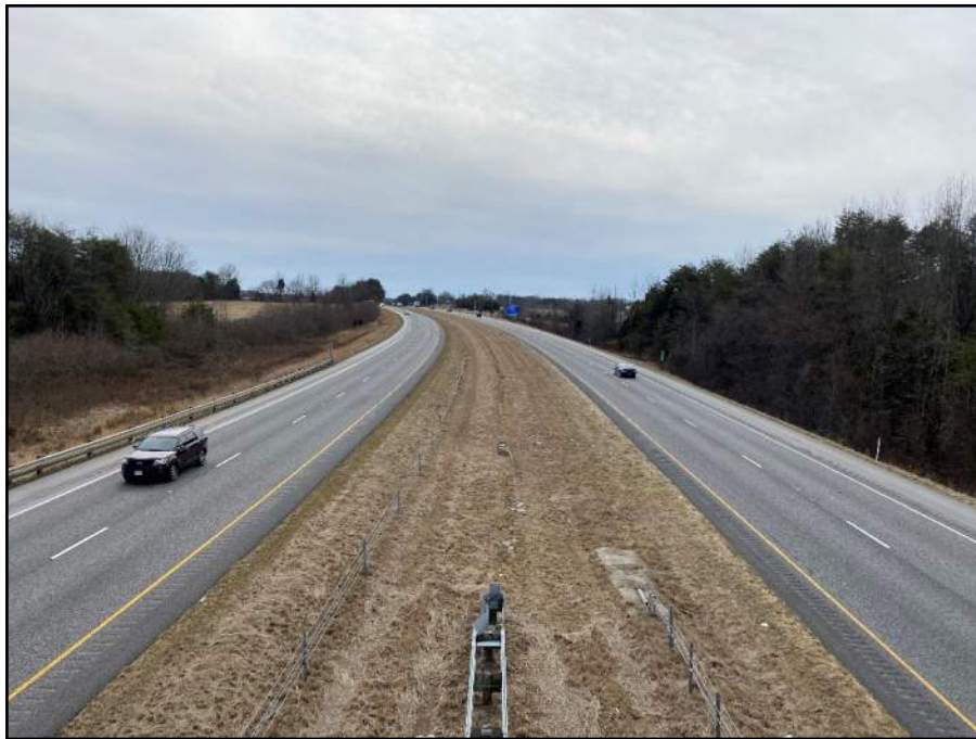
Photo 8: Looking south on I-65 from East County Line Road overpass.
