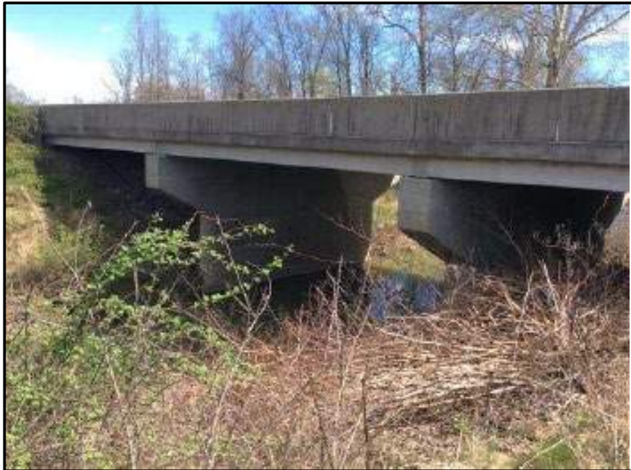
Photo 18: I-65 Bridges over Pigeon Roost Creek.
