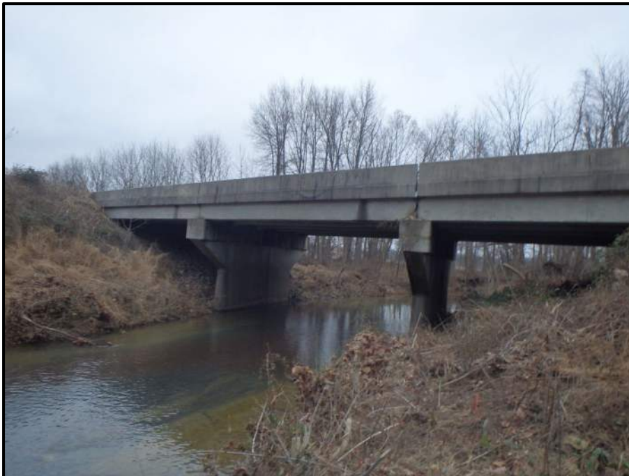
Photo 16: I-65 Bridges over Blue Lick Creek.
