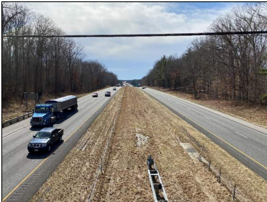
Photo 6: Looking south on I-65 from Winding Road overpass.
