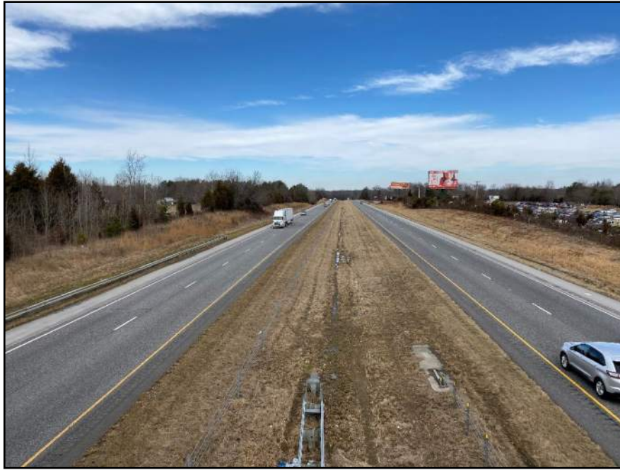
Photo 9: Looking north on I-65 from East County Line Road overpass.
