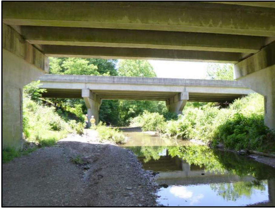
Photo 17: I-65 Bridges over Caney Fork.
