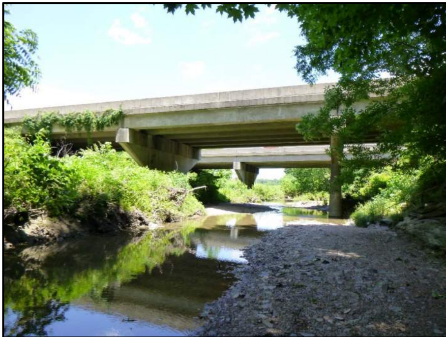
Photo 18: I-65 Bridges over Caney Fork.
