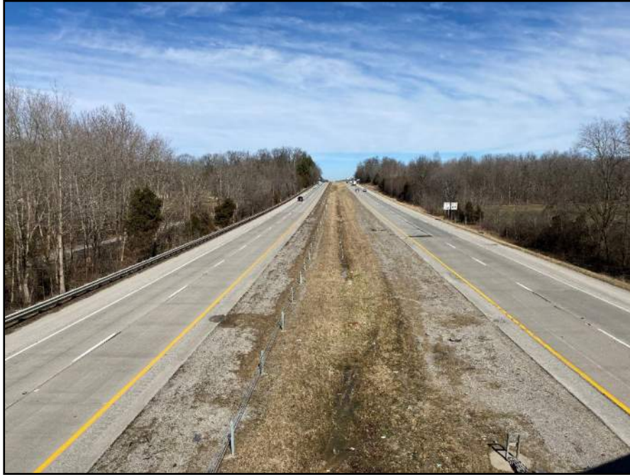
Photo 3: Looking north on I-65 towards Memphis Road from Biggs Road overpass.
