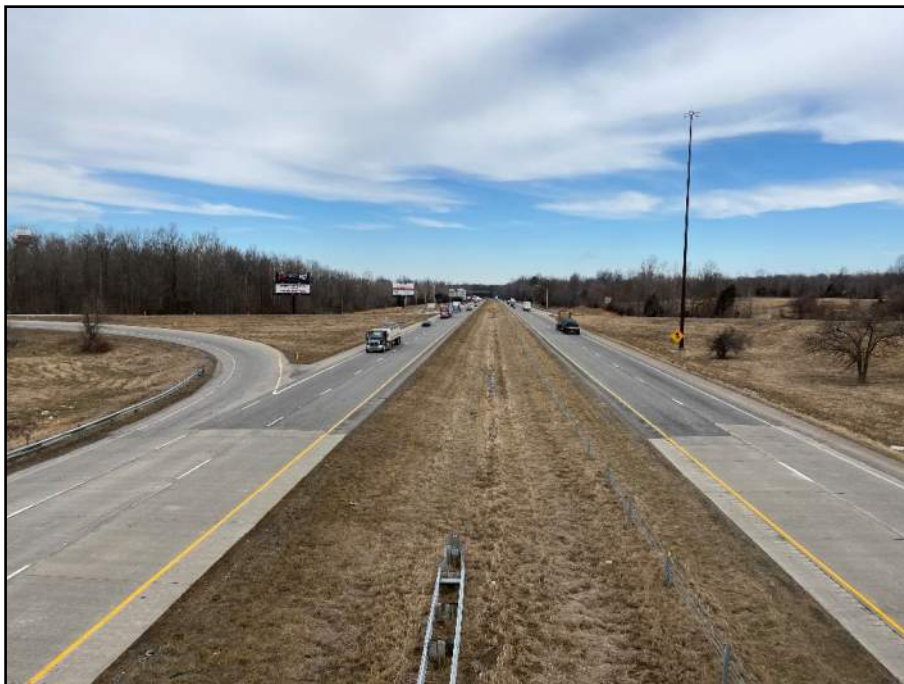
Photo 14: Looking north on I-65 from SR 56 Interchange overpass.
