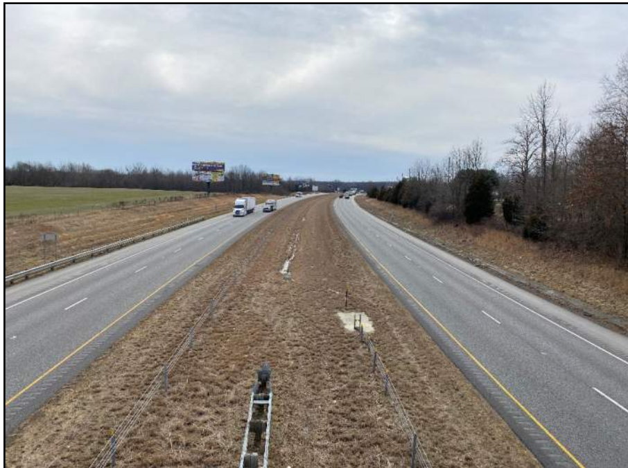
Photo 12: Looking south on I-65 from West Lake Road/ Lovers Lane overpass.
