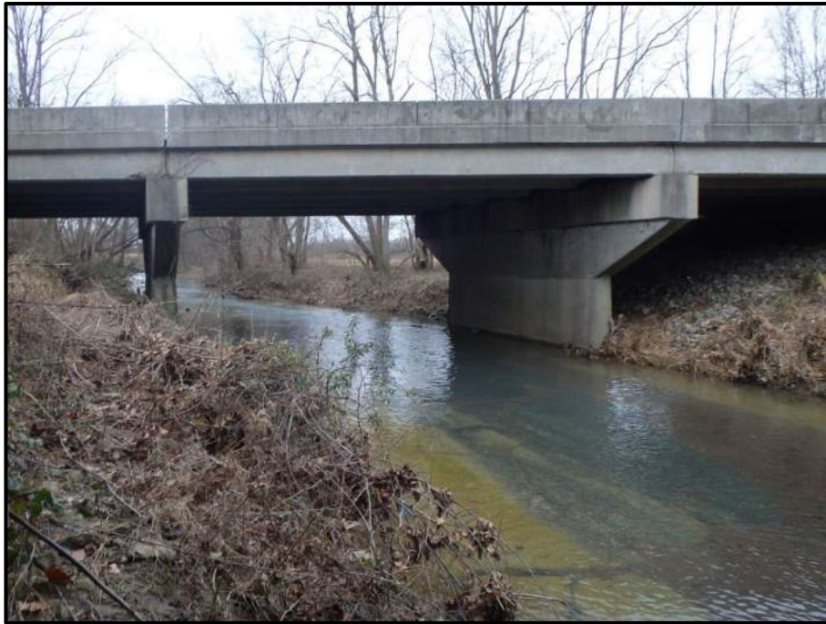
Photo 17: I-65 Bridges over Blue Lick Creek
