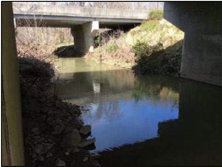
Photo 17: I-65 Bridges over Pigeon Roost Creek.
