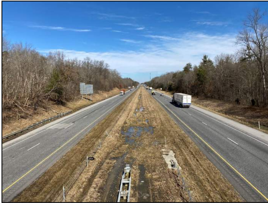
Photo 7: Looking north on I-65 from Winding Road overpass.
