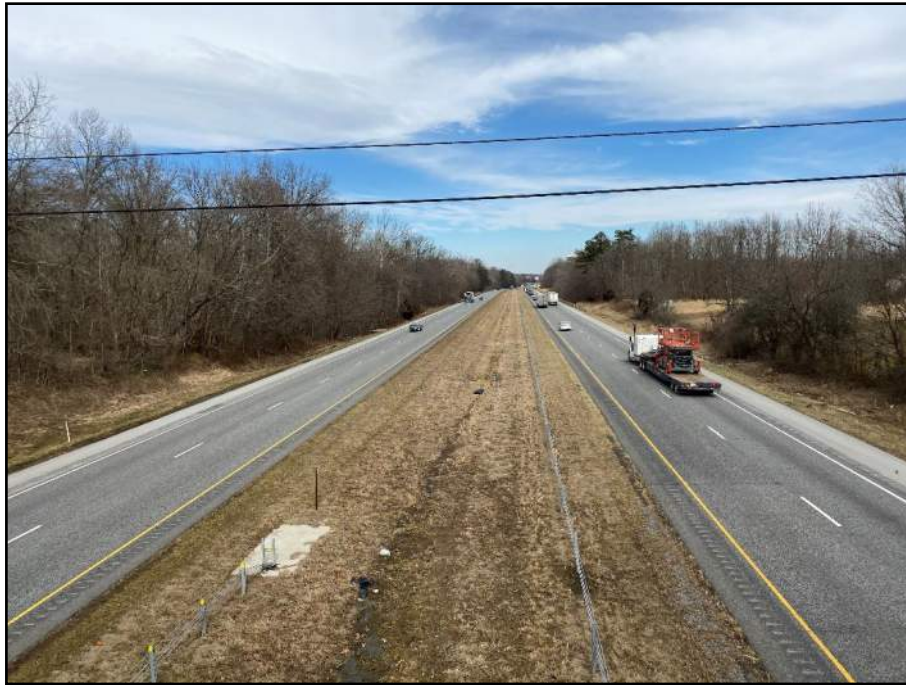
Photo 11: Looking north on I-65 from County Road 300 S overpass.
