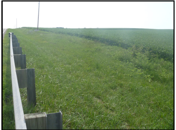
Photo 40 – Southeast Quadrant: Facing southeast from the southeast quadrant of the project location. Roadside ditch is a vegetated, poorly defined swale.
