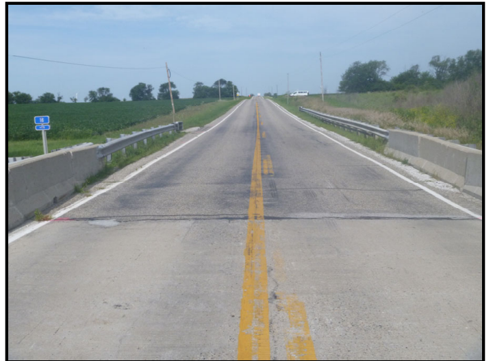
Photo 22 – SR 18 Crossing: Facing west along SR 18 from the top of the bridge over Greenwood Ditch. Topography is generally flat to rolling. Creek and bridge sit in a shallow depression of the landscape.
