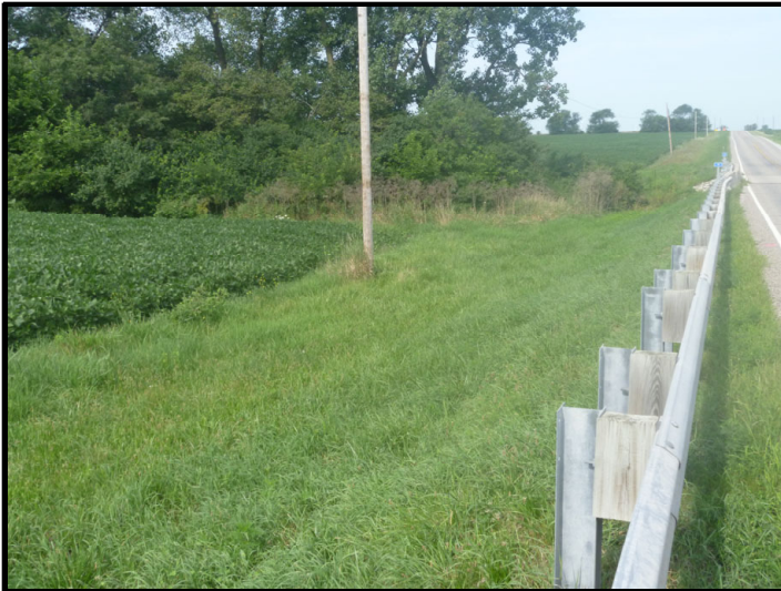
Photo 39 – Southeast Quadrant: Facing southwest toward southeast quadrant of bridge. Location of data point C-OUT is in background along tree line.
