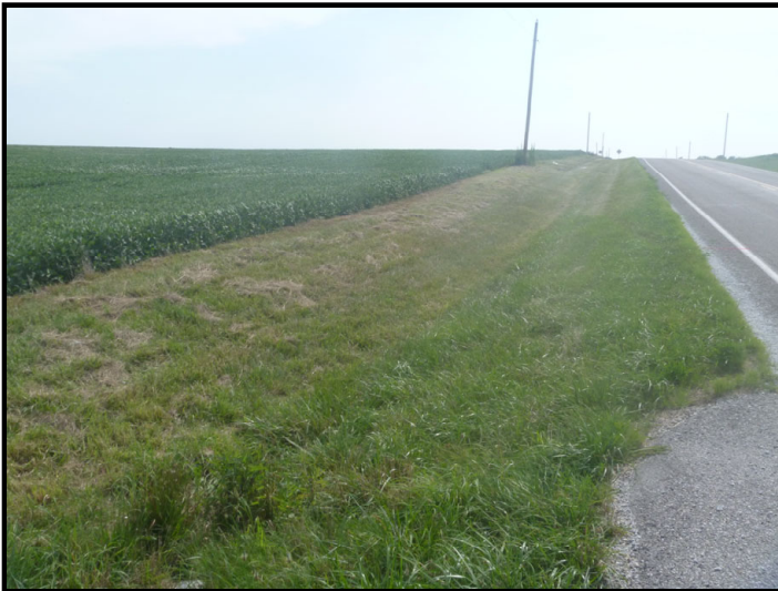
Photo 43 – Northeast Quadrant: Facing northeast along the north side of SR 18 in the northeast quadrant of the project area. The roadside ditch is a grassy swale.
