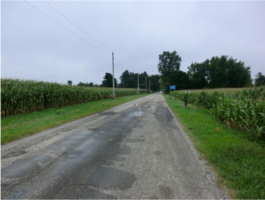
Photo 5. Main Street Near Location of Proposed Bridge Facing South
