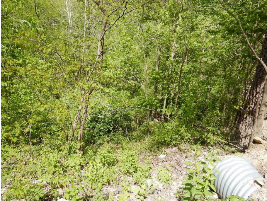
Photo 5. Facing west at outlet of drainage structure.
