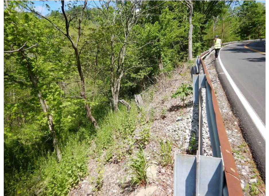
Photo 3. Facing north along west side of SR 7.
