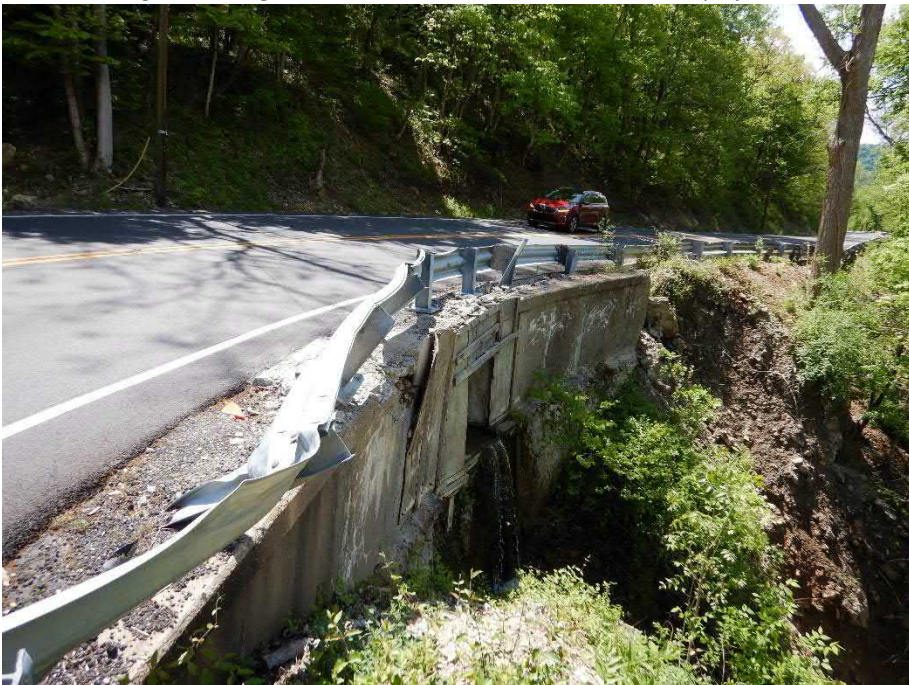
Photo 10. Facing southeast at outlet of culvert planned to be repaired.
