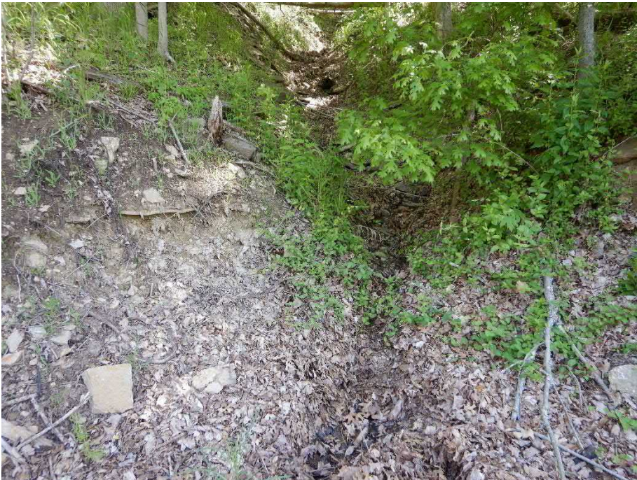
Photo 2. Facing east from structure drop inlet at upslope drainage pattern.
