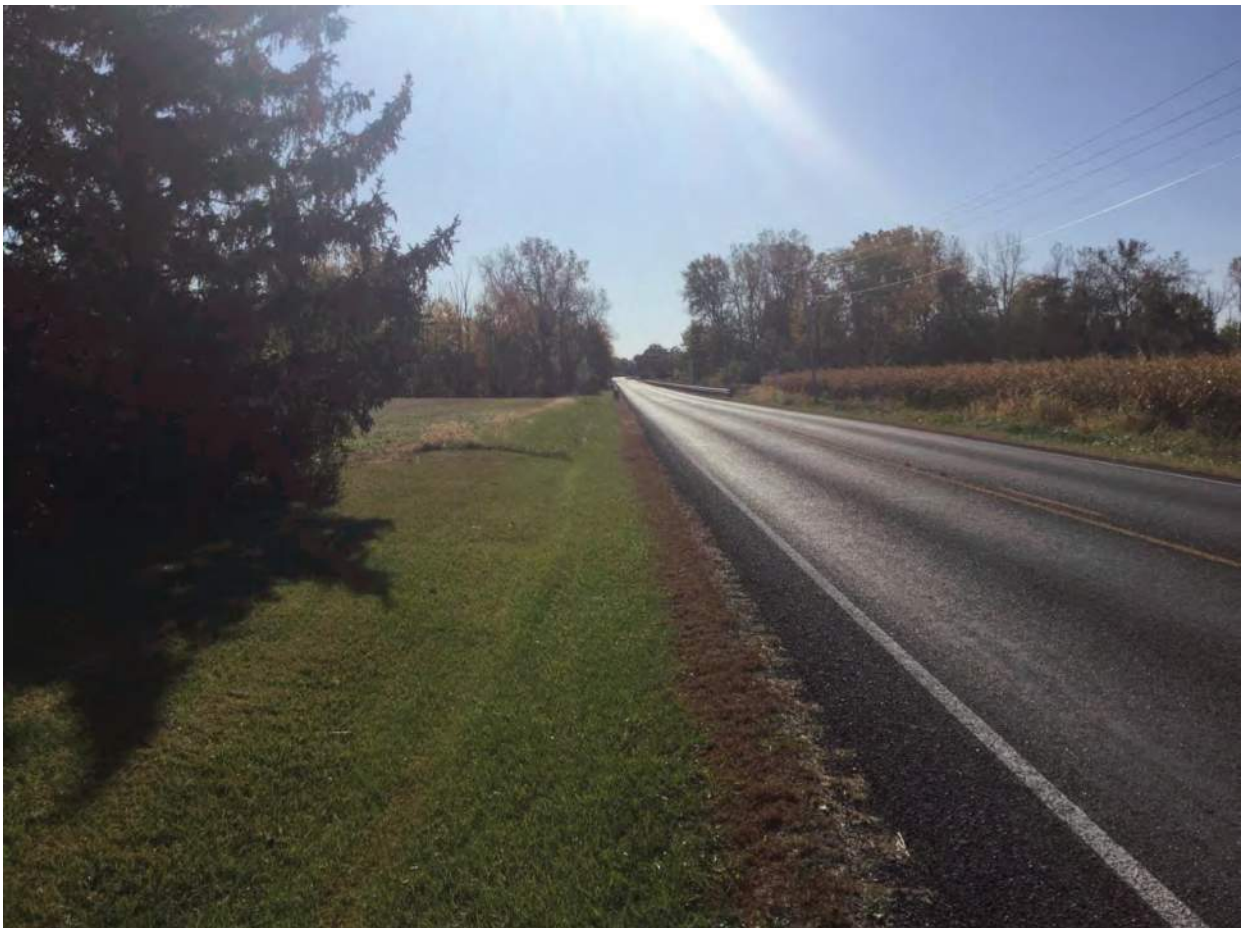
20. Looking southeast along roadside SR 116
