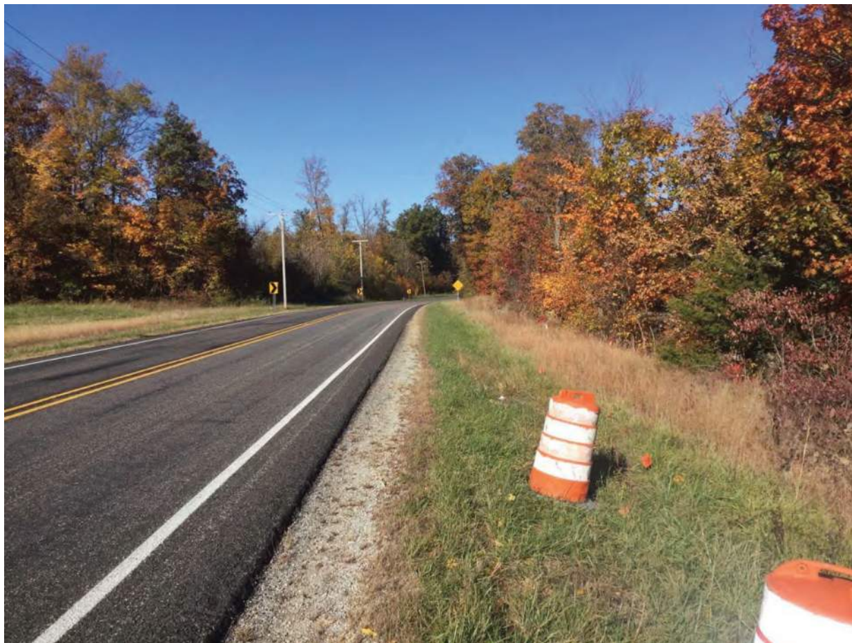
29. Looking west from roadside SR 116
