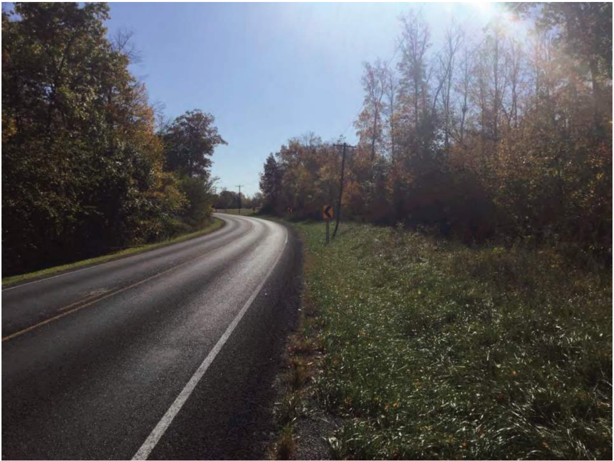
37. Looking southeast along roadside SR 116
