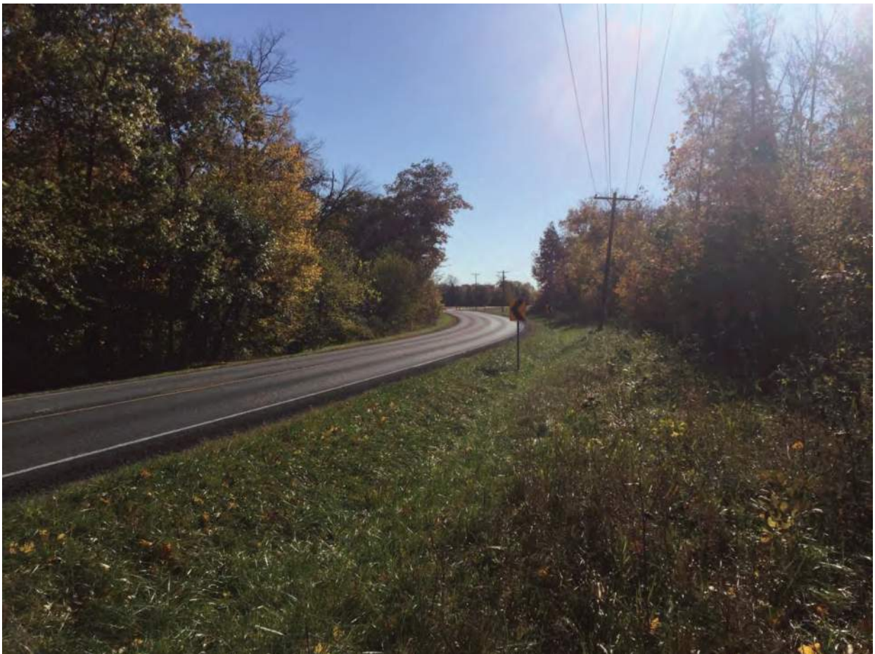
38. Looking southeast along roadside SR 116
