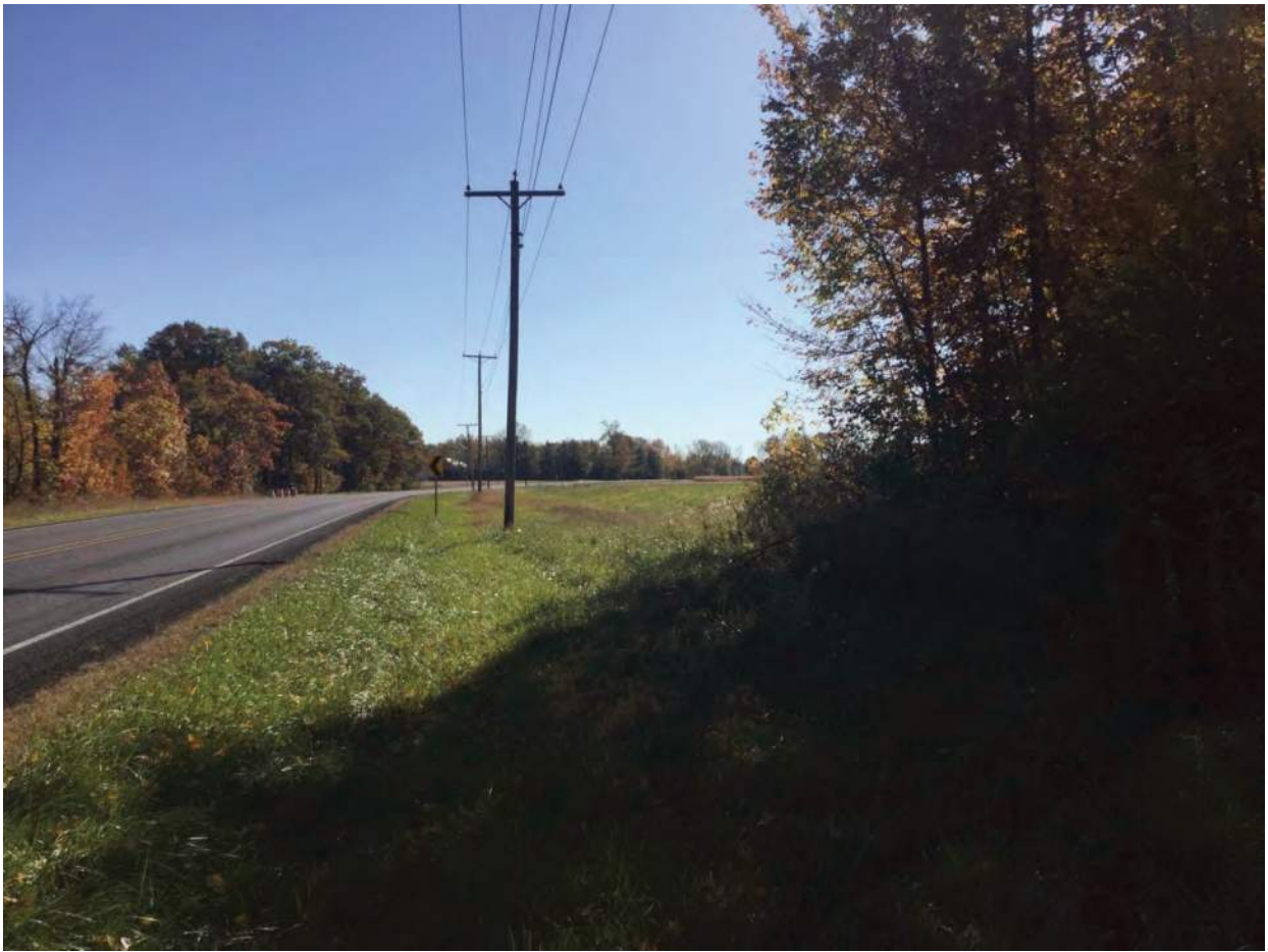
41. Looking southeast along roadside SR 116
