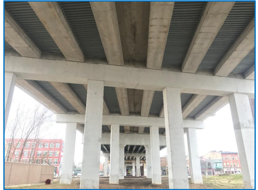
Photo 2 – View of the US 27 bridge facing south (3/12/2020).
