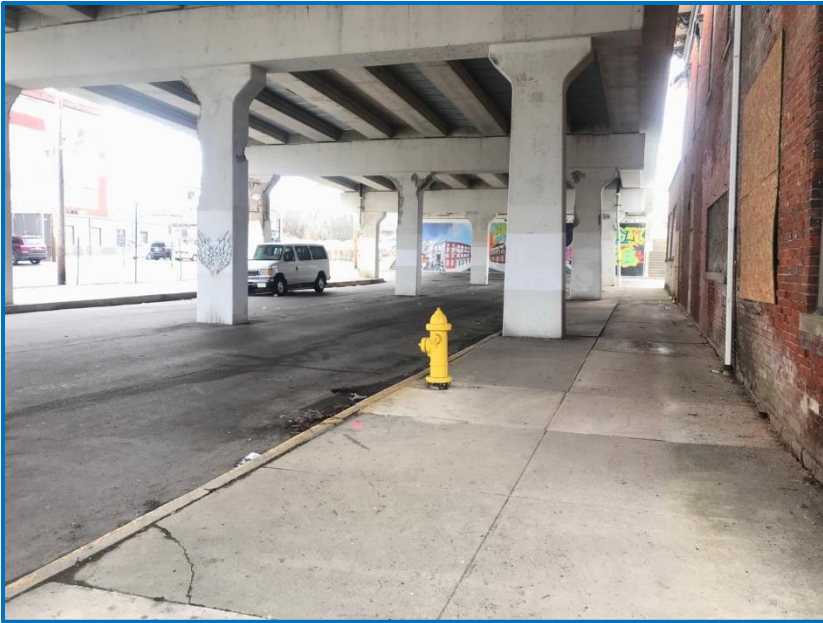
Photo 1 – View of the US 27 bridge facing south (3/12/2020).
