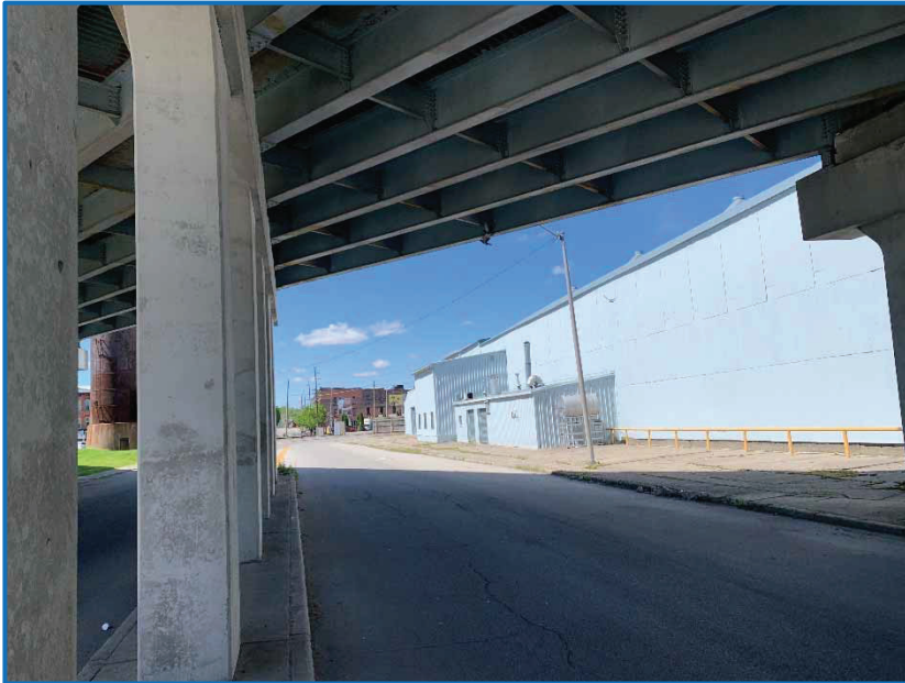
Photo 1 – View under the US 27 bridge facing southwest along Ft. Wayne Avenue (05/08/2021).
