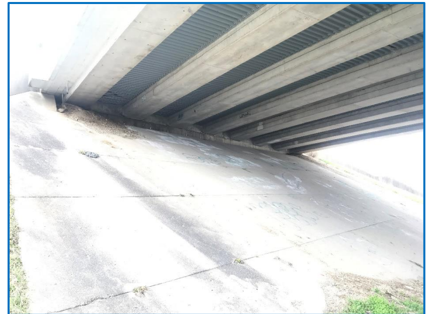
Photo 4 – View of the US 27 bridge facing northeast (3/12/2020).
