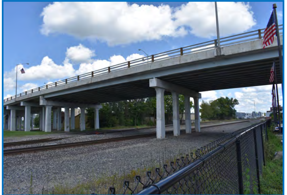
Photo 4—View of the US 27 Bridge over the NSRR, facing northeast (09/02/2018).
