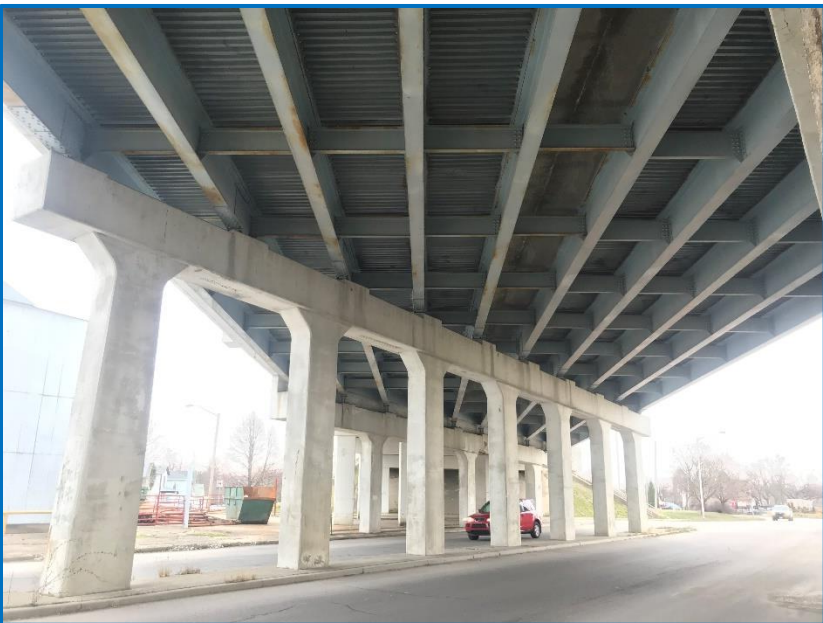
Photo 3 – View of the US 27 bridge facing north (3/12/2020).
