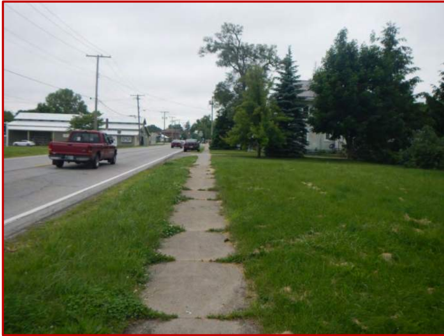
Photo 33. Looking north along investigated area located on the east side of SR 827, approximately 0.05 mile south of Pearl Street.
