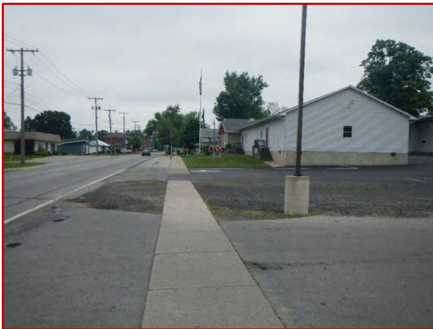
Photo 34. Looking north along investigated area located on the east side of SR 827, from just south of Pearl Street.
