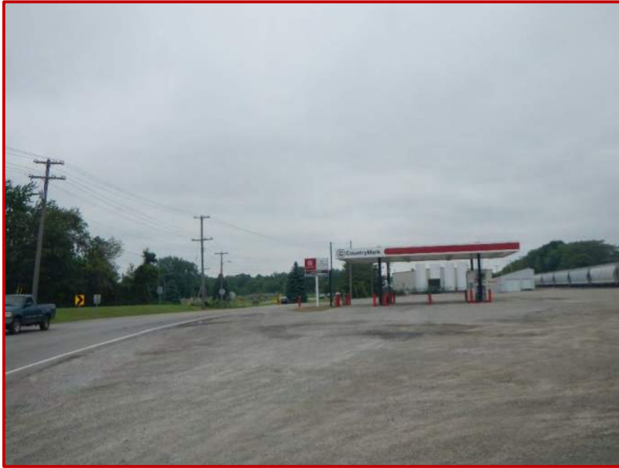
Photo 27. Looking north along investigated area located on the east side of SR 827, just north of Broad Street.
