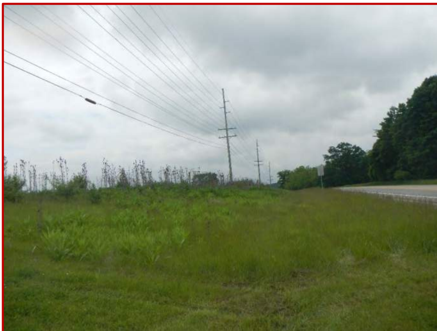
Photo 62. Looking south along investigated area located on the west side of SR 827, approximately 0.02 mile south of McSwain Drive.
