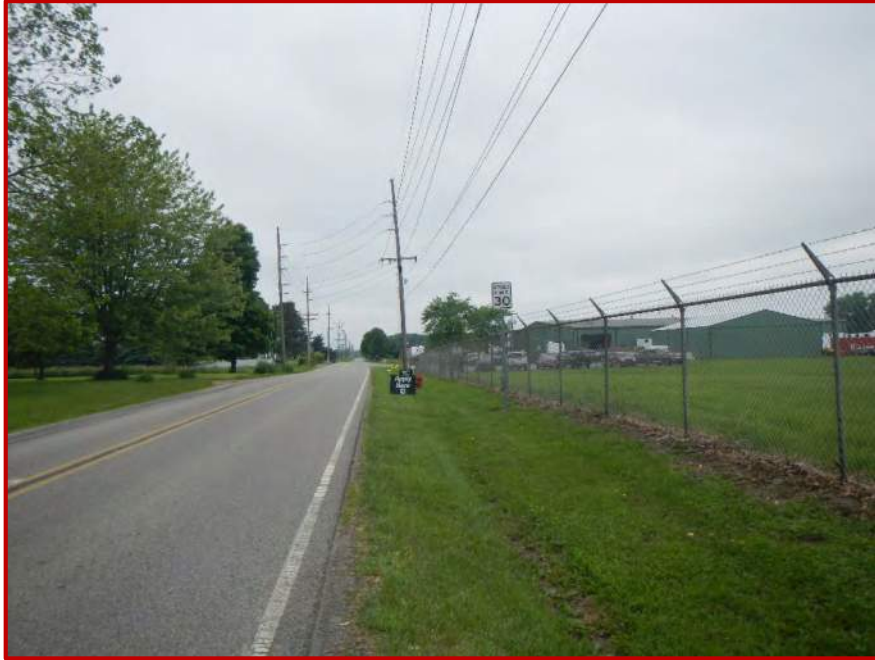
Photo 21. Looking west along investigated area located on the north side of Swager Drive, approximately 0.04 miles west of SR 827.
