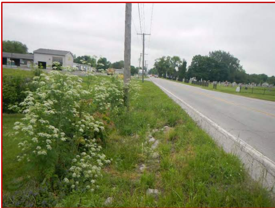
Photo 14. Looking north along investigated area located on the west side of SR 827, approximately 0.07 mile north of the Broad Street.
