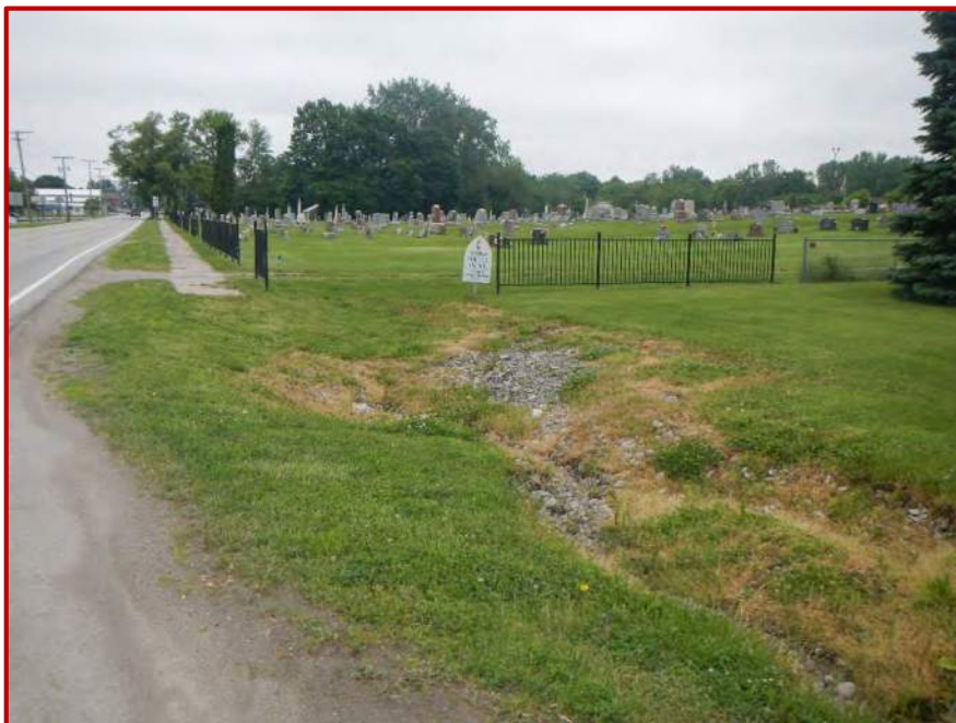
Photo 30. Looking north along investigated area located on the east side of SR 827, approximately 0.09 mile north of Broad Street.
