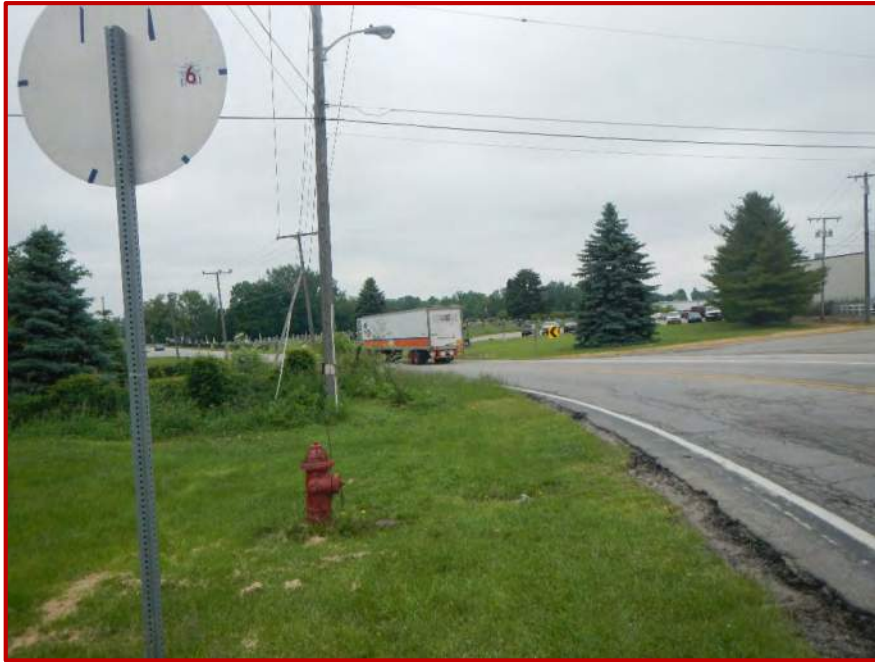
Photo 15. Looking northeast along investigated area located on the west side of SR 827 from approximately 0.04 mile north of the Broad Street.
