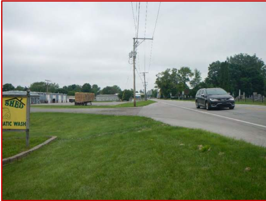
Photo 9. Looking north along investigated area located on the west side of SR 827 from approximately 0.1 mile south of Pearl Street.
