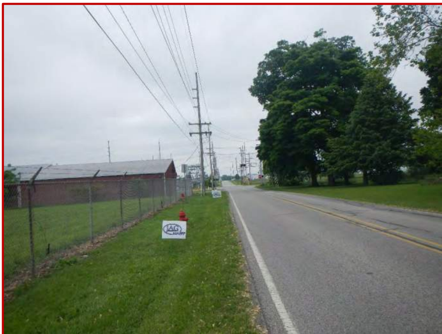
Photo 22. Looking east along investigated area located on the north side of Swager Drive, approximately 0.06 miles west of SR 827.
