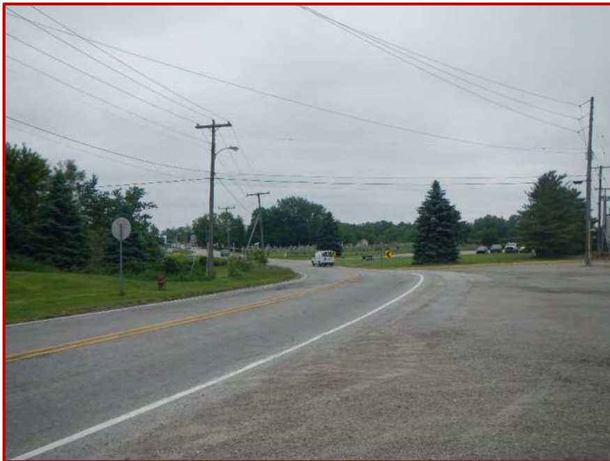
Photo 28. Looking north along investigated area located on the east side of SR 827, approximately 0.03 mile north of Broad Street.
