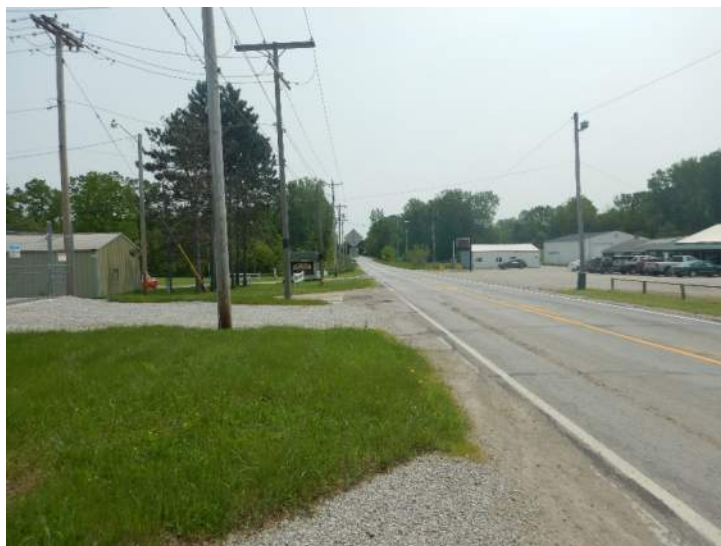
Photo 5: Looking east along SR 1 to project terminus.
