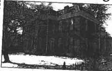
This Second Empire-style house at 288 Washington St. in St. Joe was once the home of a U.S. congressman. The house was rated "outstanding" on the just-released DeKalb County interim report on historic sites and structures completed by the Historic Landmarks Foundation of Indiana. The rating means the house has enough historic and architectural significance that it should be considered for listing on the National Register of Historic Places.
