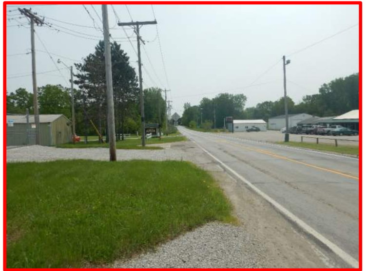
Photo 4: Looking east along SR 1 to project terminus.
