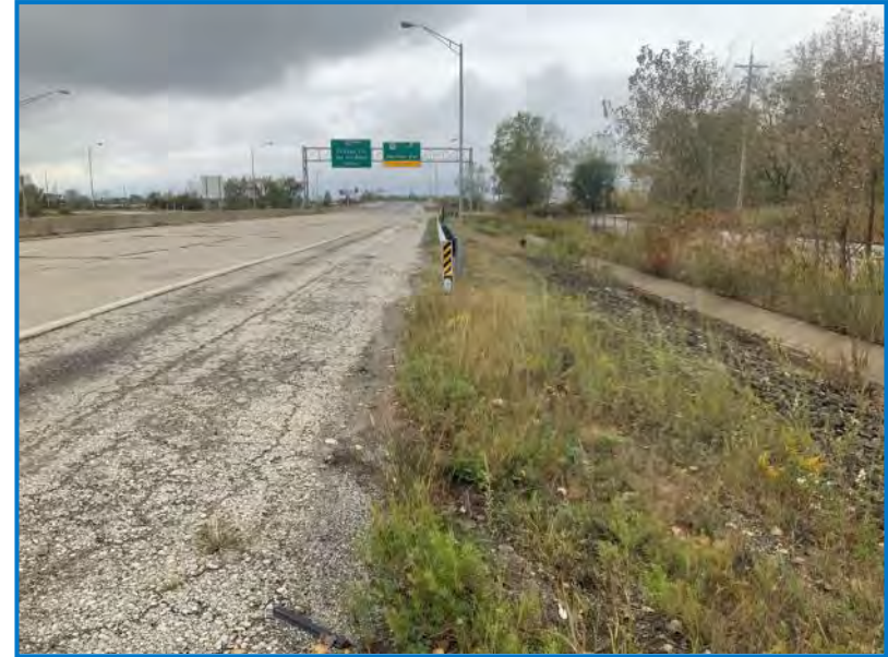
Photo 2 - View of the roadside along westbound SR 912 facing west (10/5/2021).
