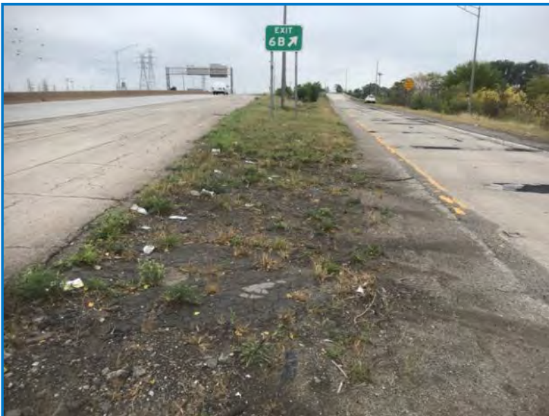
Photo 7 - View of the eastbound SR 912 exit ramp to Industrial Highway facing south (10/5/2021).
