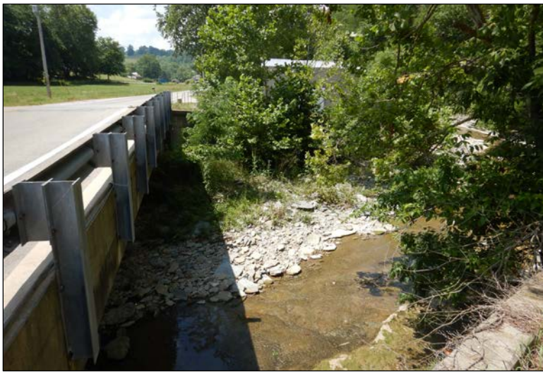
Photo 1: Looking south at SR 62 bridge over downstream side of Toddy's Branch.
