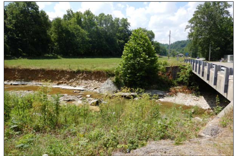
Photo 4: Looking south at SR 62 bridge over upstream side of Toddy's Branch.
