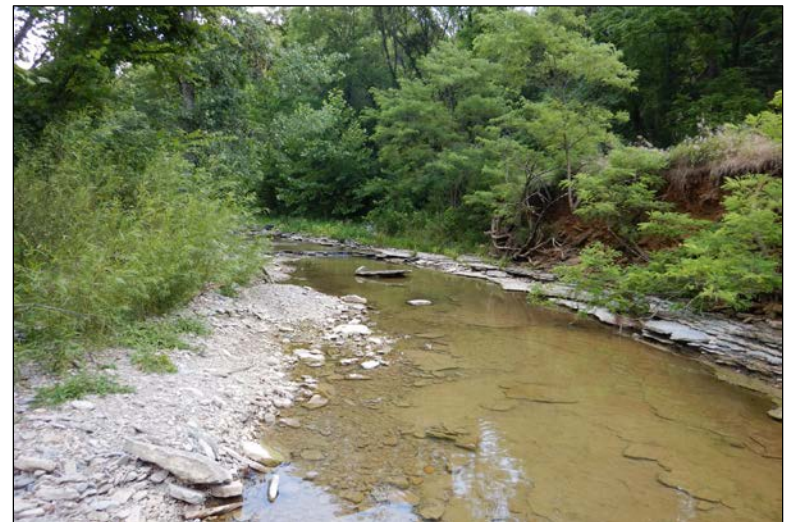
Photo 12: Looking downstream of SR 62 bridge and out of the project area. Note river right bank erosion and bedrock.
