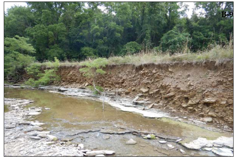
Photo 14: Looking upstream on Toddy's Branch just east of SR 62 at the severe bank erosion.
