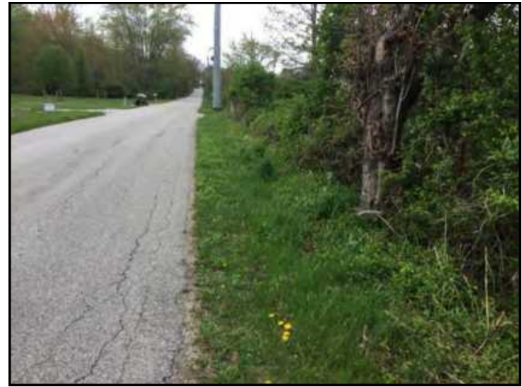
86. View of Barrett Switch Rd. ROW, looking west.
