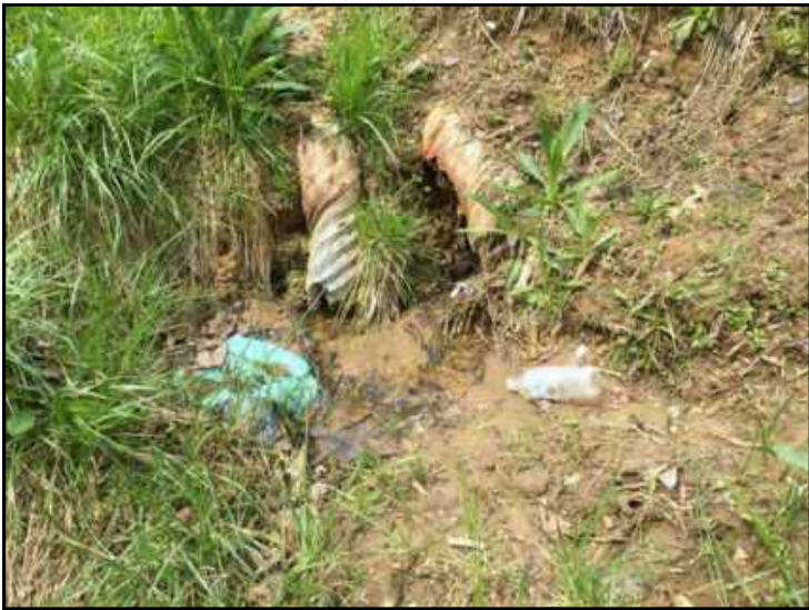
17. View of Culvert (CV) 1, looking northwest.
