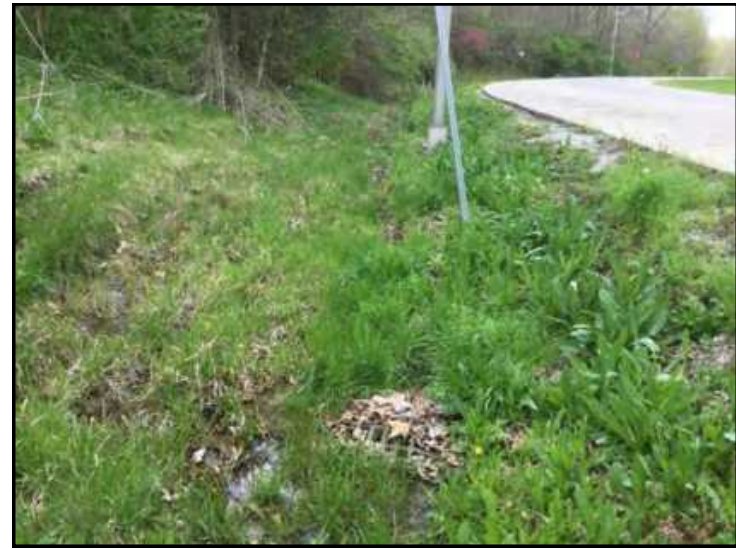
30. View of RSD 2, looking west.
