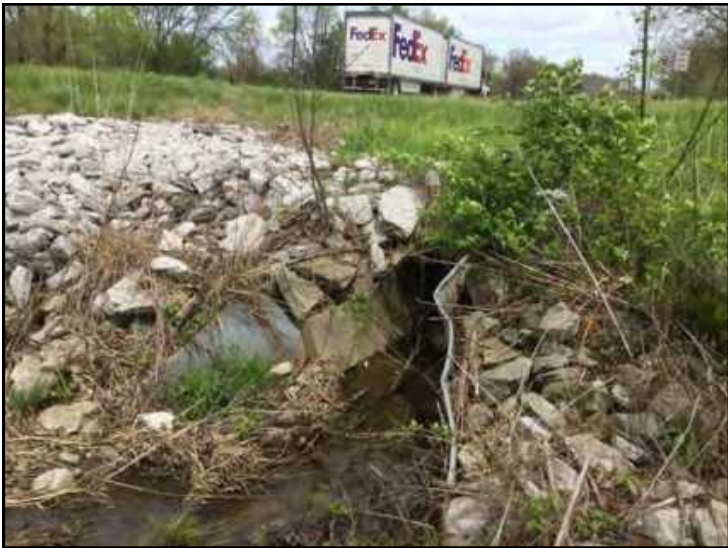
35. View of CV 6 inlet, looking northeast.
