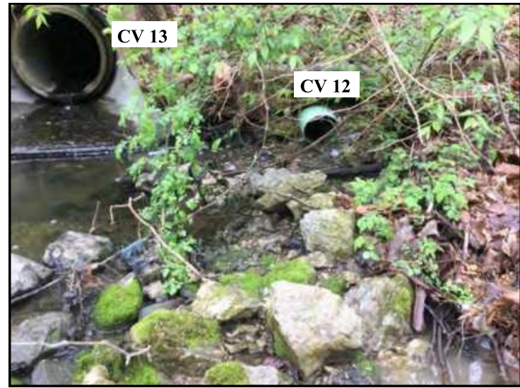
74. View of CV 12 and CV 13, looking south.
