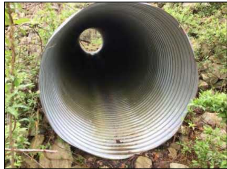
80. View inside of CV 14, looking southwest.
