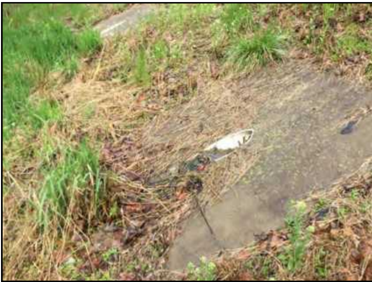
53. View of CV 9, looking southwest.
