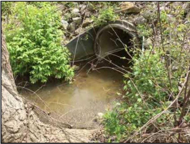
33. View of CV 4, looking southwest.
