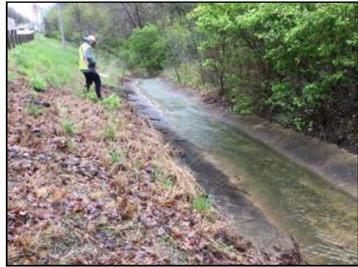
50. View of UNT 1 to Clear Creek, looking east.
