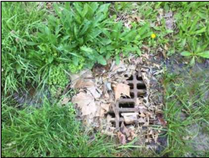
29. View of Storm Drain (SD) 1, looking north.
