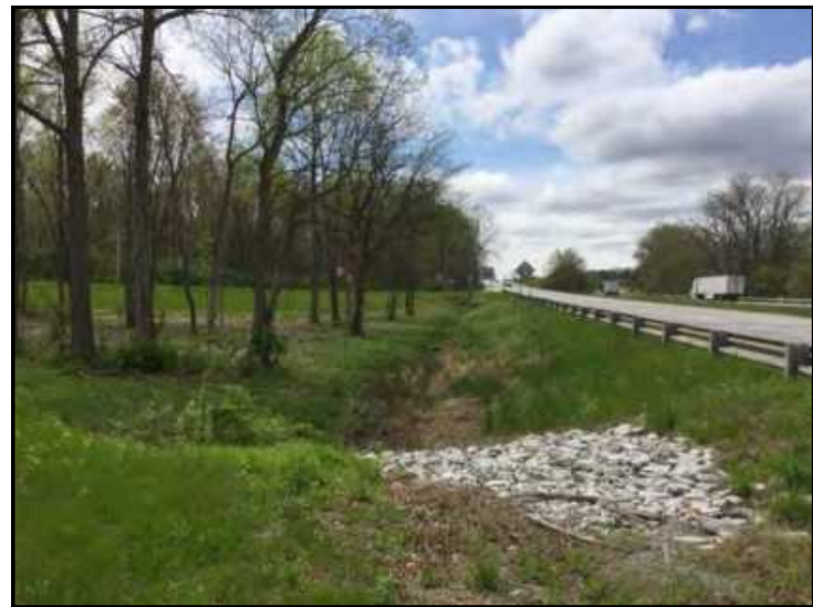
36. View of I-70 ROW, looking southwest.
