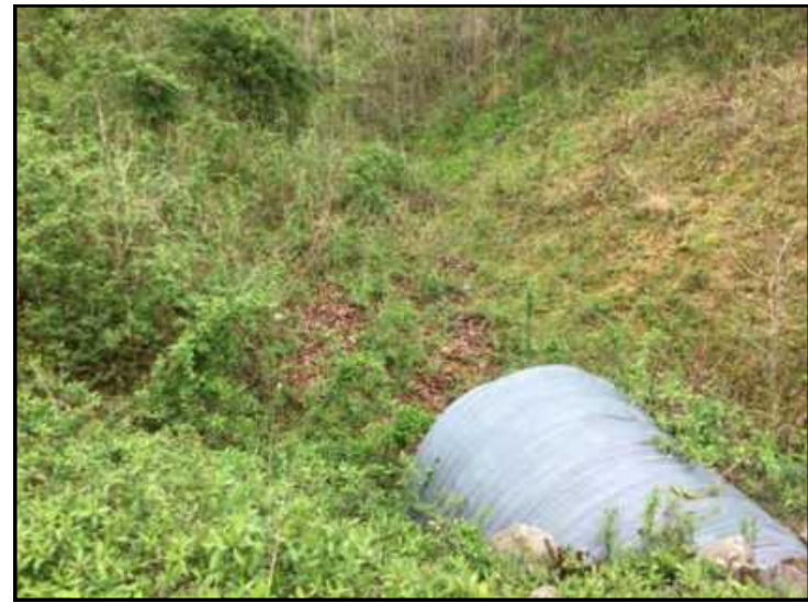
78. View of CV 14 inlet, looking southwest.
