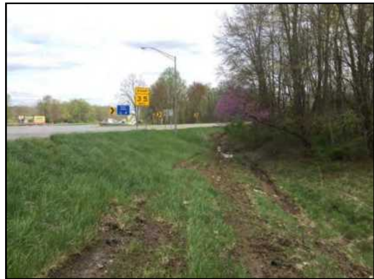
16. View of roadside ditch (RSD) 1 from northern limits of investigated area (IA), looking southeast.
