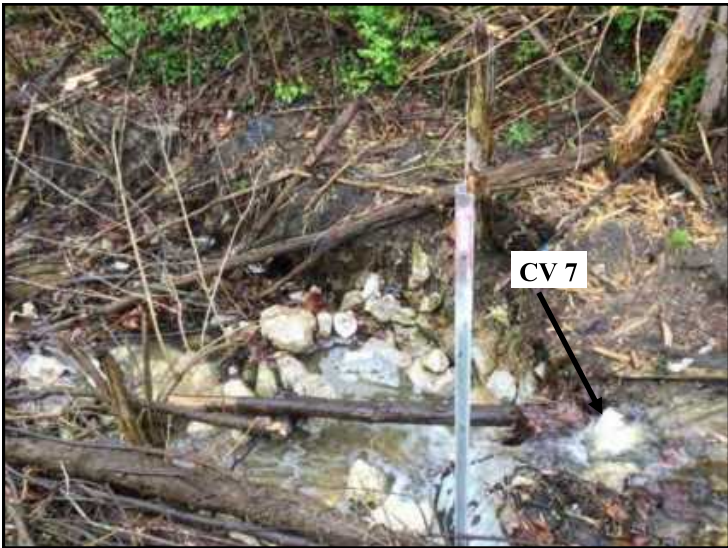
47. View of CV 7, looking south.
