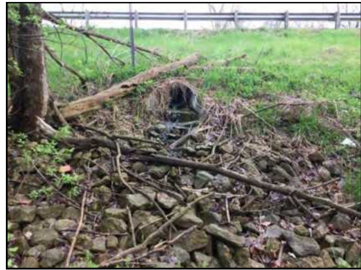
54. View of CV 10, looking north.
