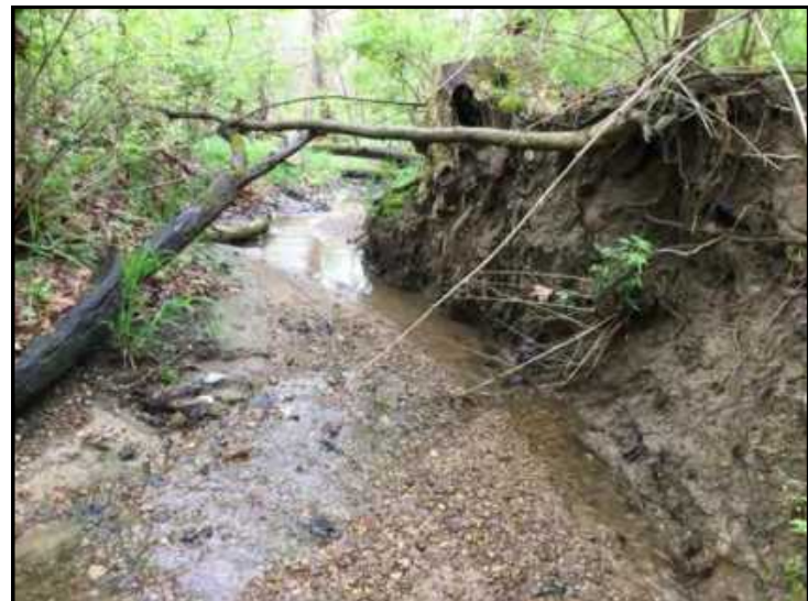
72. View of undercut banks in UNT 4 to Clear Creek, looking northwest.
