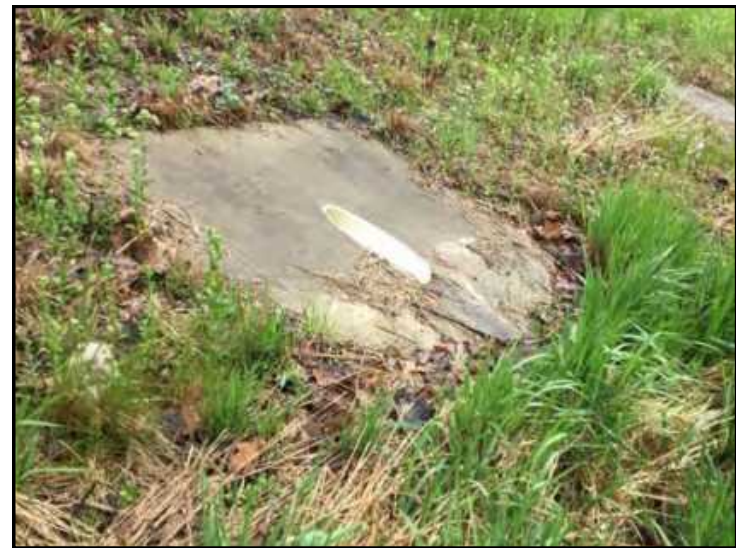
52. View of CV 8, looking northeast.
