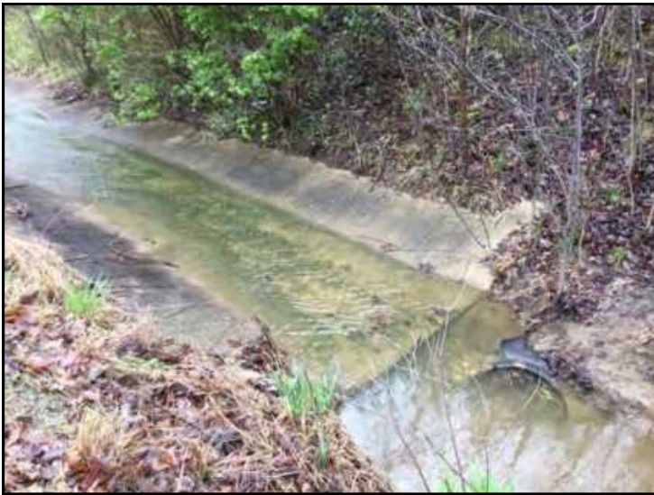
49. View of concrete ditch within UNT 1 to Clear Creek, looking northeast.
