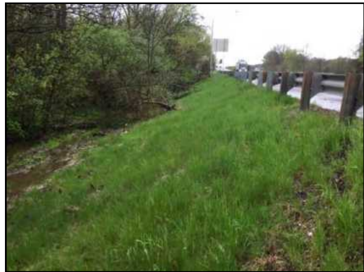
44. View of UNT 1 to Clear Creek and I-70 ROW, looking southwest.
