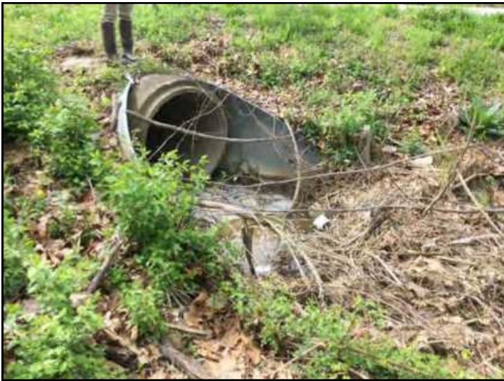
41. View of CV 6 outlet, looking northwest.
