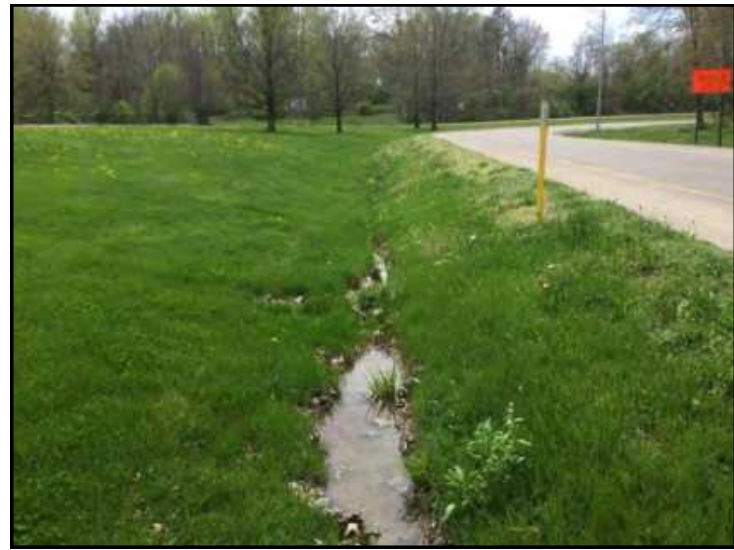
38. View of RSD 3, looking southwest.
