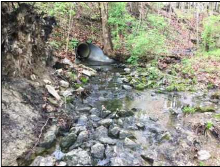
73. View of CV 13 and UNT 4 to Clear Creek, looking west.
