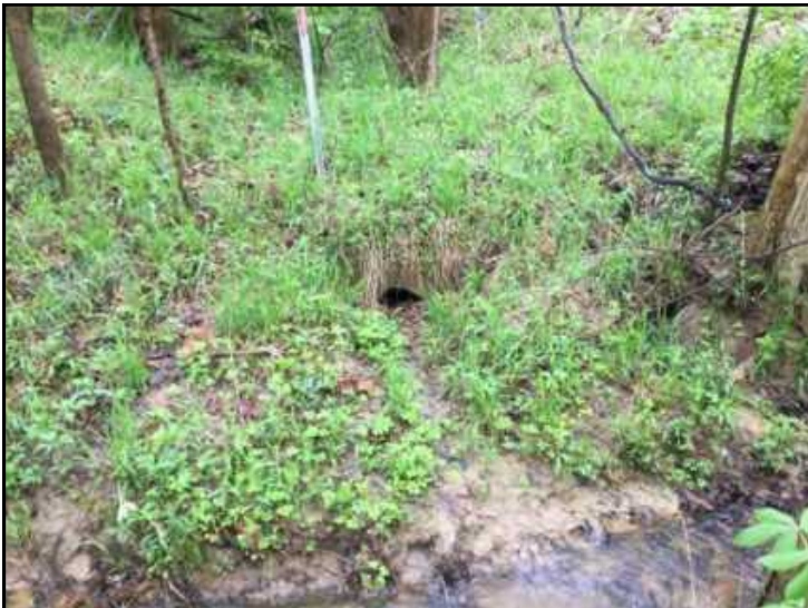
55. View of CV 11, looking south.
