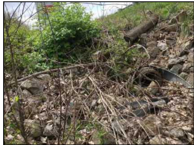
32. View of CV 3, looking northwest.
