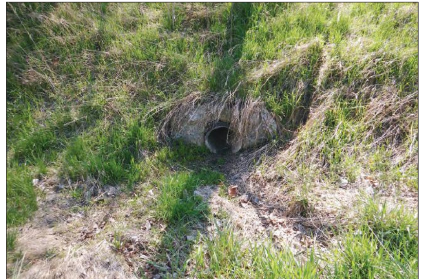
Photo 20: Culvert inlet to the east of S.R. 9, facing east.
