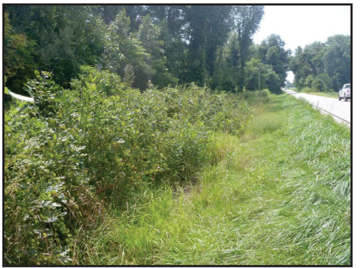
Photo 90 – Northeast Quadrant, Wetland A and RSD-3: Facing south along Wetland A and RSD-3 from the northern terminus of the AOI. The northern segment of Wetland A is confined to RSD-3.
