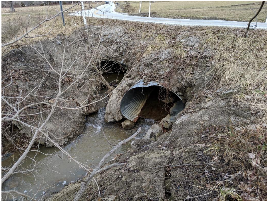
Figure 4 South end of existing structure.
