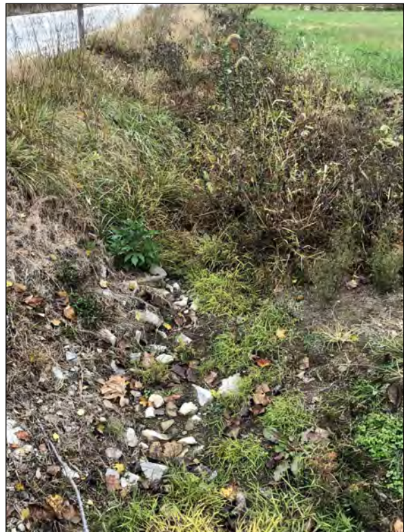
Picture 12—UNT to Kiper Creek; north view; 16 Oct 19.
