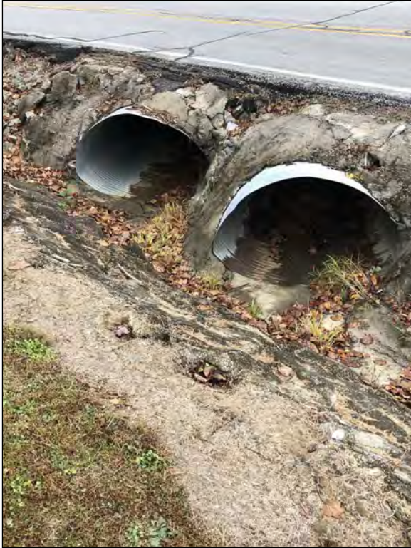
Picture 1—UNT to Kiper Creek; southwest view; 16 Oct 19.
