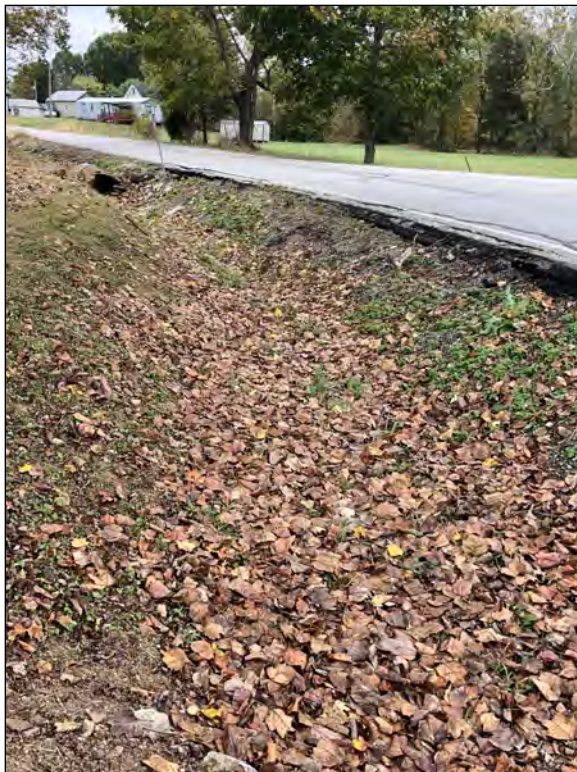
Picture 27—RSD2 , southeast view; 16 Oct 19.
