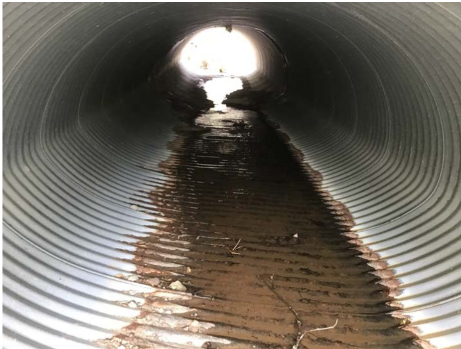
PHOTO 6 Condition Description Inside South Pipe facing West
