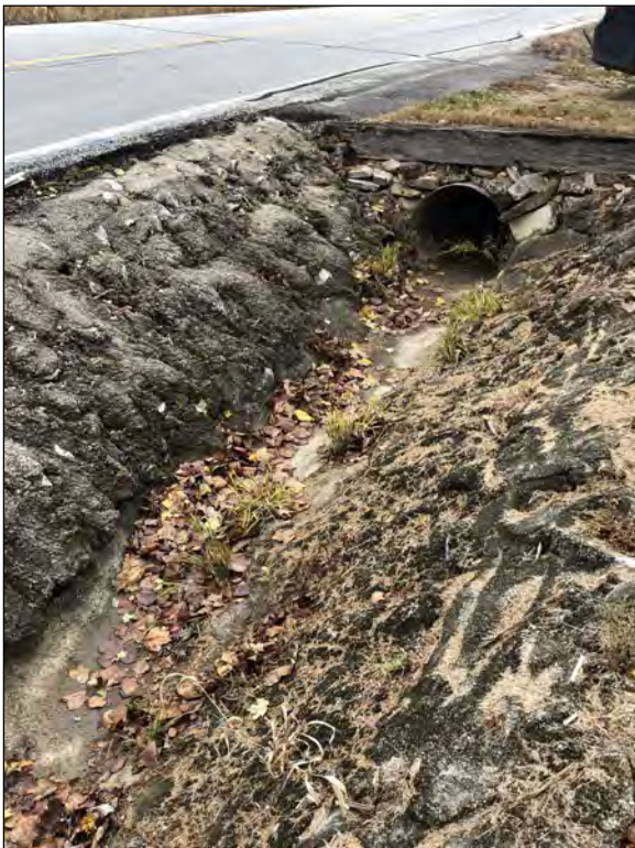
Picture 3—UNT to Kiper Creek; northwest view; 16 Oct 19.
