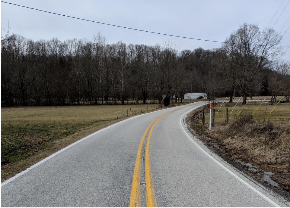
Figure 1 Road alignment looking west.
