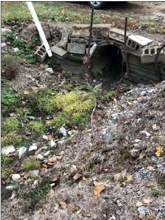
Picture 11—UNT to Kiper Creek; southeast view; 16 Oct 19.
