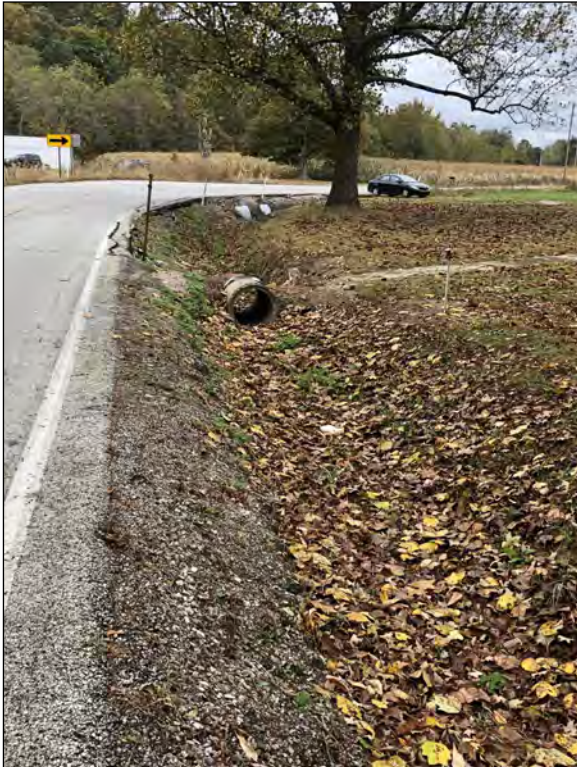
Picture 33—Southeast quadrant, northwest view; 21 APR 2020.
