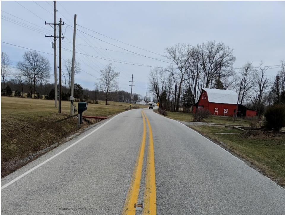
Figure 2 Road alignment looking east.
