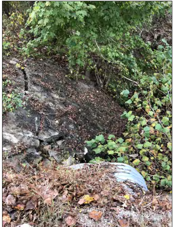
Picture 2—UNT to Kiper Creek, southwest view; 16 Oct 19.
