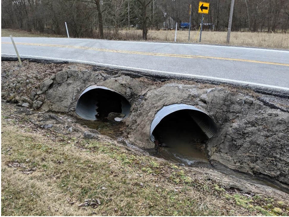
Figure 3 North end of existing structure.
