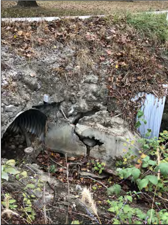
Picture 5—UNT to Kiper Creek; southeast view; 16 Oct 19.
