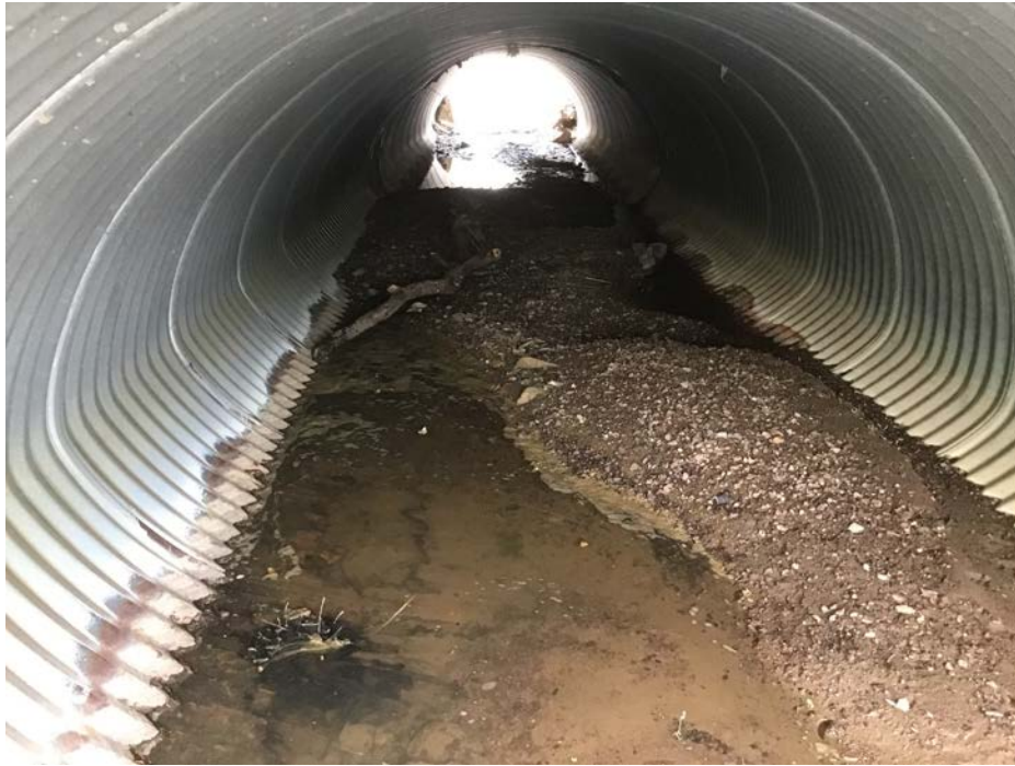
PHOTO 3 Condition Description Inside North Pipe facing West
