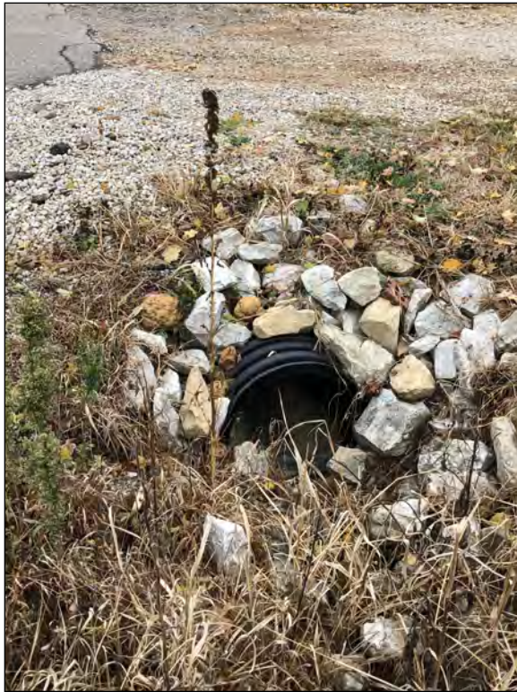
Picture 23—RSD1 pipe; south view; 16 Oct 19.
