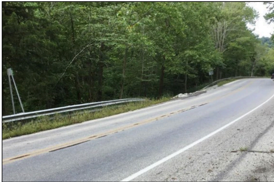
Guardrail along SR 1
