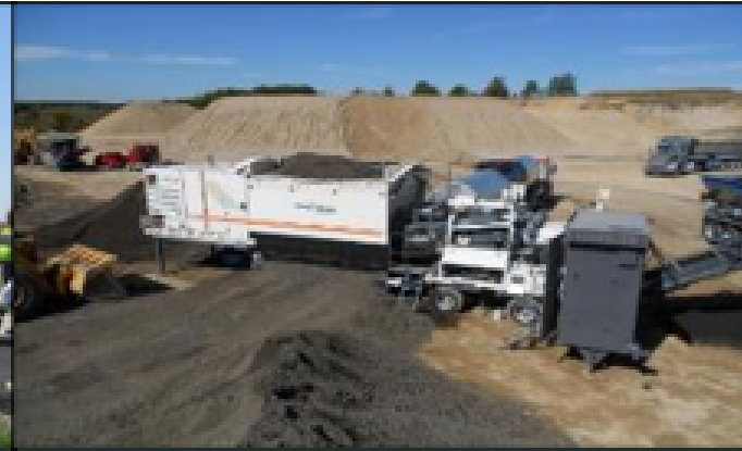
Cold Central Plant Recycle (CCPR)
