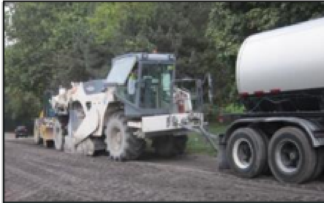
Full Depth Reclamation (FDR)
