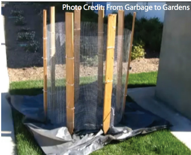
Figure 12: This picture shows one of two compost bins that were constructed by students at Arroyo High School. Photo: www.coolcalifornia.org
