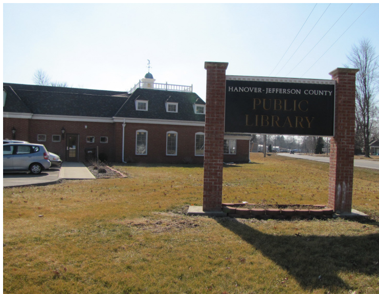
Hanover town library, located along State Road 56/62
