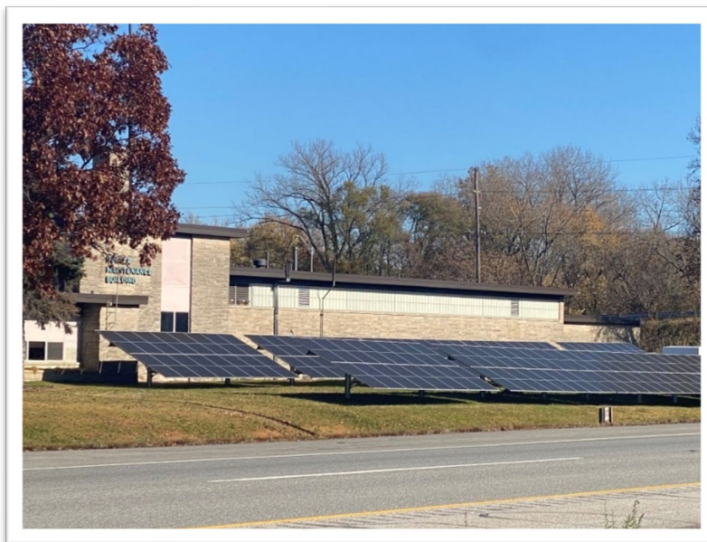
Image 5.1: Maintenance Unit 1 Solar Panel Layout
