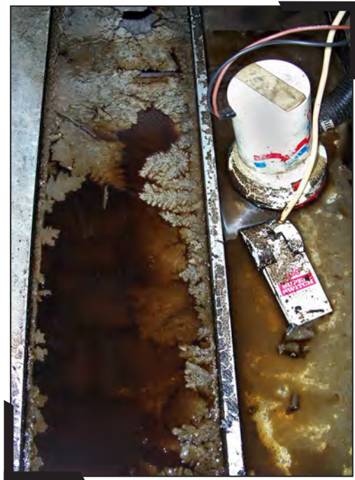
The use of a bilge sock would help prevent oil collected in the bottom of this bilge from being discharged to the lake (Photo by Joe Exl, IDNR).
