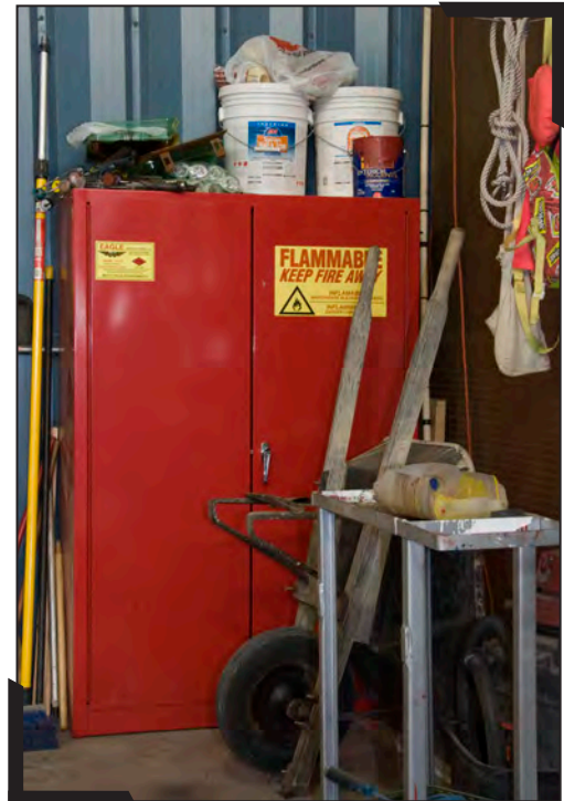
Storage cabinets may contain hazardous materials.
