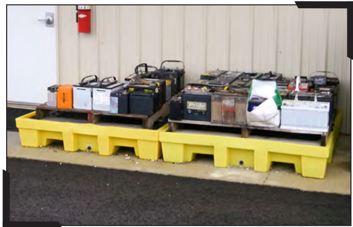
Spent lead acid batteries should be stored in an area with secondary containment or in an area that provides a means to control and contain any battery acid spillage (Photo by Cathy Csatori, IDEM).
