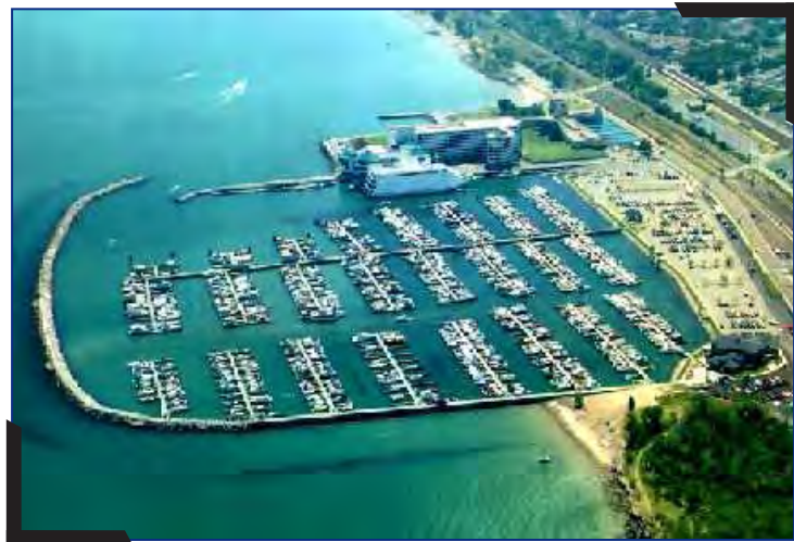
The Hammond Marina located on Indiana's Lake Michigan shoreline was built in 1991 on a former Brownfield site. The shoreline consisted of steel slag. The 54-acre complex was carved out of the steel mill slag and the shoreline was created from dredged sand, which created a mile-long sandy beach (Source: Hammond Marina).
