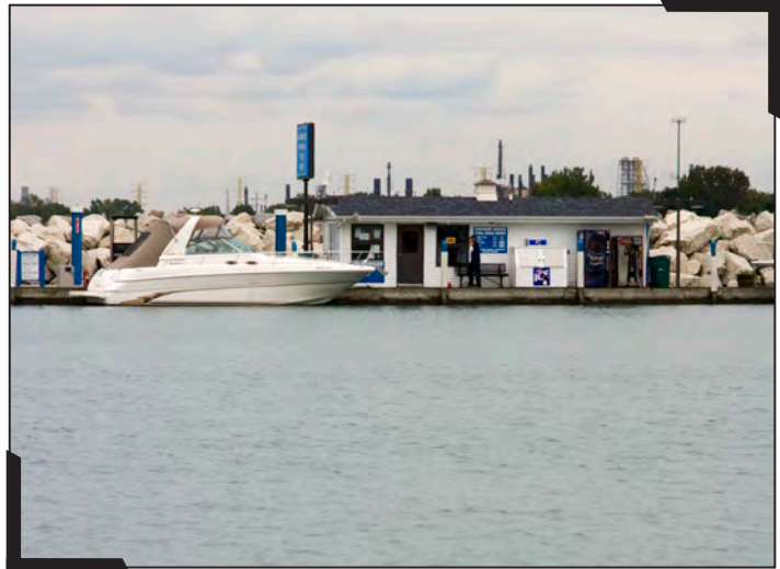
This fueling station is at the Hammond Marina.
