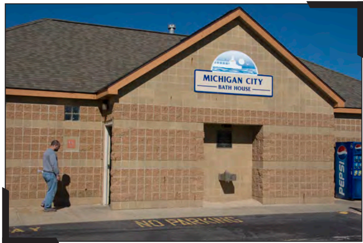
This bath house and public restroom is located at Washington Park Marina.
