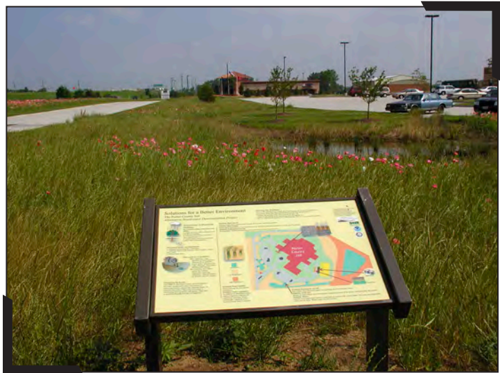
This rain garden installed in Porter County captures and treats run-off from the parking lot (Source: Indiana Lake Michigan Coastal Program).
