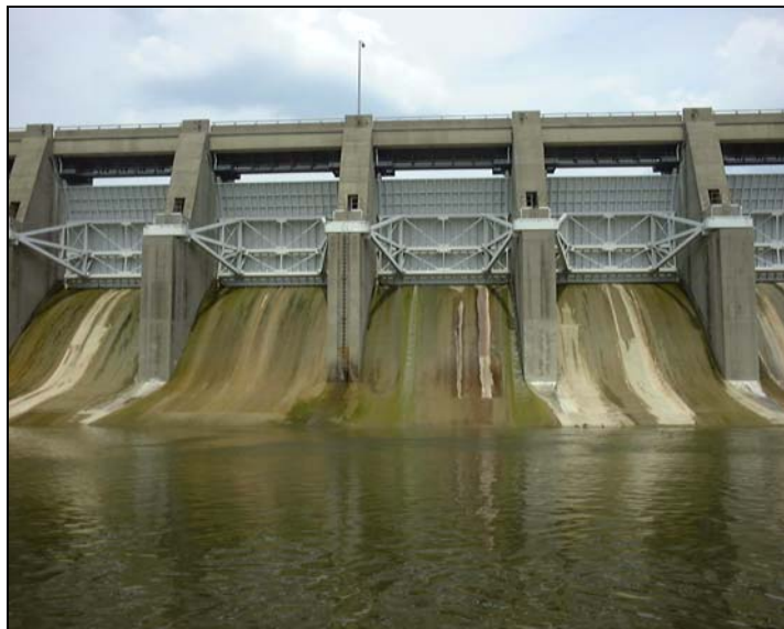
Figure 8-5 Downstream view of gates on a central-Indiana dam.
