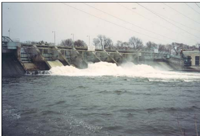
Figure 4-8 Dam with significant concrete spillway structures.
