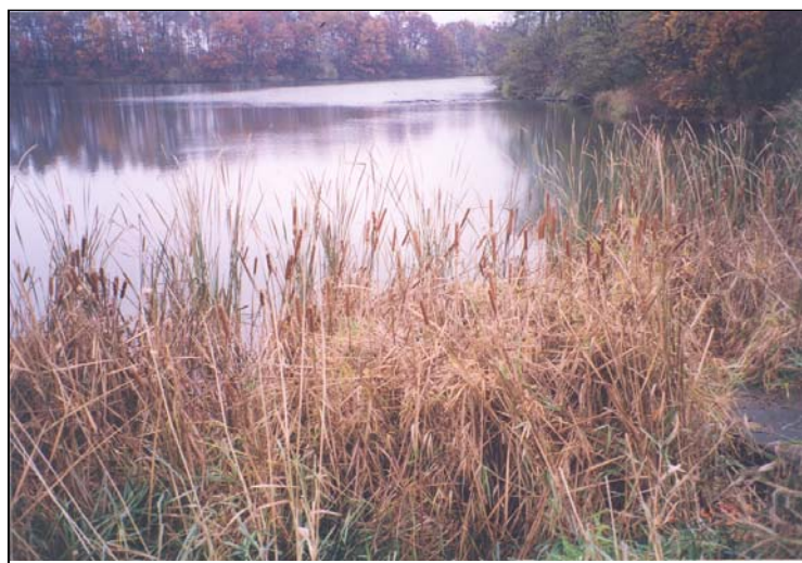
Figure 8-4 Excessive vegetation in reservoir almost completely conceals the spillway riser.
