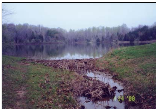
Figure 6-50 Beavers have blocked this spillway.
