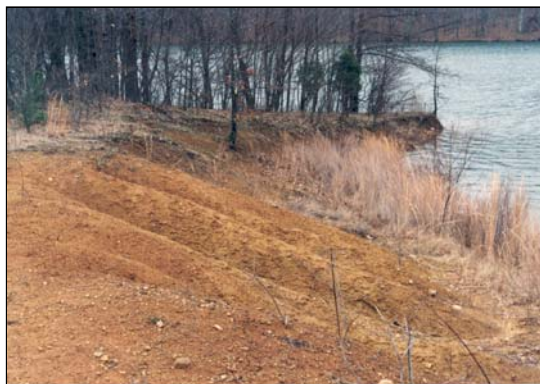
Figure 8-3 This reservoir has severe shoreline erosion due to inadequate vegetation.
