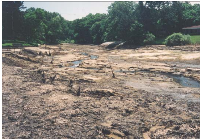
Figure 1-3 Dam breach failures cause significant downstream damage.
