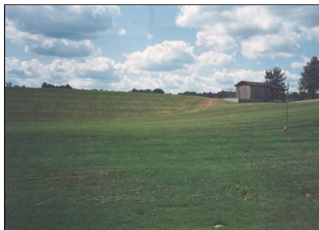
Figure 6-45 A building constructed in the emergency spillway obstructs flow and poses a safety risk to the building.
