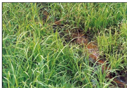
Figure 5-41 This seepage has produced iron oxide stains.
