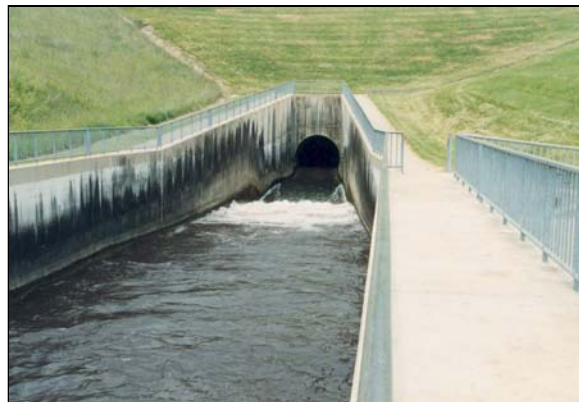
Figure 6-33 Inspecting a spillway that has flowing water is very difficult.
