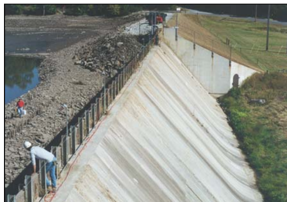
Figure 4-9 Dam requiring extensive concrete inspection.
