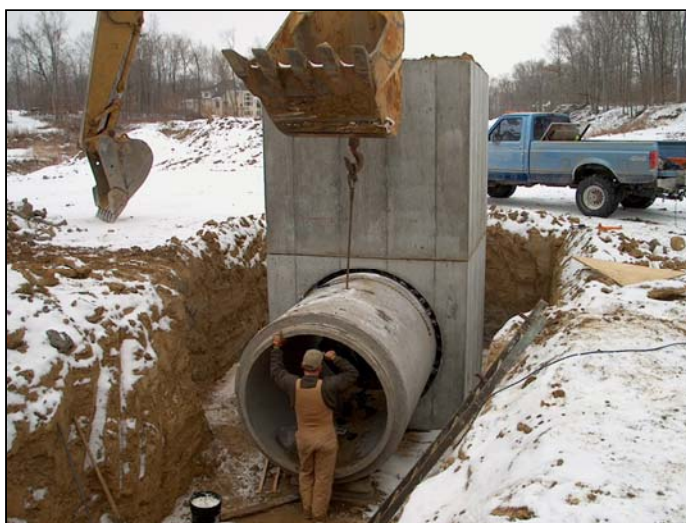
Figure 3-7 Installation of a riser pipe during winter weather.
