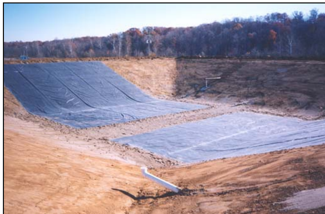
Figure 6-42 A geomembrane liner being installed in a waste water reservoir.
