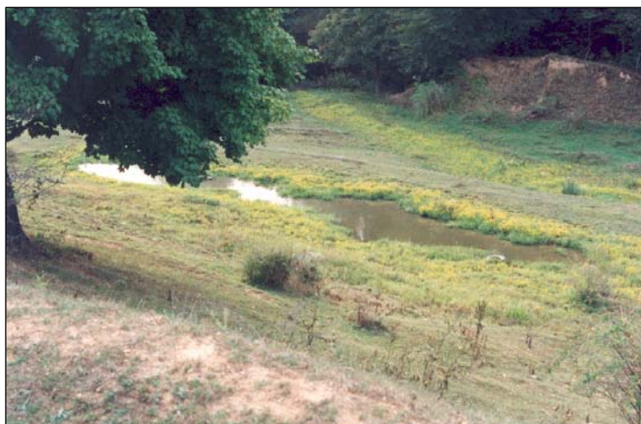
Figure 5-42 Excessive seepage near embankment toe.
