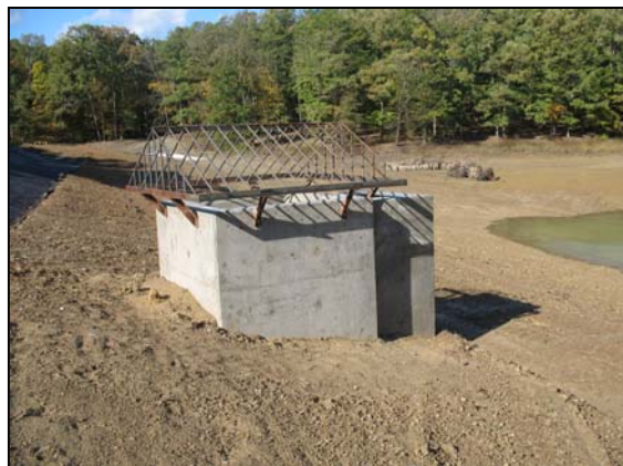
Figure 3-6 Construction photograph of spillway and embankment rehab.
