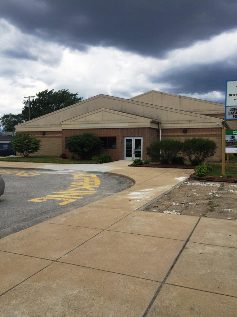
South Side (Front) of Building (Primary Area of Improvements)
