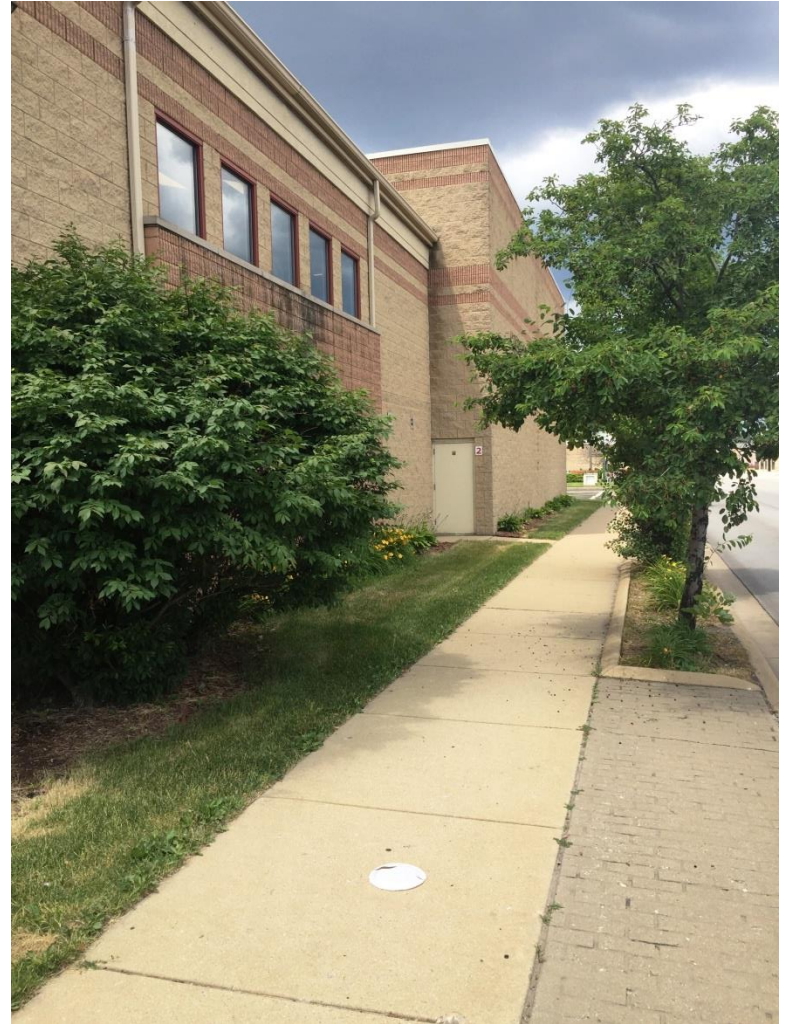
Looking North Along East Face of Building (2)
