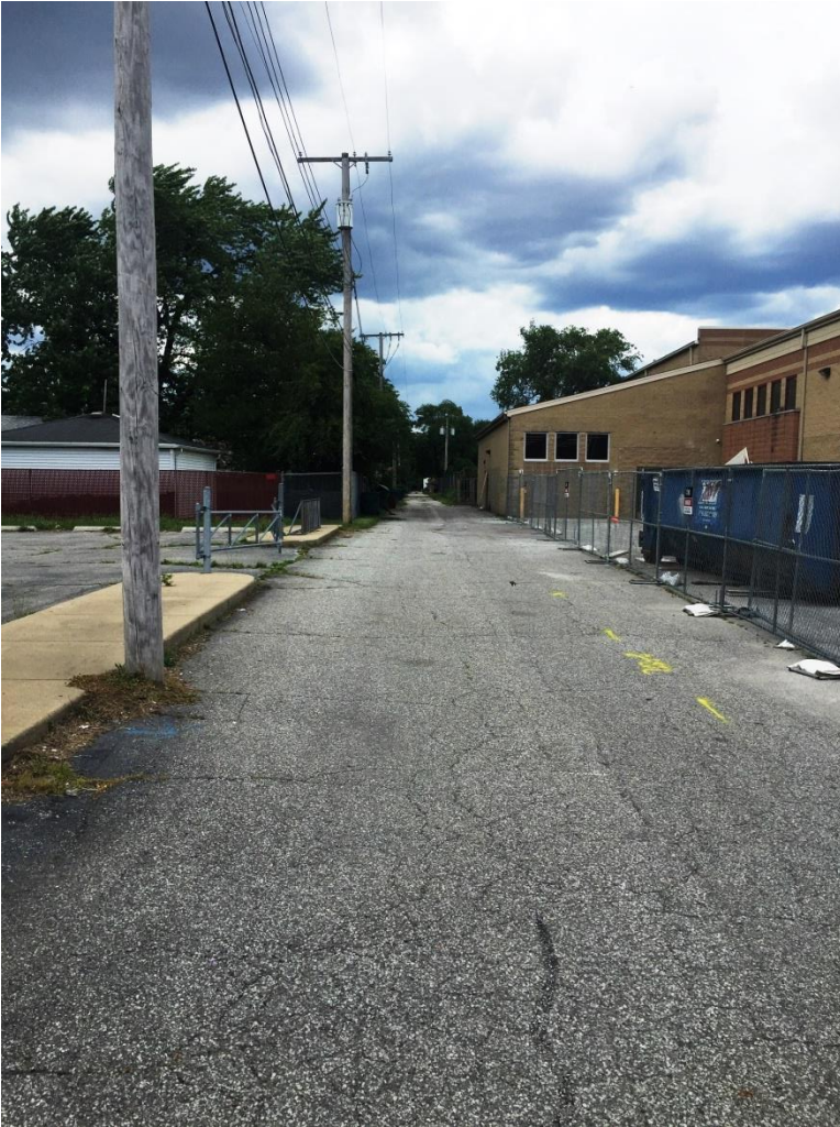
Alley West of Building & East of Existing Parking Lot
