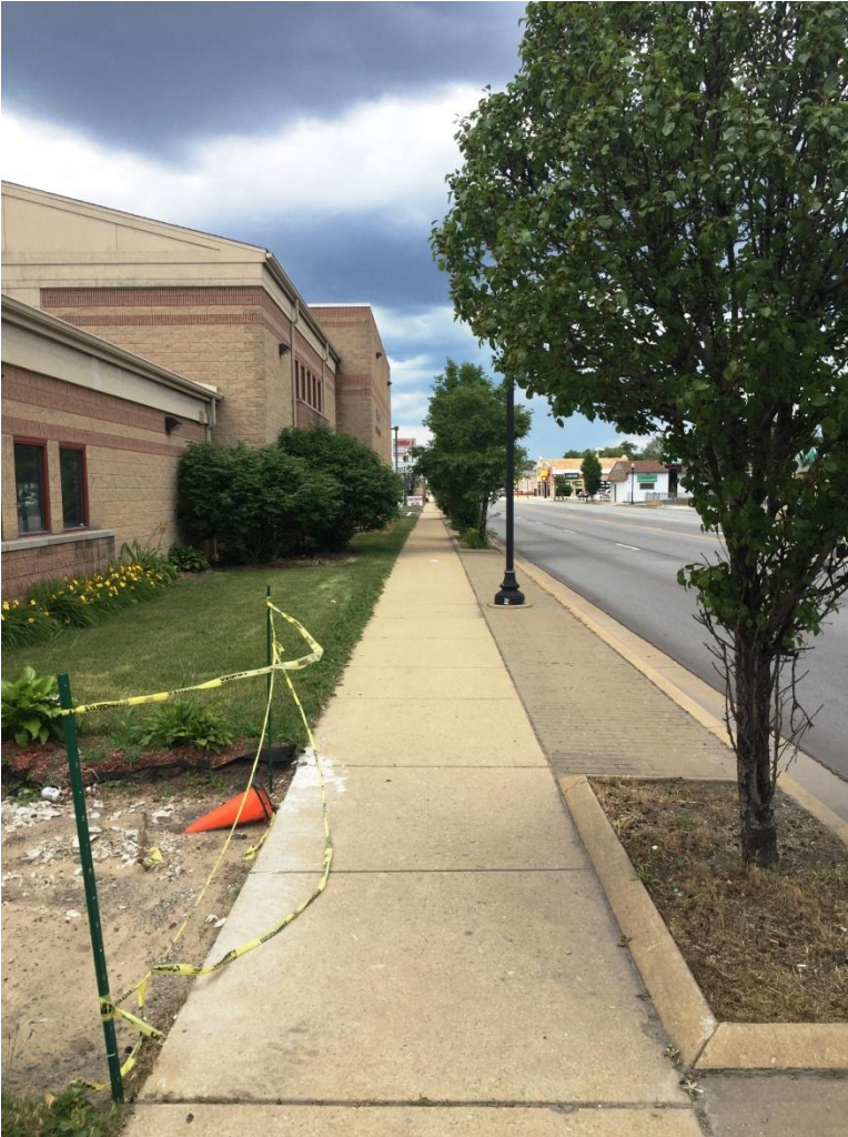
Looking North Along East Face of Building (1)
