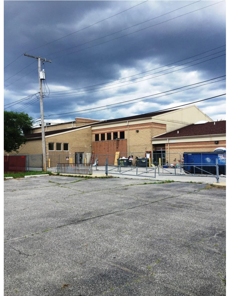
Southwest Side of Building (2) (Showing Area for New Canopy & Bus Drive)
