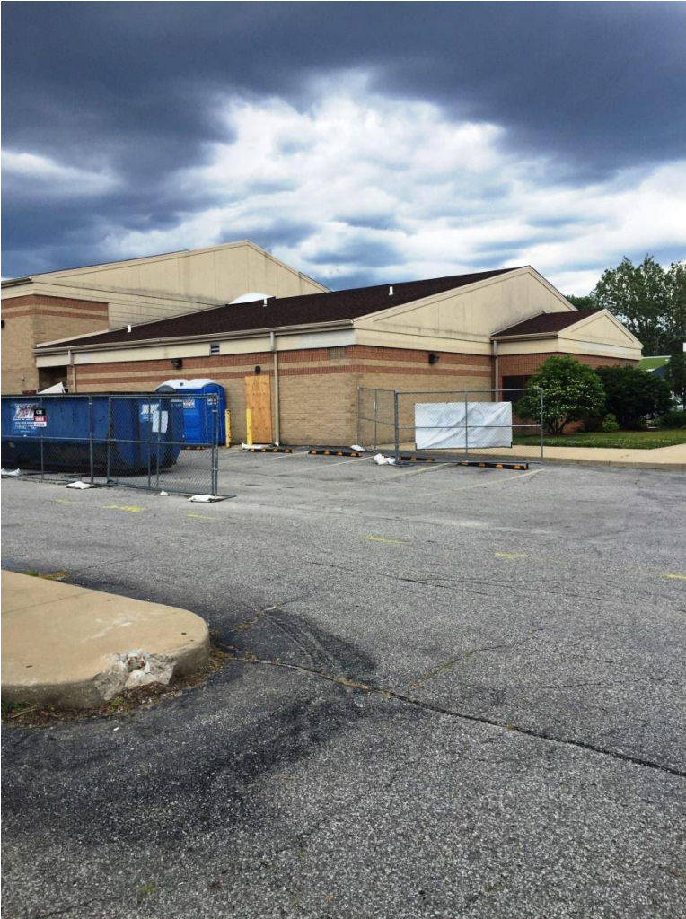
Southwest Side of Building (1) (Area for New Bus Drive Along West Face of Building)
