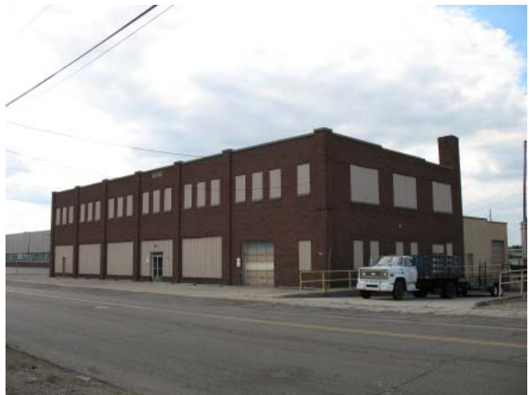
Photo 8: Plank Brothers Salvage and Auto Parts in Muncie (Delaware County).
