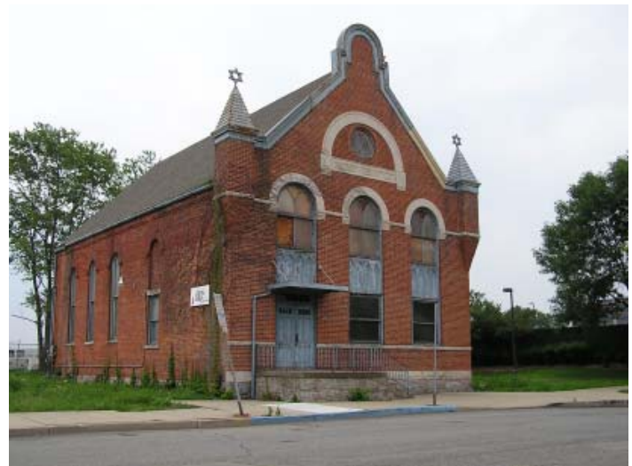
Photo 53: The Sons of Israel building has been purchased and will be converted into housing.
