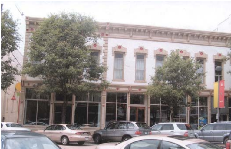
Photo 6: Joseph Hilger's White House Dry Goods Store's 1882 store front location.
