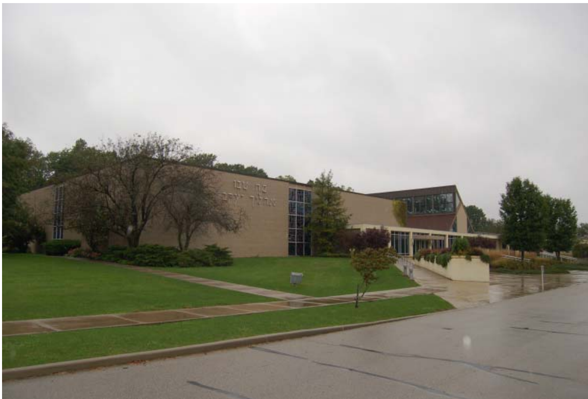
Photo 35: Congregation Beth-El Zedeck in Indianapolis (Marion County). This building was constructed in 1958, with a remodel in 2002.
