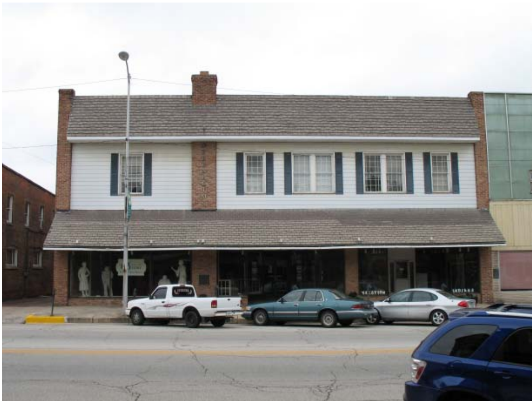
Photo 68: This building was the location of the Oppenheim Store in North Manchester.
