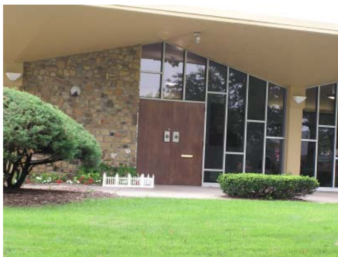
Photo 52: The 1971 Orthodox synagogue in South Bend (St. Joseph County).
