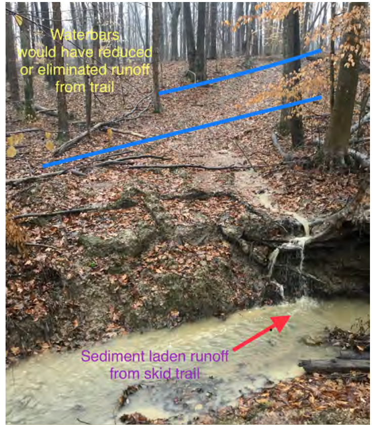
Lack of water diversions on this trail is causing active erosion, leading to sediment-laden runoff reaching the stream.
