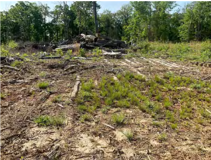
In this pine clearing, the smaller pine trees that were not marketable were used to stabilize the log landing area, as pine plantings can be quite wet. This allowed the landing to be stable even during wetter periods.
