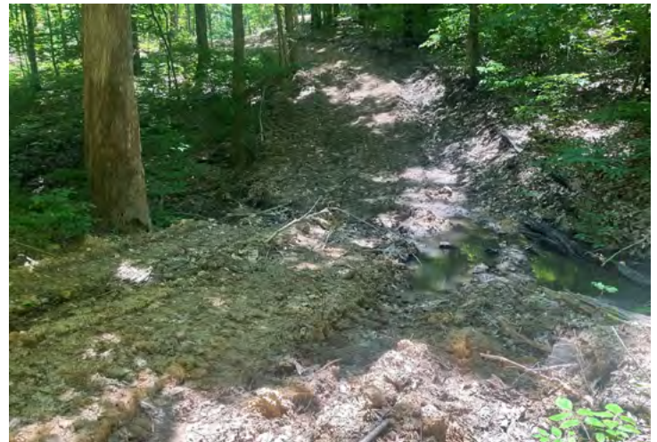
A skid trail was constructed with soil and pushed into this ephemeral channel blocking the flow, causing the water back up and to go over the trail, eroding the trail and causing sediment deposition in the channel. This will also lead to the eventual failure of this skid trail.
