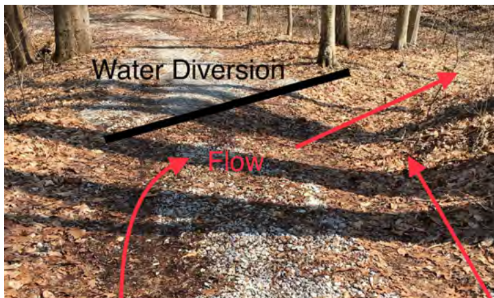
This gravel access has a well-armored and constructed waterbar to both allow movement of water off the road while still allowing the road to be functional.
