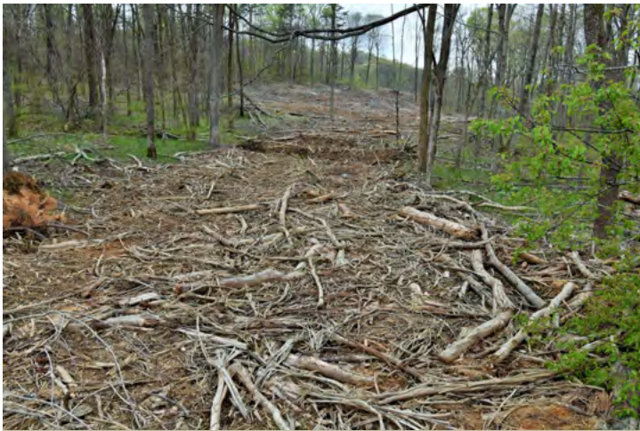
Debris used to armor a skid trail.
